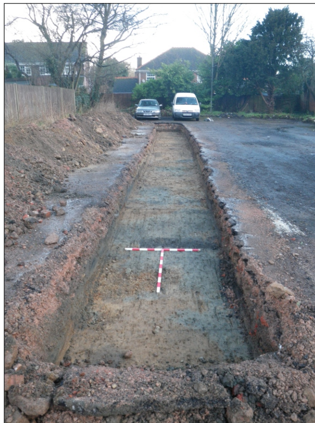
Plate 2: View of Trench 1 from the south
