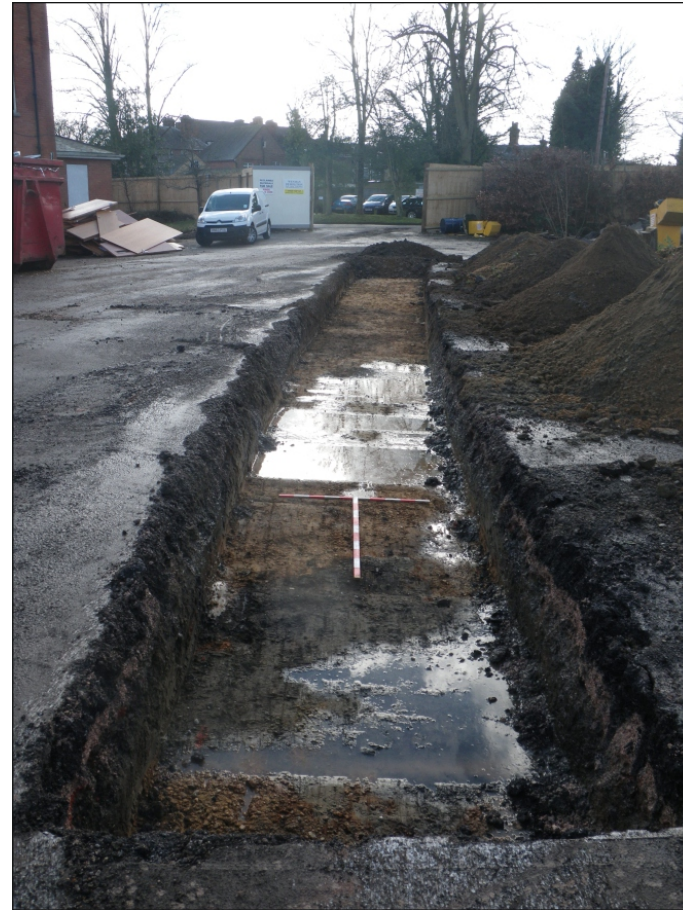
Plate 4: View of Trench 3 from the north
