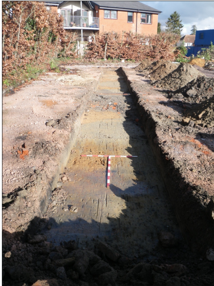
Plate 3: View of Trench 2 from the south
