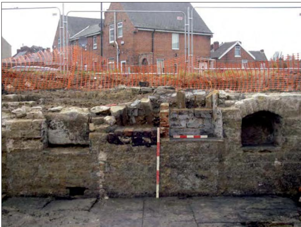
Plate 2: Northwest cellar wall - window and alcove blocking partially removed.
