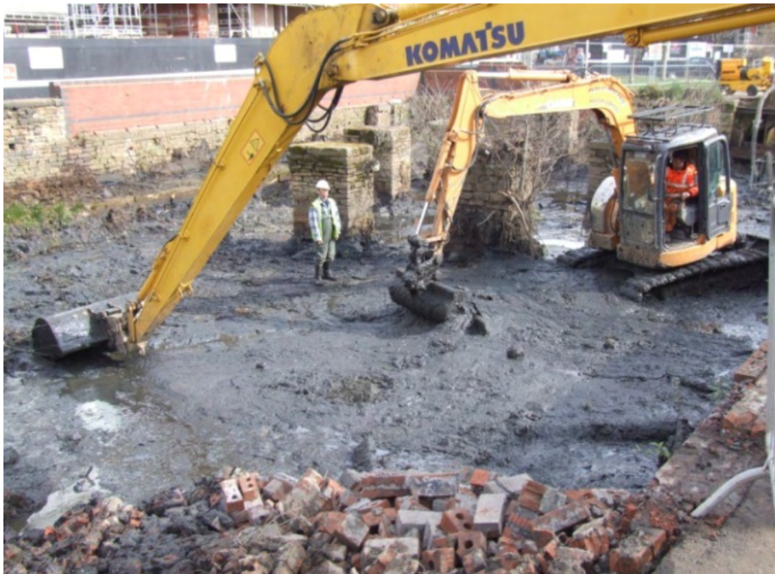
Plate 23: Watching Brief at Mill Sands goit; Dredging working shot
