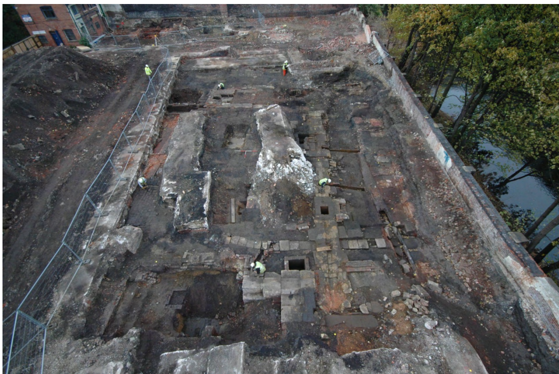
Plate 8: Trench 2/Mitigation Area B; Kelham Rolling Mill
