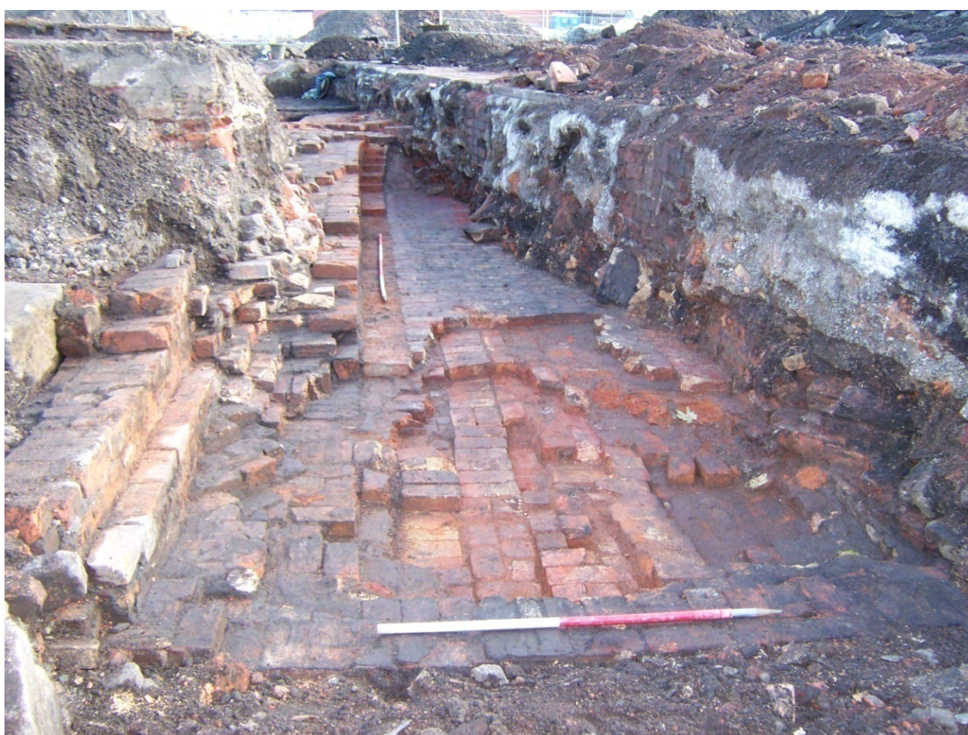
Plate 11: Trench 2/Mitigation Area B; Kelham Rolling Mill; boiler base
