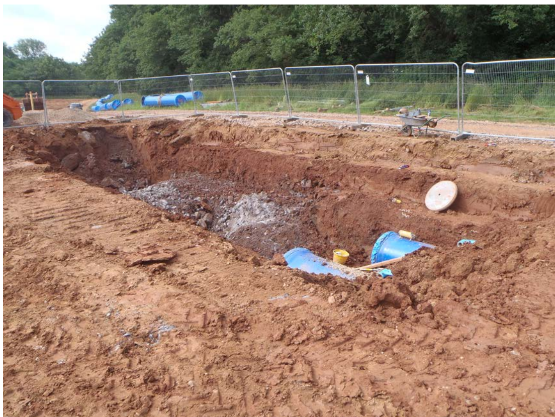
Plate 2: Typical stepped pipe trench section.
