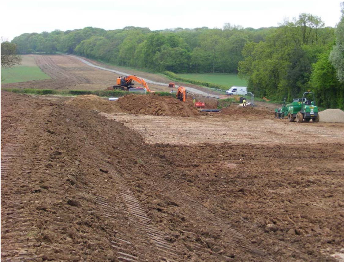
Plate 1: Shallow topsoil strip and bund.
