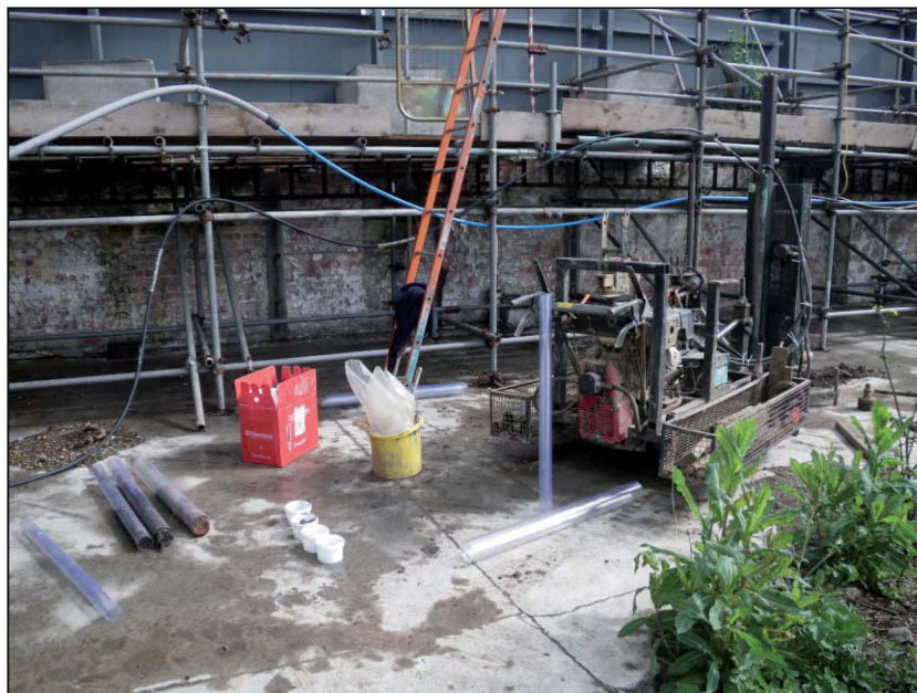
Plate 4: Excavation of Window Sample 1
