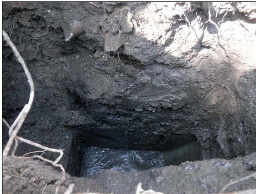
Plate 5: North facing section of Foundation Pit 1
