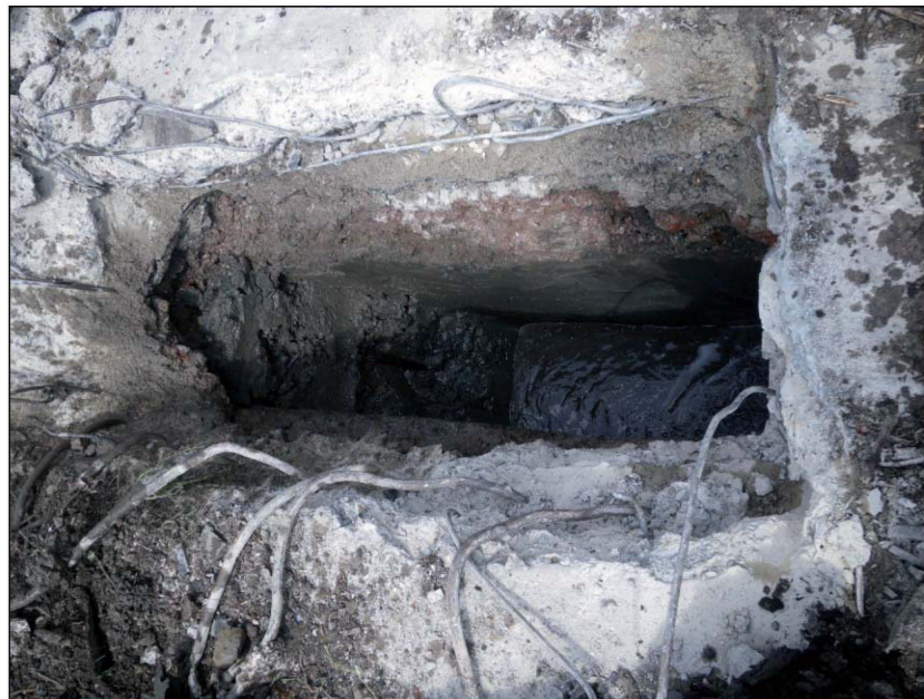
Plate 2: North Facing section of Test Pit 1
