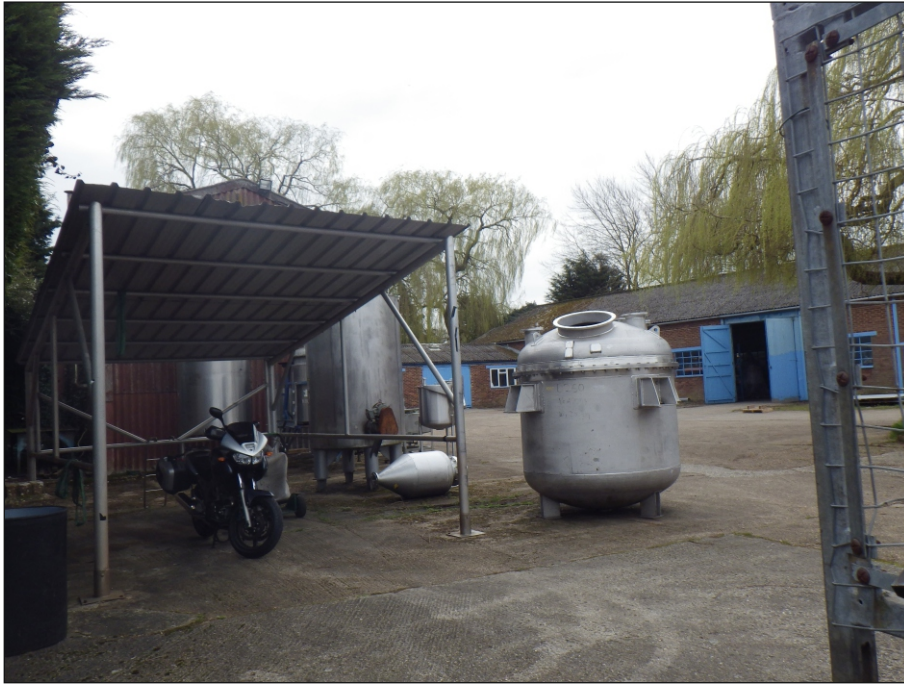
Plate 3: View facing south-east of structures and equipment associated with the works
