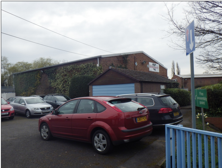
Plate 7: View facing south-east of central works buildings
