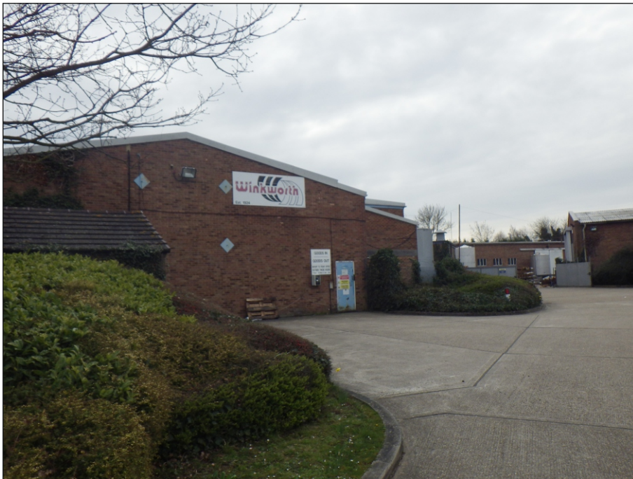
Plate 4: View facing east of the central buildings within the Site
