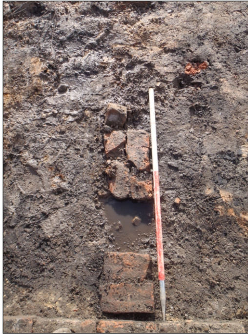
Plate 11: Ephemeral structure 2024 , possibly to support floor joists, from north
