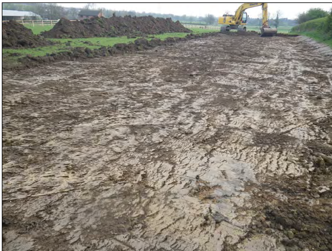
Plate 1: Topsoil strip along easement north of Desford Lane, facing north
