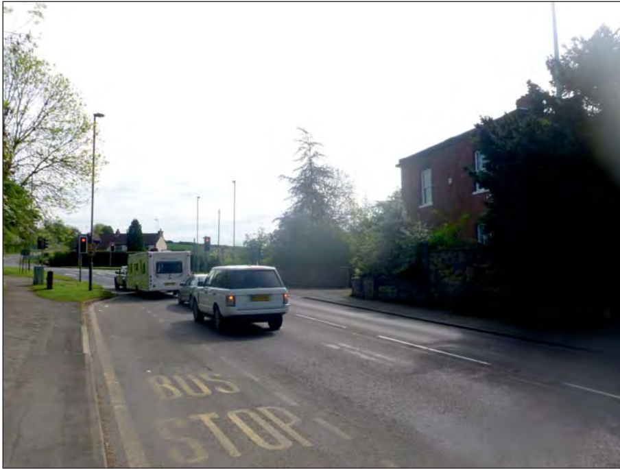
Plate 7: View of the Grade II Listed Norbriggs House towards the Site from the west
