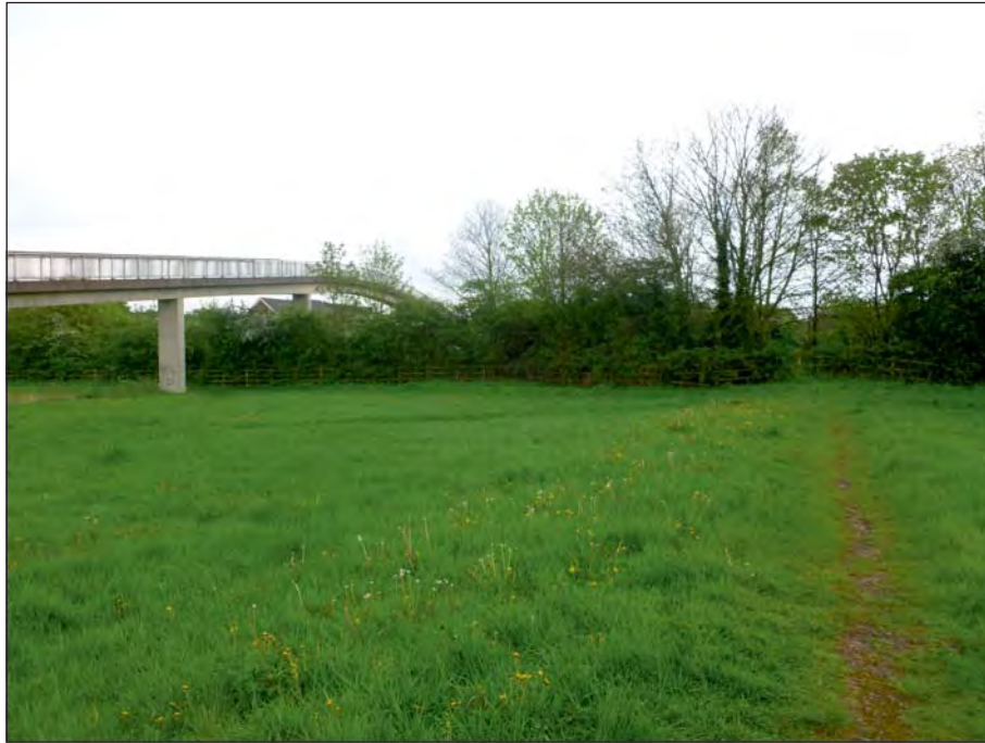
Plate 3: Extant pipeline and pedestrian bridge crossing the M40
