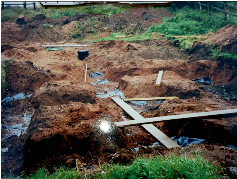
Plate 2: Site during construction of original sewage and drainage system, looking northwest
