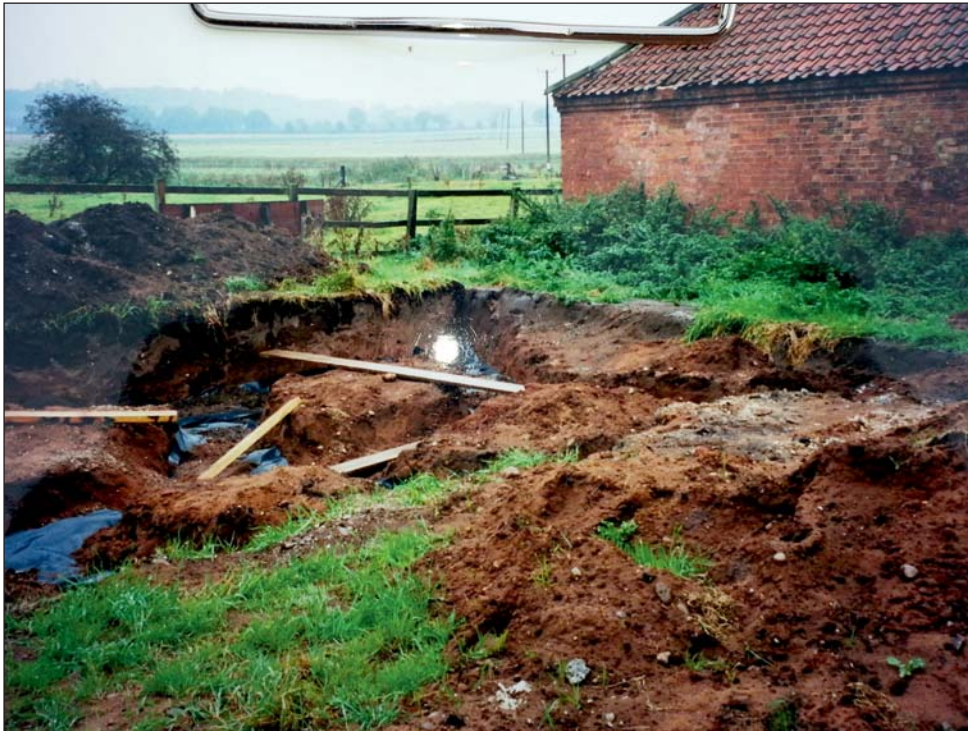
Plate 3: Site during construction of original sewage and drainage system, looking northeast
