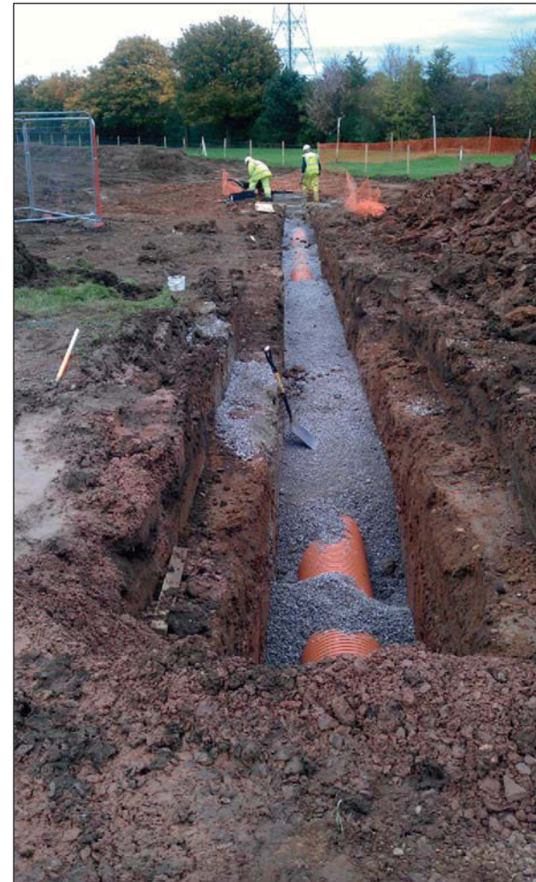
Plate 2: Excavation of pipe trench, facing north-east.
