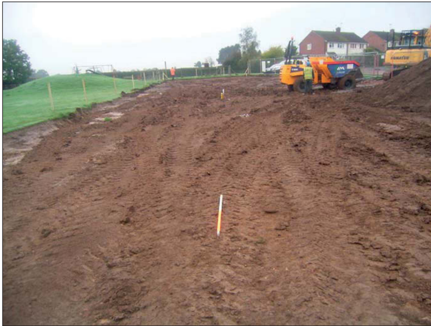
Plate 1: Topsoil strip to south of Peartree Close, facing south-west.
