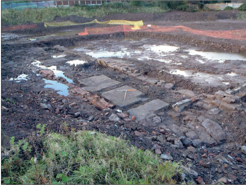
Plate 7: Area 2. General view looking south-west.
