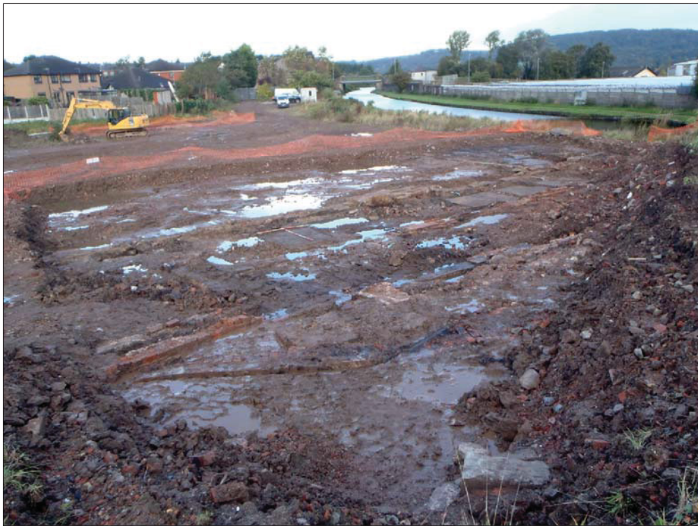
Plate 6: Area 2 General view looking north-west.
