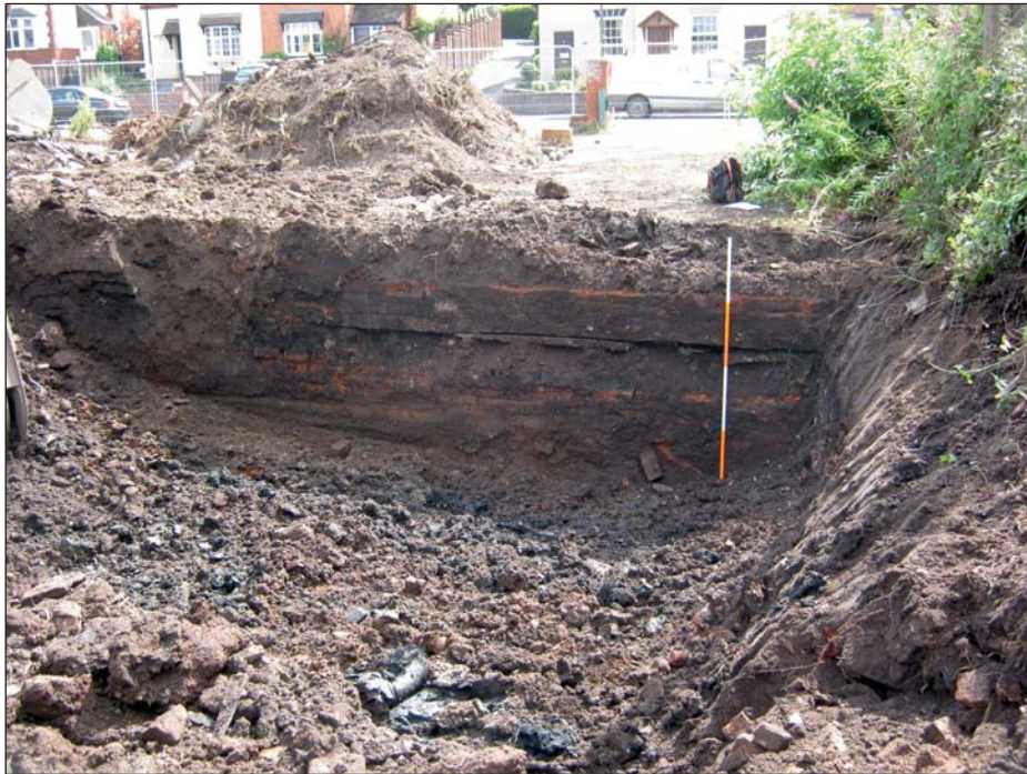
Plate 2: Canal wall, 1012 , looking south
