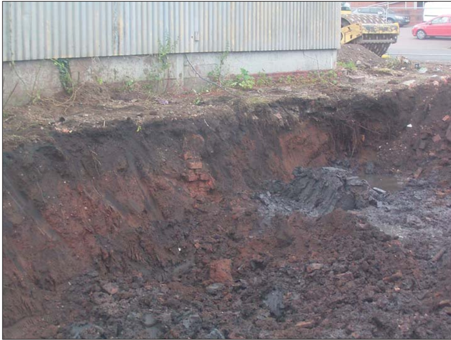
Plate 3: Canal wall, 1016 , looking south-east
