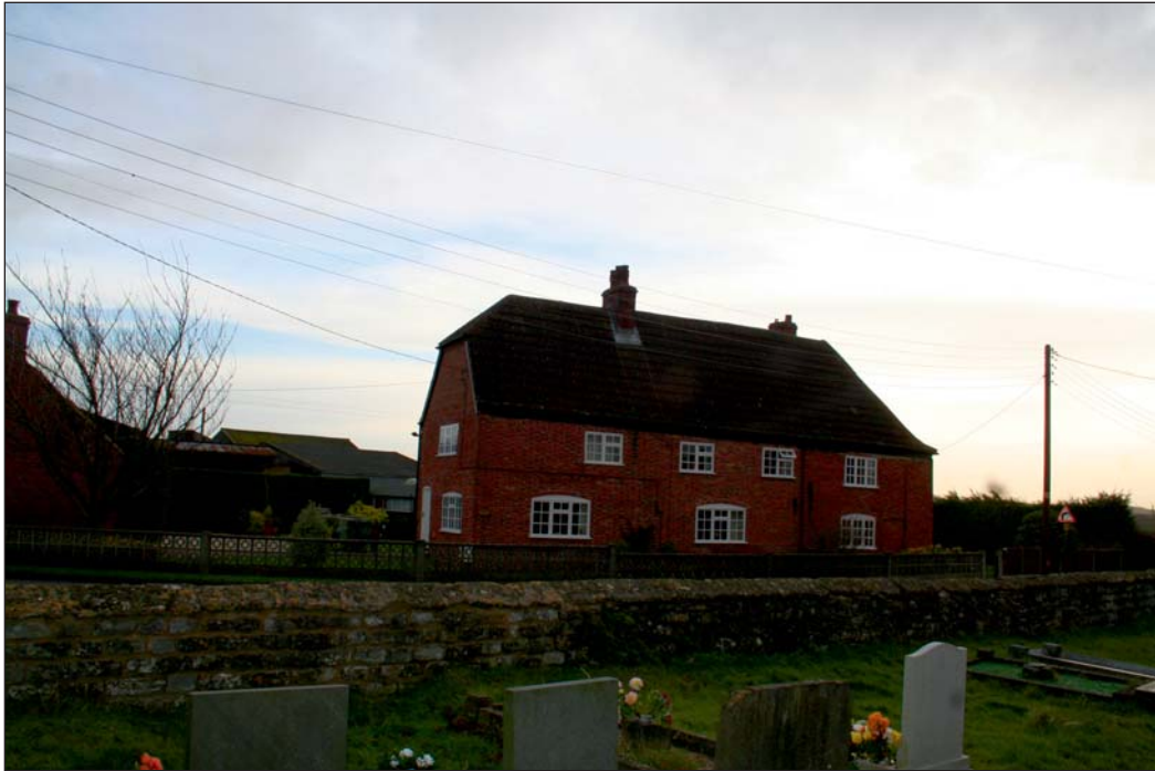
Plate 9: Grade II Listed Church View Cottages, view from northwest
