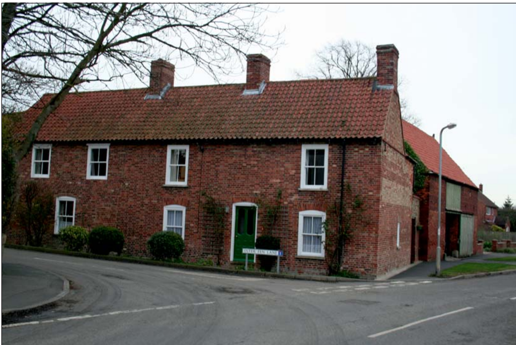
Plate 10: Grade II Listed Station Farmhouse, view from west
