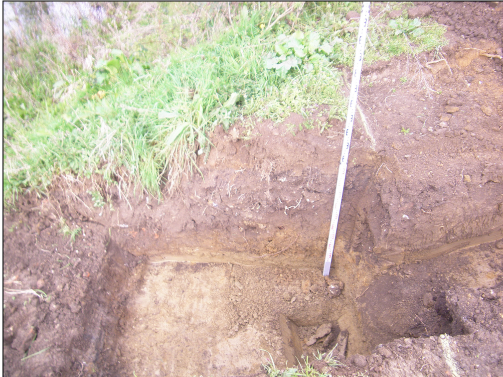
Plate 1: Pipe trench through canal bank, view from east
