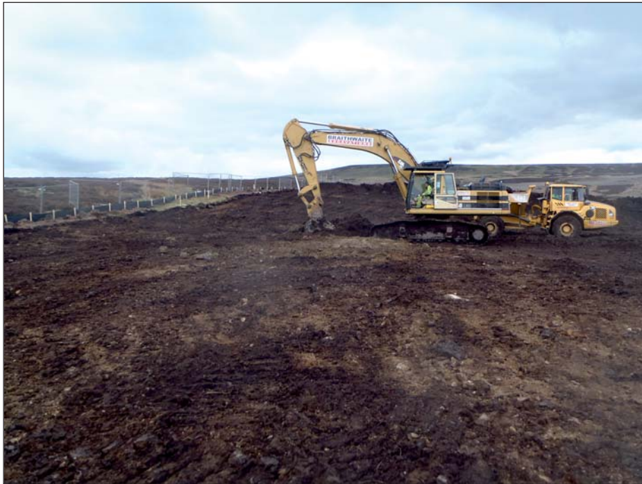
Plate 6: Stripping of topsoil.
