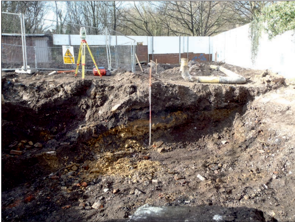
Plate 1: Southeast facing section of Trench 1, showing made ground deposits 100 , 104 , 105 , 106 and 107 .
