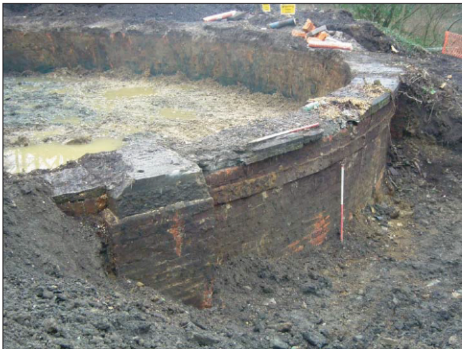
Plate 4: View of the external face of Gas Holder 1's cistern
