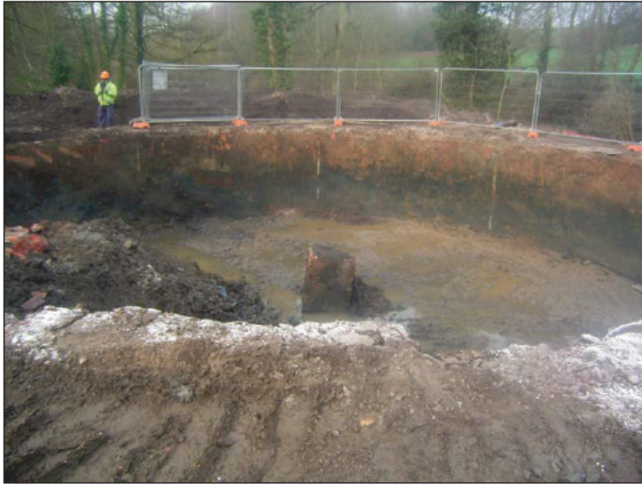
Plate 3: General view overlooking Gas Holder 1, noting iron guide rails 014 on internal face of cistern wall and central pier 015
