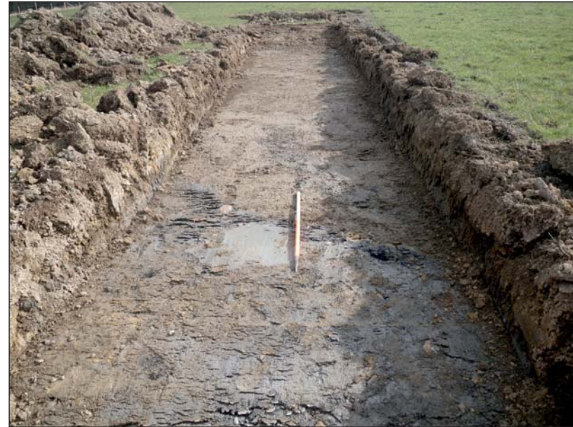
Plate 2: Trench 6, boundary of former opencast mine and coal seam
