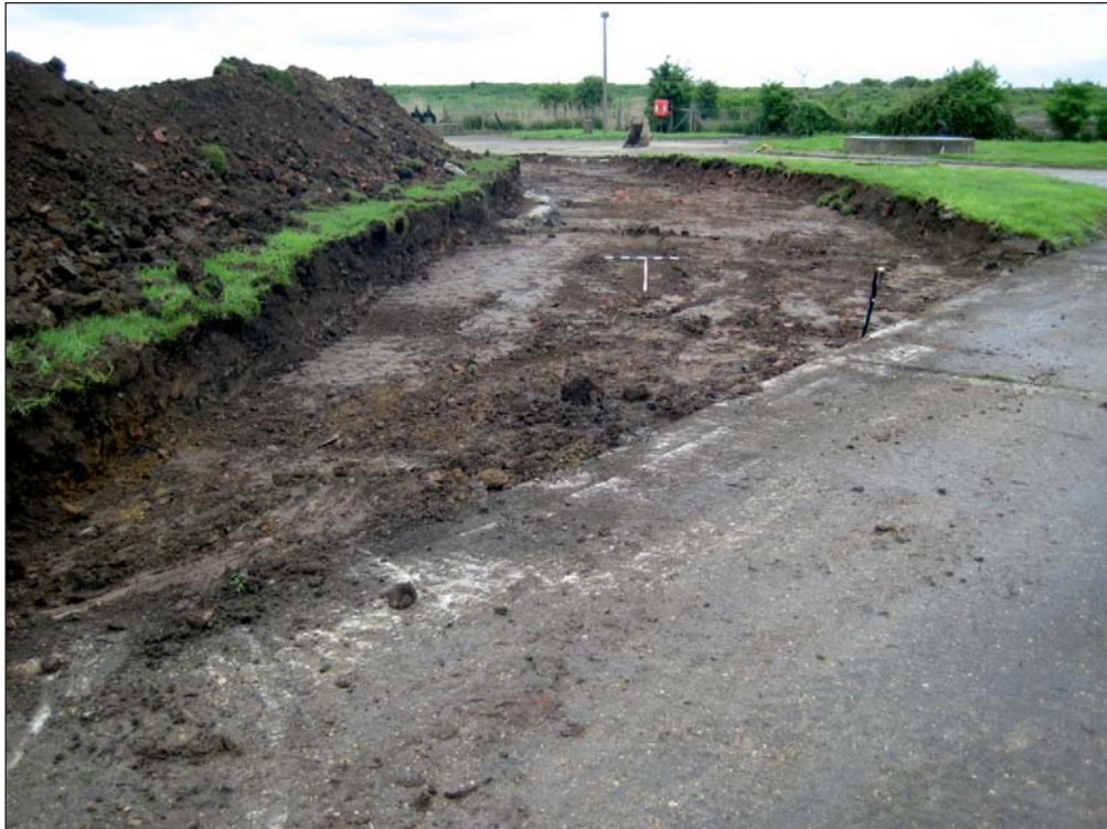
Plate 1: Trench 2, post excavation, from north-east.
