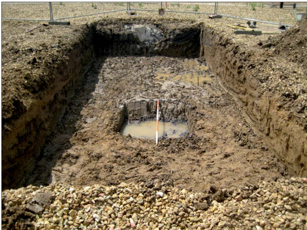
Plate 4: Trench 7, post excavation, from north-east.
