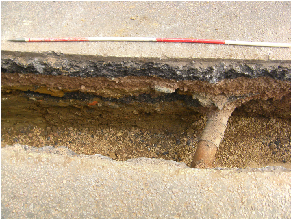
Plate 1: West facing section of pipe trench on High Street
