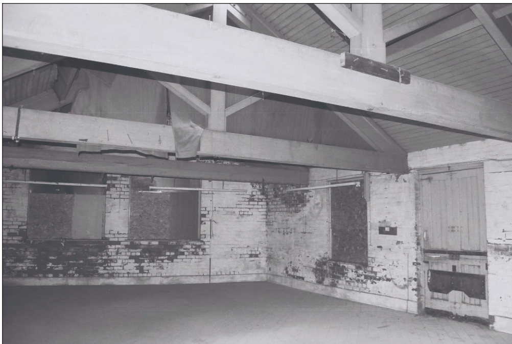
Plate 22: General view of room F6, looking northeast.
