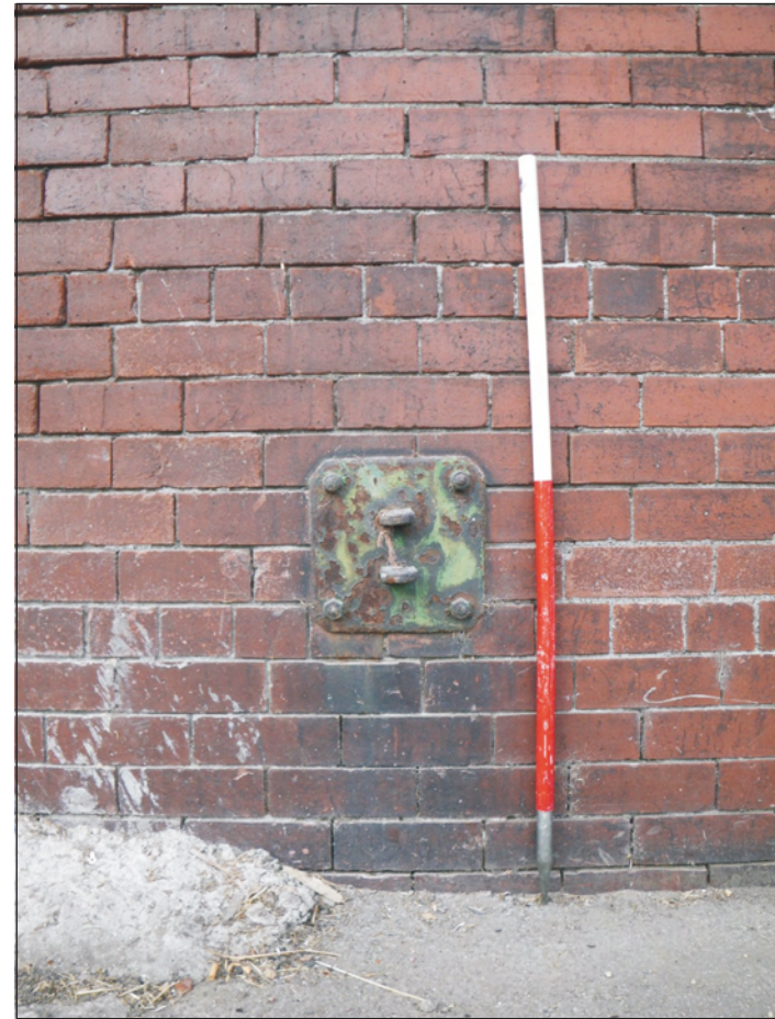
Plate 8: Detail of mounting, possibly for a gib crane.
