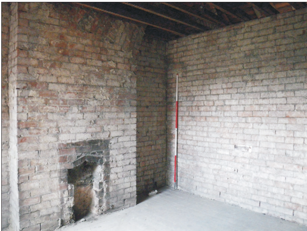
Plate 20: General view of room F3, looking northeast.
