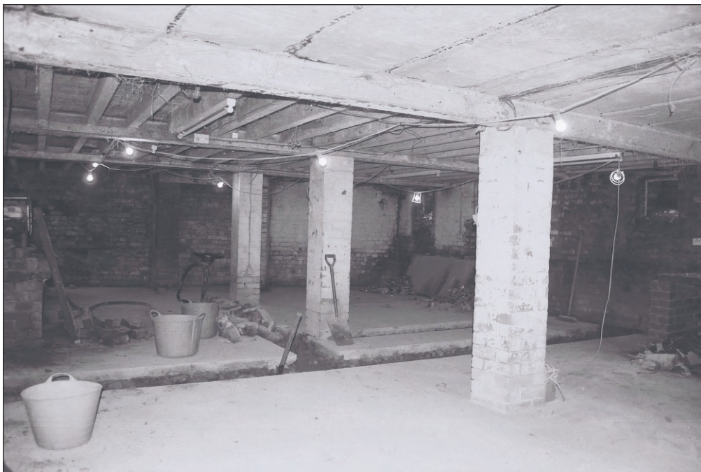
Plate 12: General view of room C2, looking northeast.
