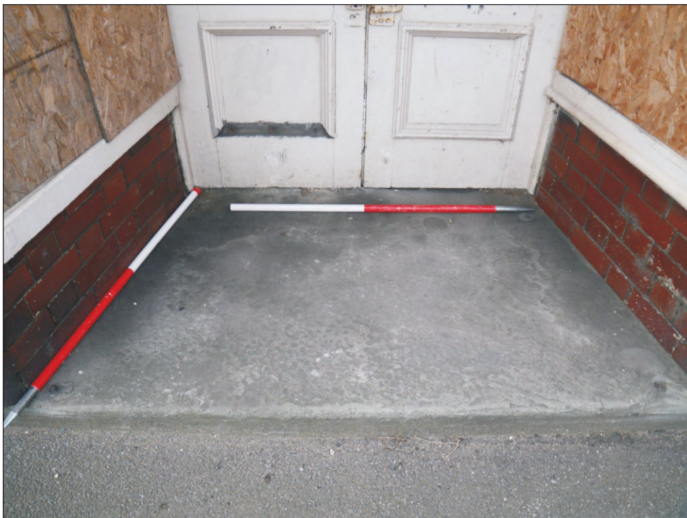
Plate 4: Detail of shop entrance threshold showing scars and glazed bricks.
