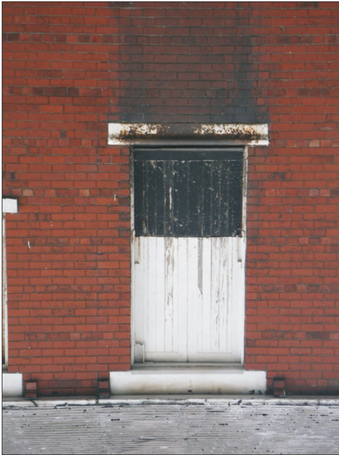
Plate 7: Detail of taking in door, noting iron threshold.
