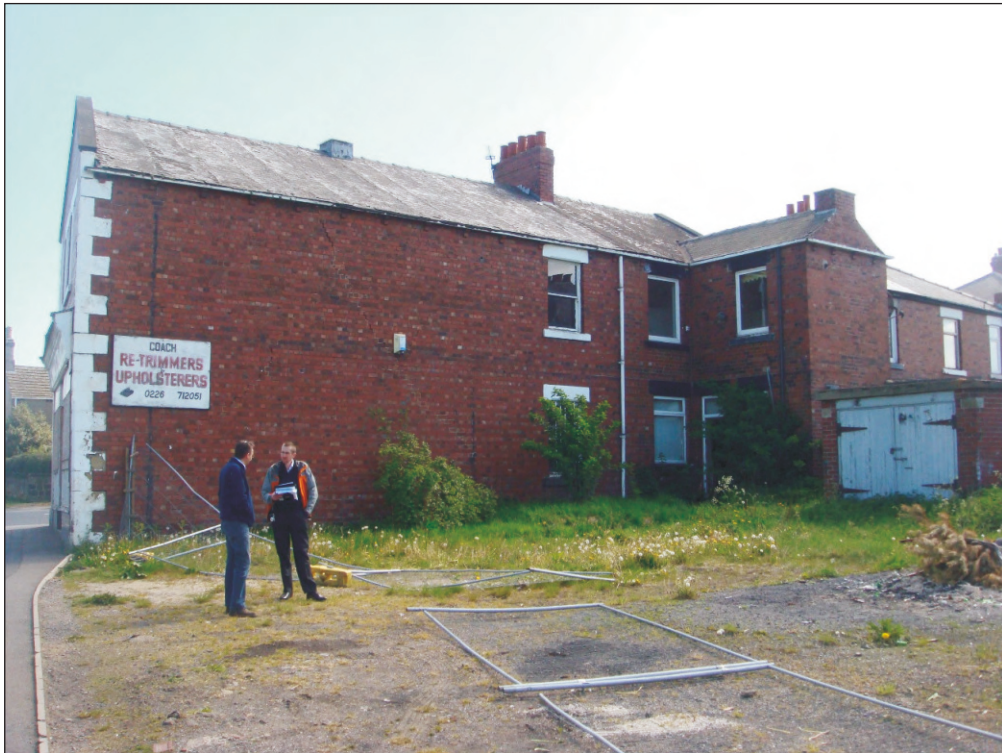
Plate 9: General view of west elevation.
