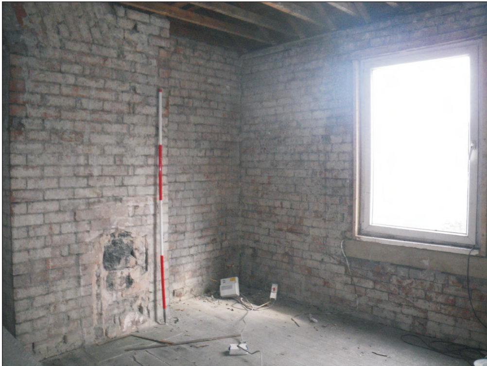
Plate 21: General view of room F5, looking northeast.
