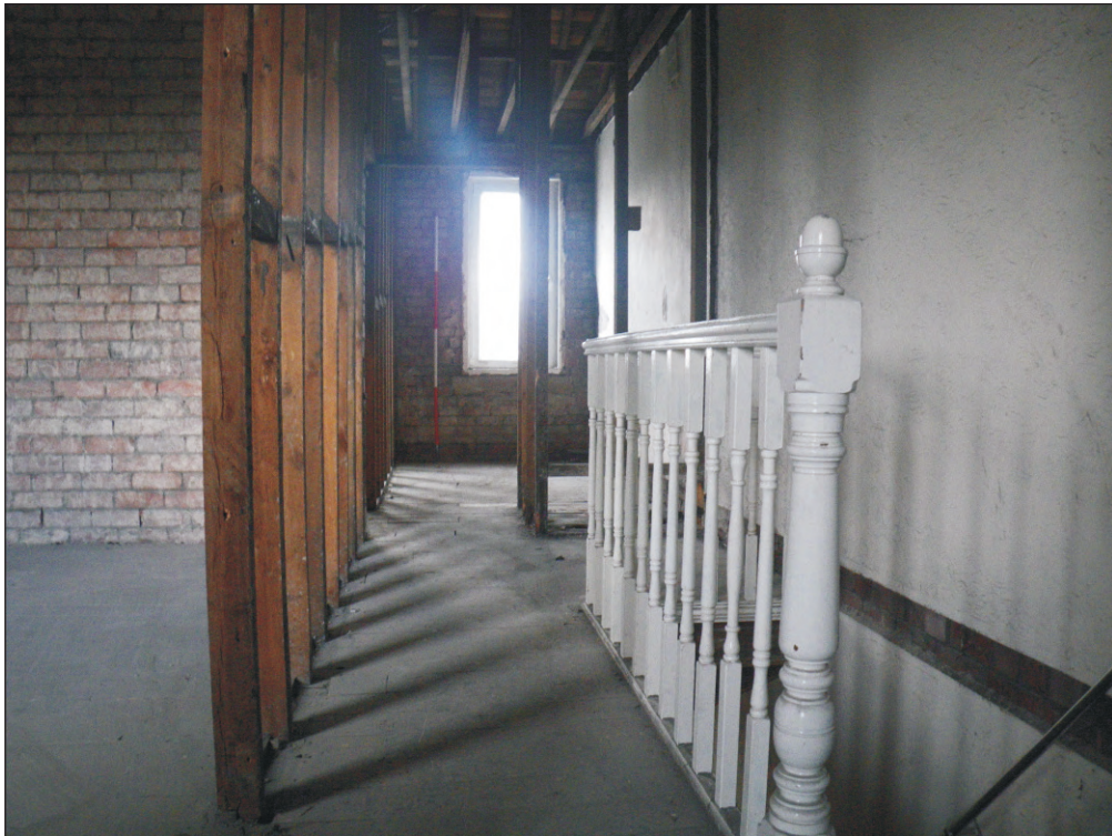
Plate 19: General view along hall F2 into room F4, looking east.
