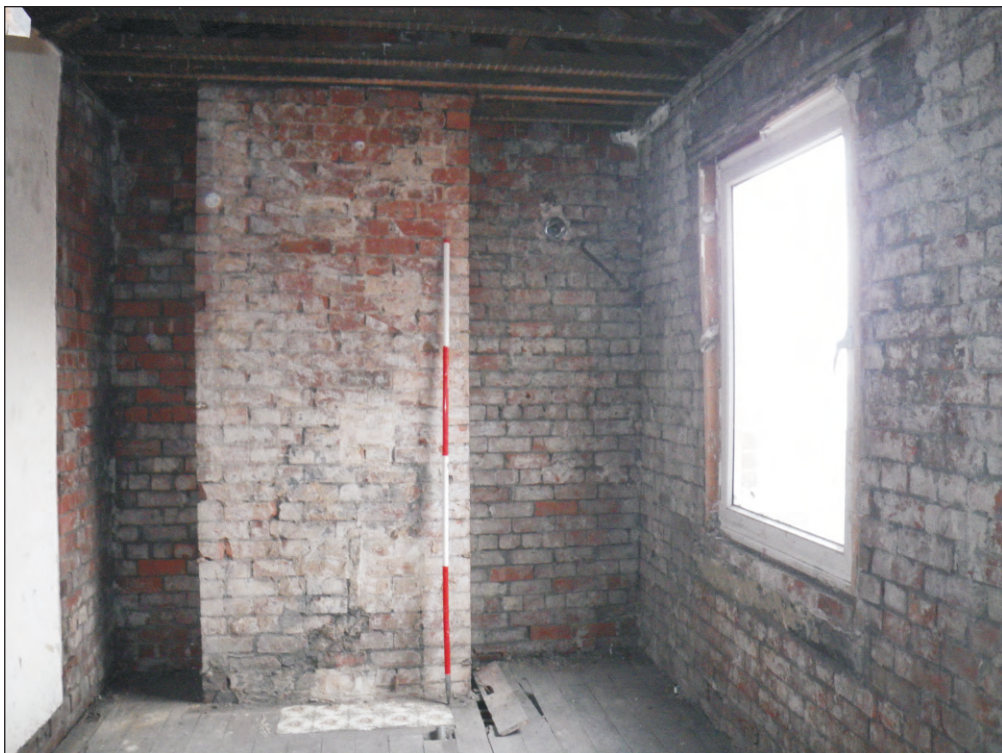
Plate 18: General view of room F1, looking west.
