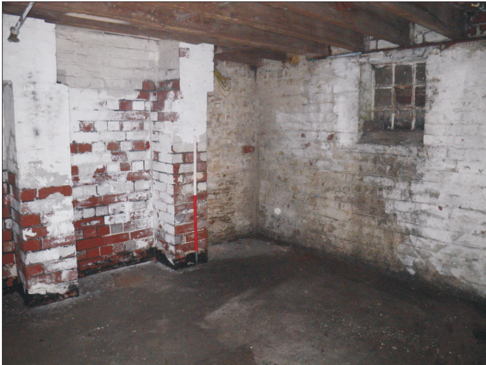
Plate 11: General view of room C1, looking northeast.
