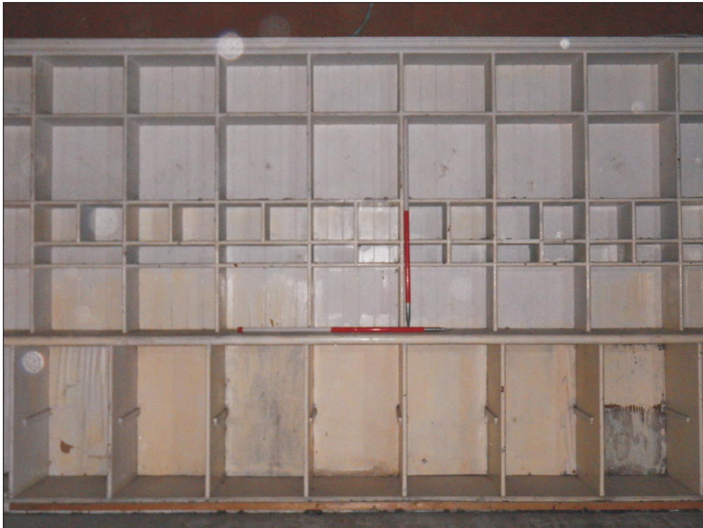
Plate 17: Detail of shelving in room G8, looking west.
