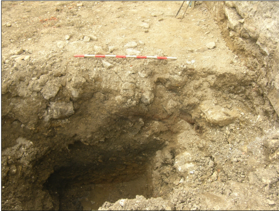
Plate 1: Footing adjacent to south-east corner of existing building, view from north-east
