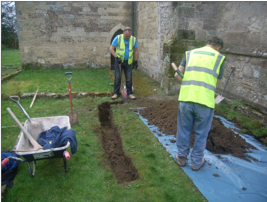
Plate 8: Hand excavation of cable trench in the churchyard
