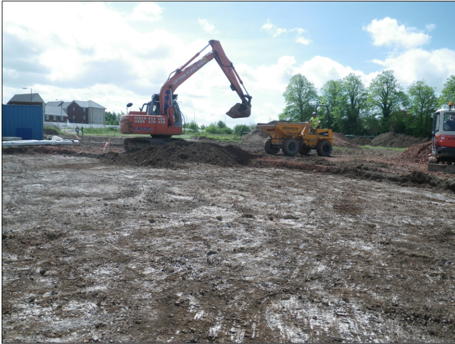
Plate 1: Stripping of site
