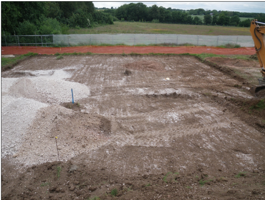
Plate 2: Stripping of site
