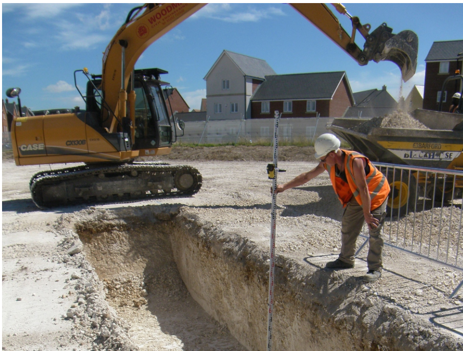
Plate 4: Machining through made up ground
