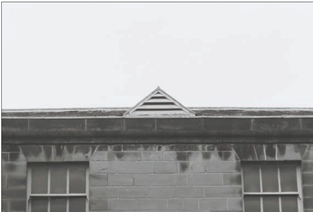
Plate 27: Detail of pitched timber louvered roof vents of the east end of the North Range (Film 20.34)
