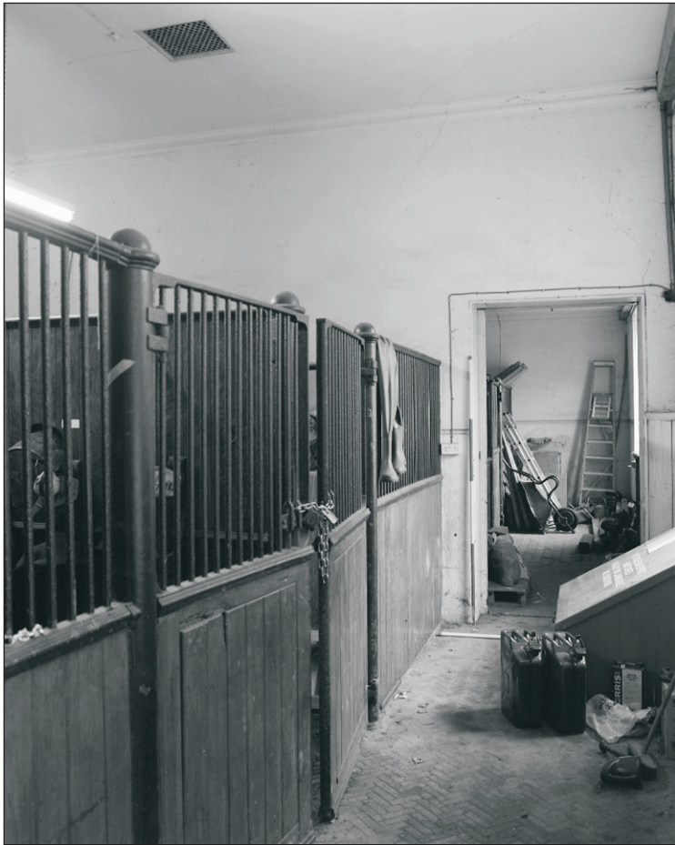
Plate 585: General view of G56, East Range (Film 19.01)
