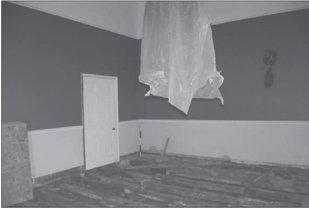
Plate 477: General view of G47, South Range - Agent's House (Film 75.14)
