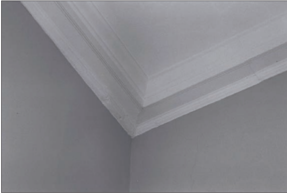
Plate 293: Detail of cornice, G22, West Range (Film 23.18)
