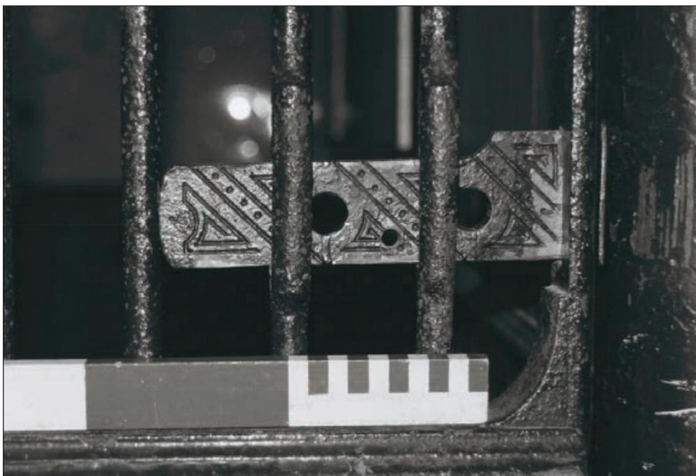
Plate 57: Detail of original decorative loose box door latch, room G2, East Side of the North Range (Film 14.27)
