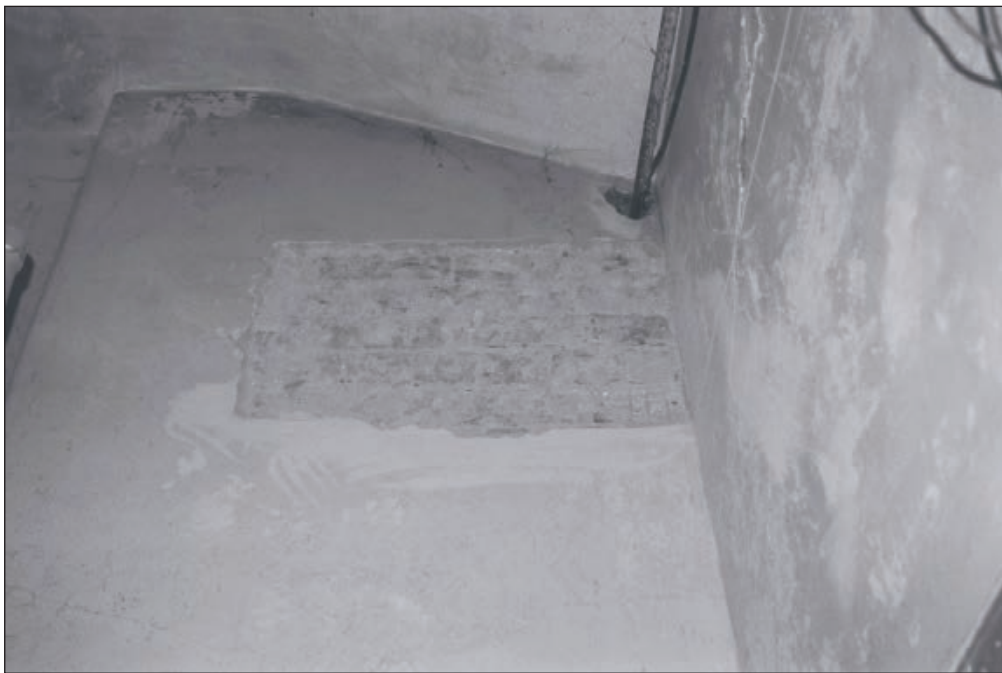
Plate 207: View of area of removed plaster exposing brick fabric, west wall of F12, Central Entranceway of the North Range - OB. 27 (Film 48.17)
