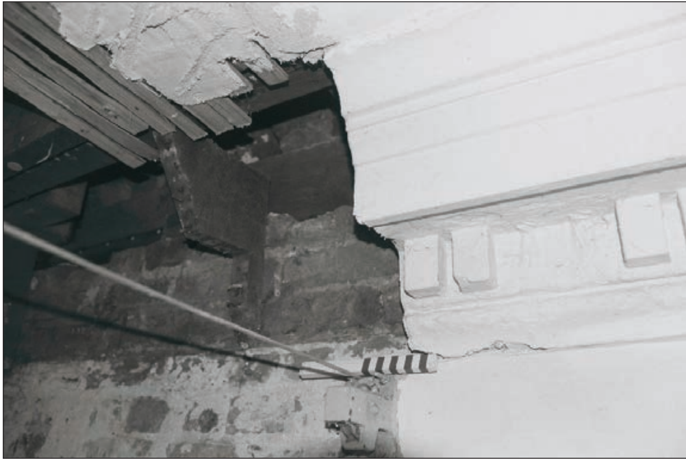
Plate 409: Detail of cornice structure, G30, South Range - OB. 104 (Film 72.14)
