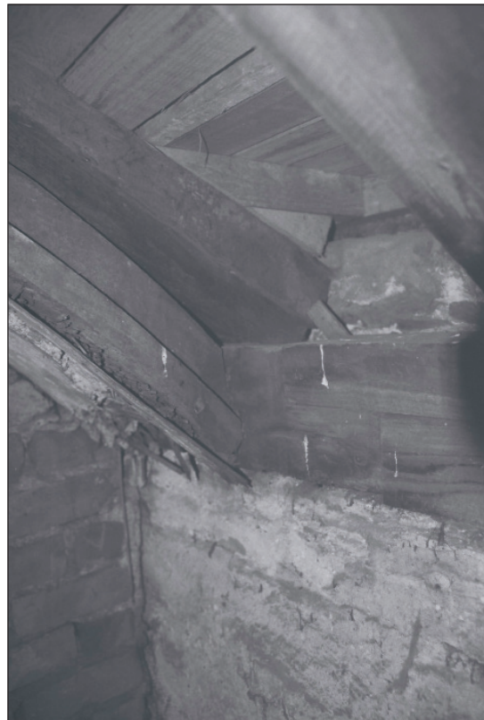
Plate 455: Detail of original ceiling construction, G42, South Range - OB. 97 (Film 74.30)
