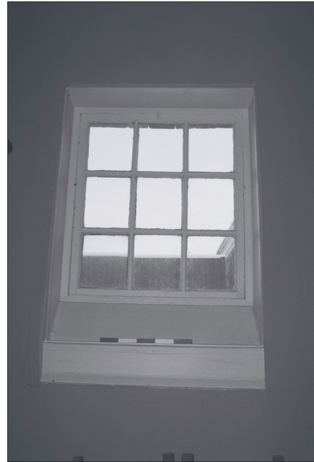
Plate 310: Detail of high window, east wall of G24, West Range (Film 22.09)
