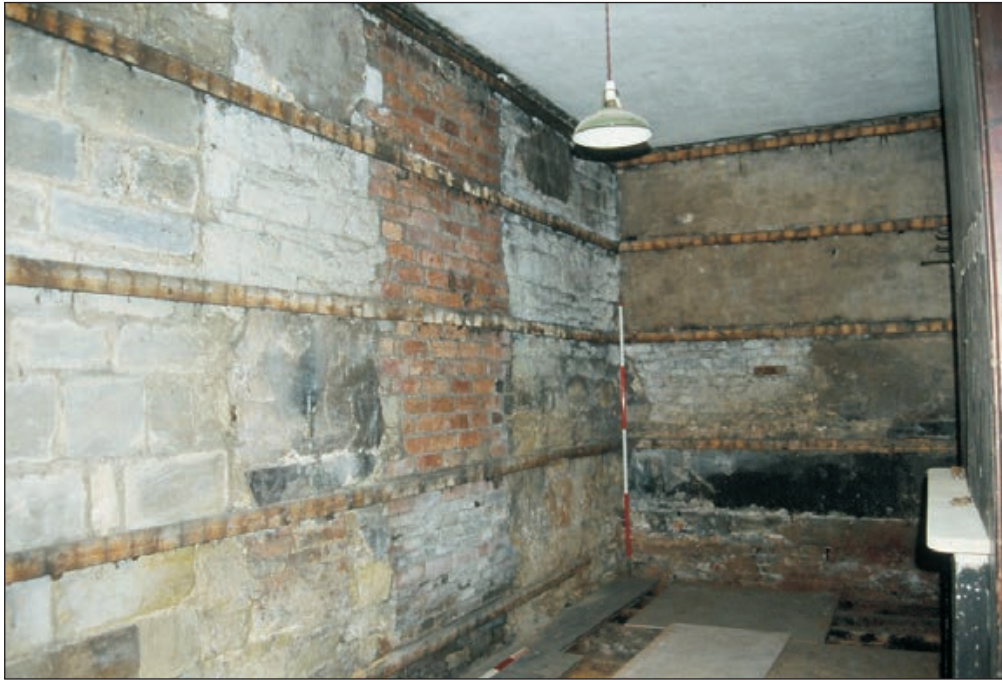
Plate 84: View of room G4, 'Tack Room', Central Entranceway of the North Range, after removal of match boarding, showing blocked openings - OB. 71 & 73 (Film C.S. 39)
