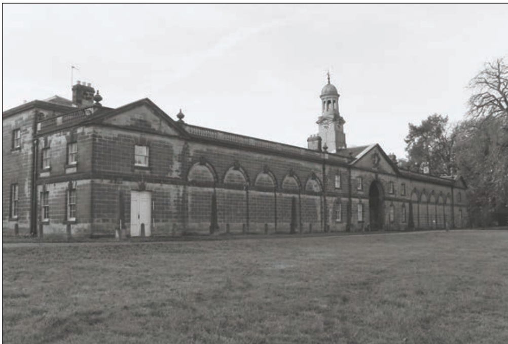
Plate 4: General view of the north elevation of the North Range from the northeast (Film 11.25)
