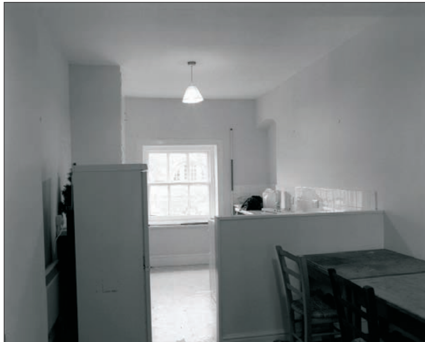
Plate 158: General view of room F9, Central Entranceway of the North Range (Film 04.08)
