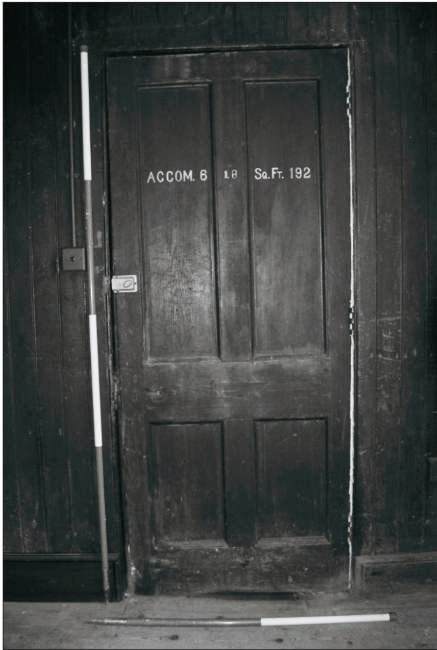
Plate 74: Detail of timber panelled door, room G4, 'Tack Room', Central Entranceway of the North Range (Film 15.25)
