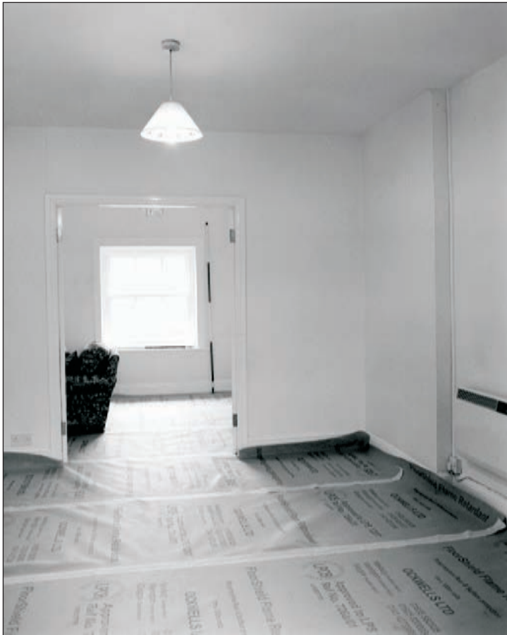
Plate 154: General view of room F6 with F7 beyond, East Side of the North Range (Film 05.01)
