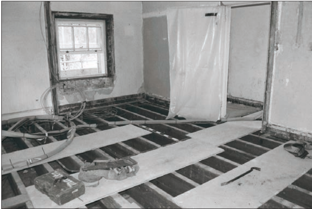
Plate 260: General view of exposed timber and RSJ floor structure, room F22, West Side of the North Range - OB. 58 (Film 72.34)
