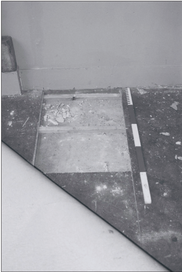
Plate 411: Detail of exposed concrete floor of G30, South Range - OB. 15 (Film 46.16)
