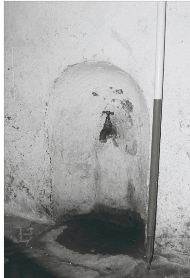
Plate 576: Detail of recessed drain, west wall of G55, East Range (Film 16.23)
