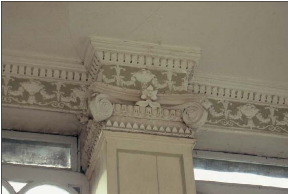
Plate 462: Detail of original cornice and column head, G41, South Range (Film C.S. 6.)
