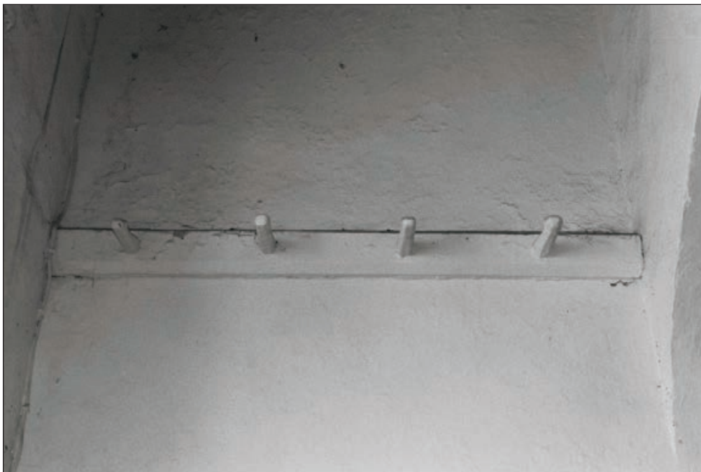
Plate 106: Detail of timber hooks, west wall of room G11, Central Entranceway of the North Range (Film 52.11)
