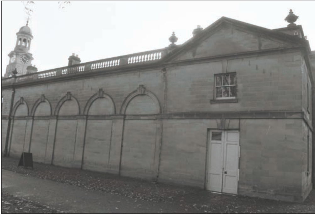
Plate 29: General view of the west end of the north elevation of the North Range (Film 11.18)
