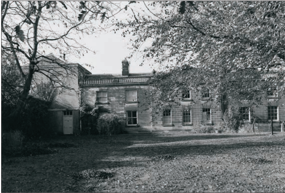
Plate 565: View of the south end of the east elevation of the South and East Ranges (Film 01.09)
