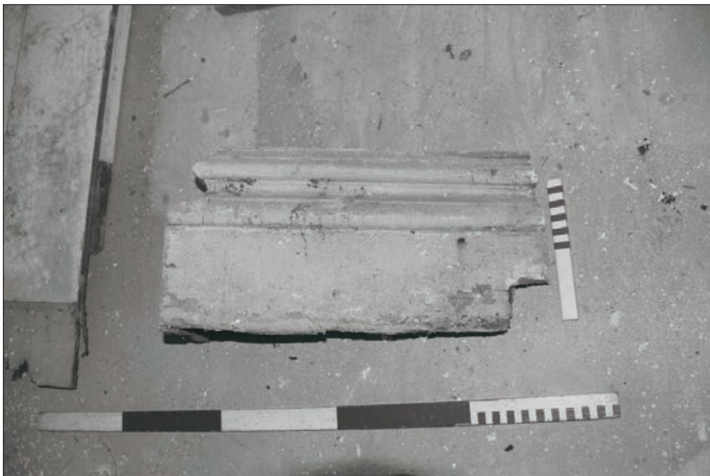
Plate 471: Detail of removed moulded skirting from base of columns, G41, South Range - OB. 106 (Film 73.21)
