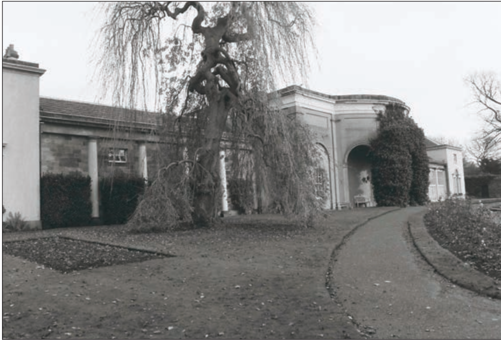
Plate 337: General view of the south elevation of the South Range (Film 13.34)
