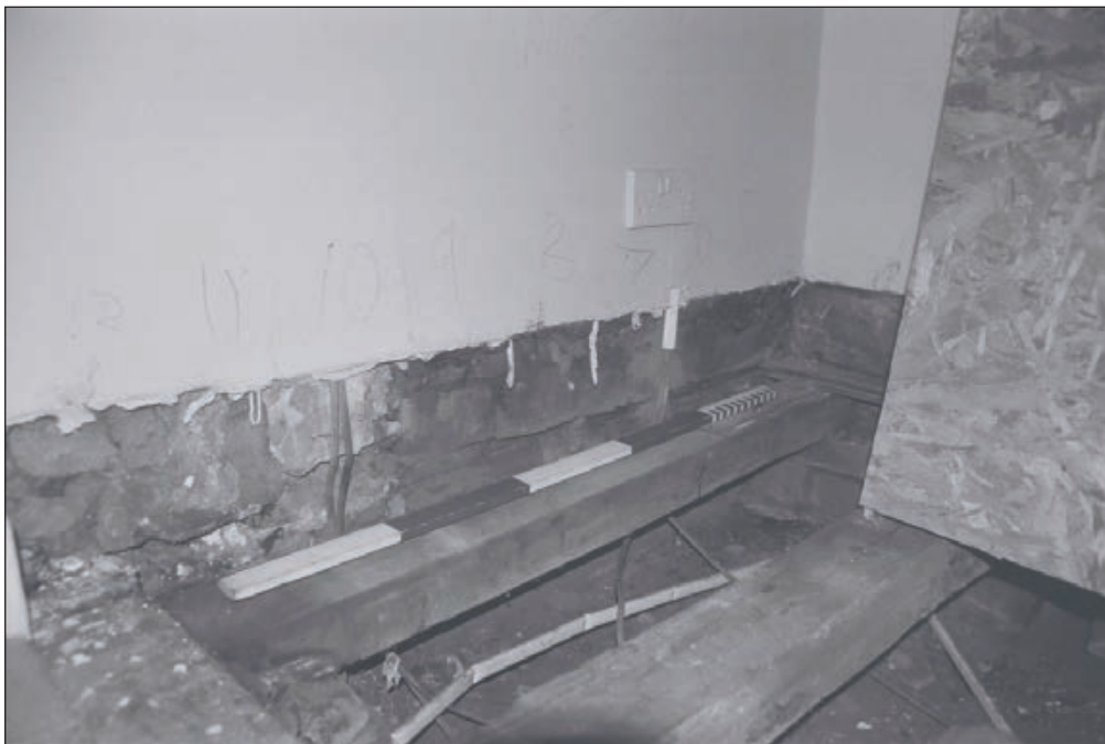
Plate 484: Detail of probable blocking within the west wall of G47, South Range - Agent's House - OB. 118 (Film 75.07)
