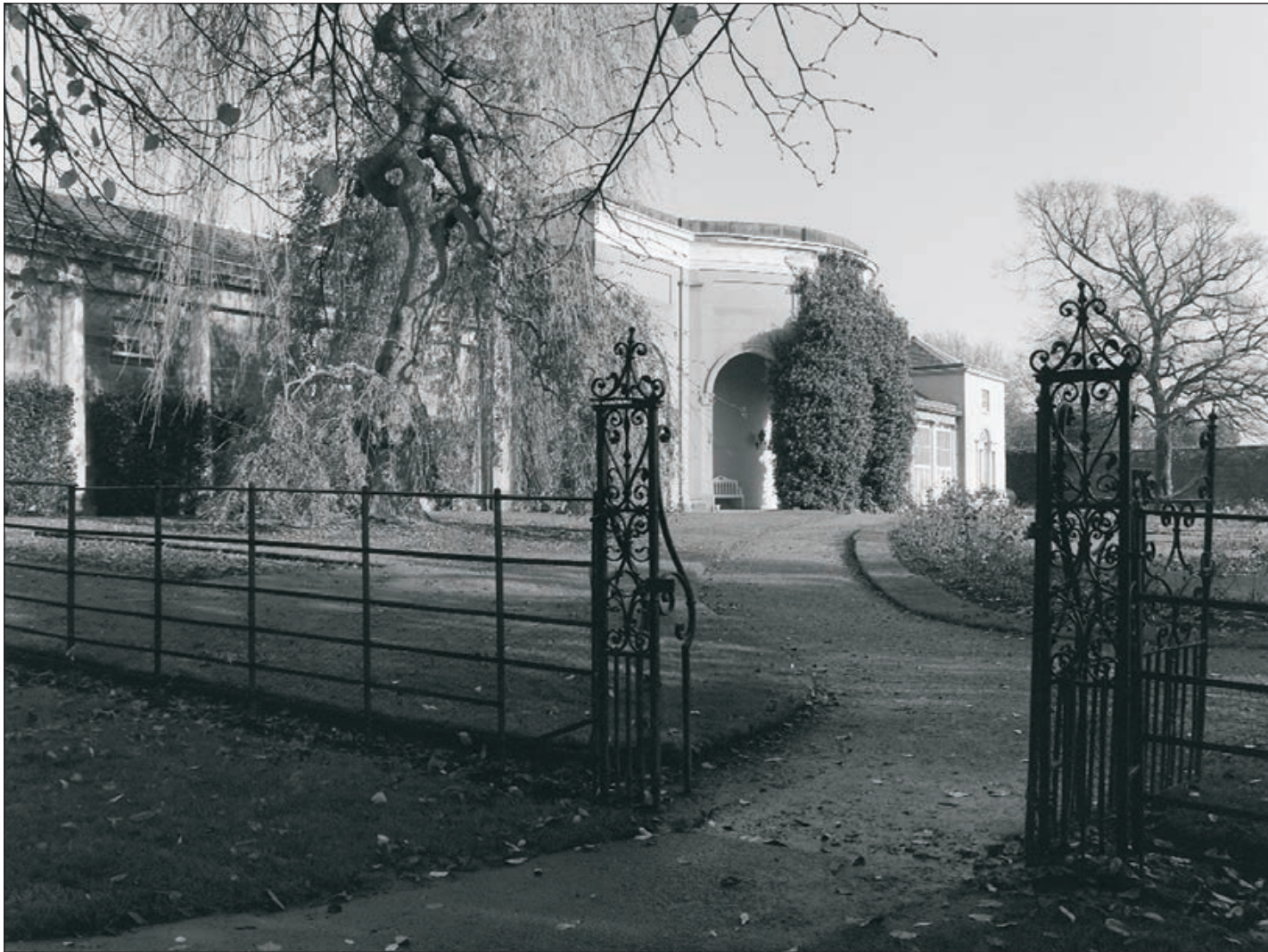
Plate 7: General view of the south elevation of the South Range, from the southwest (Film 02.01)
