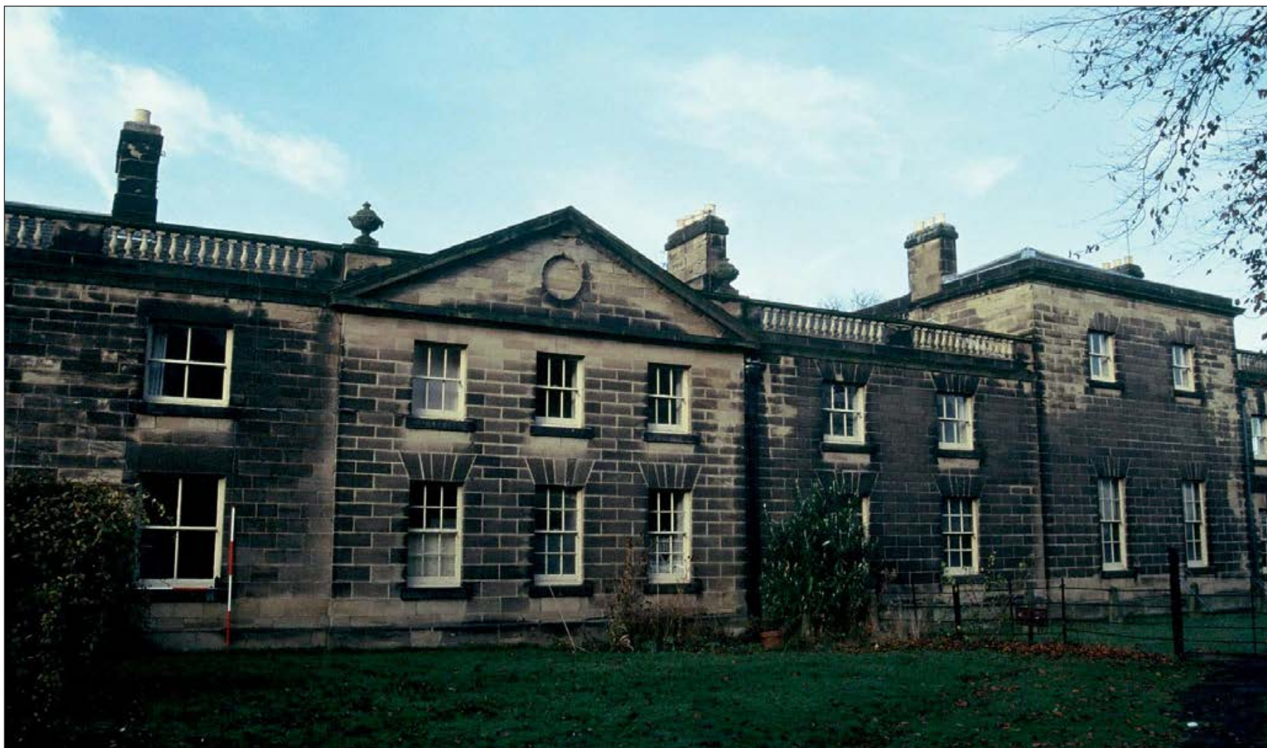
Plate 564: General view of the east elevation of the South and East Ranges, looking northwest (Film C.S.2.)
