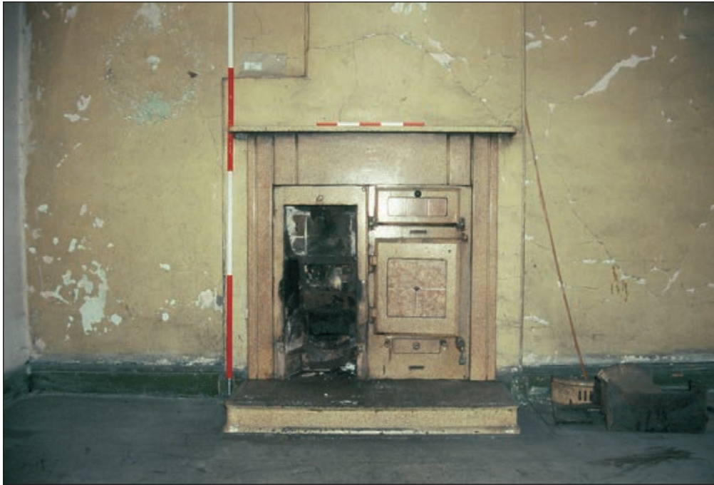
Plate 226: View of range, east wall of room F15, West Side of the North Range (Film C.S. 28)
