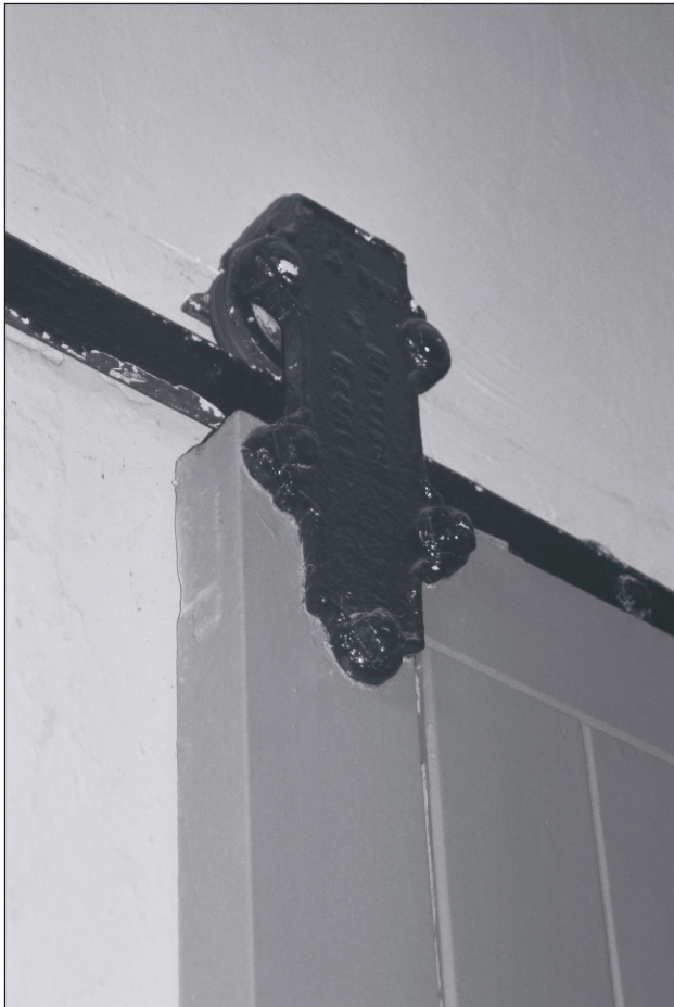
Plate 299: Detail of iron bracket and roller on rolling door, G23, West Range (Film 23.33)
