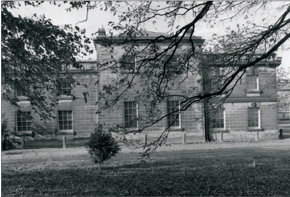
Plate 562: View of the north end of the east elevation of the North and East Ranges (Film 01.08)
