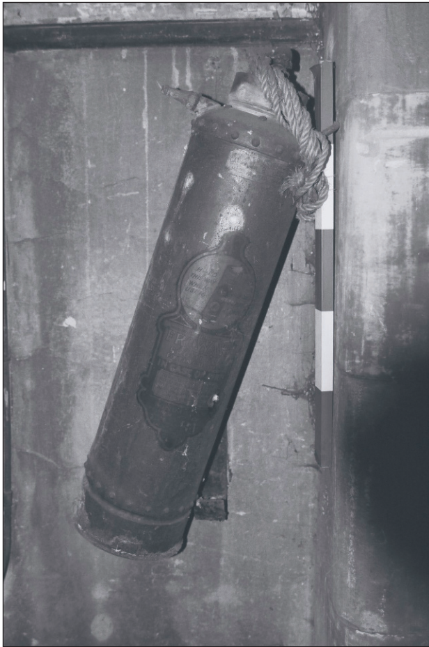
Plate 120: Detail of 1944 fire extinguisher, room G15, West Side of the North Range (Film 26.15)
