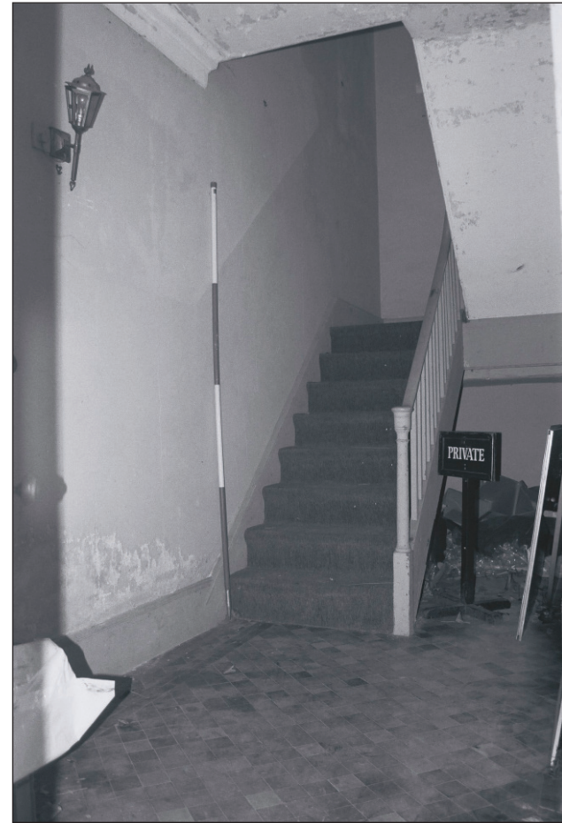
Plate 425: General view of G35, South Range (Film 41.13)
