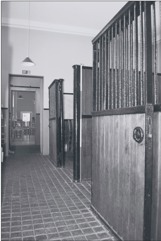
Plate 289: General view of loose boxes in G22, West Range (Film 23.14)
