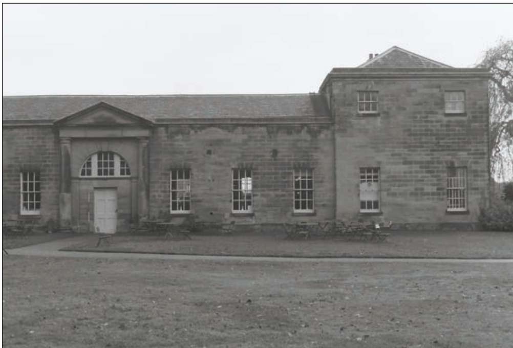
Plate 264: General view of the south end of the west elevation of the West and South Ranges (Film 12.19)
