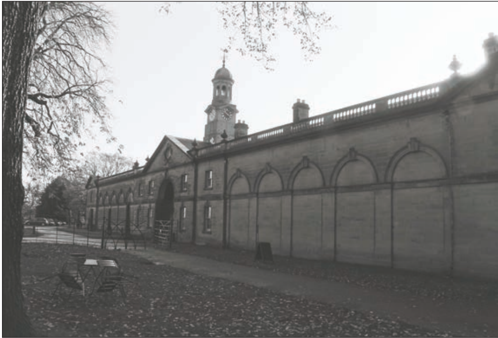
Plate 5: General view of the north elevation of the North Range from the northwest (Film 11.20)
