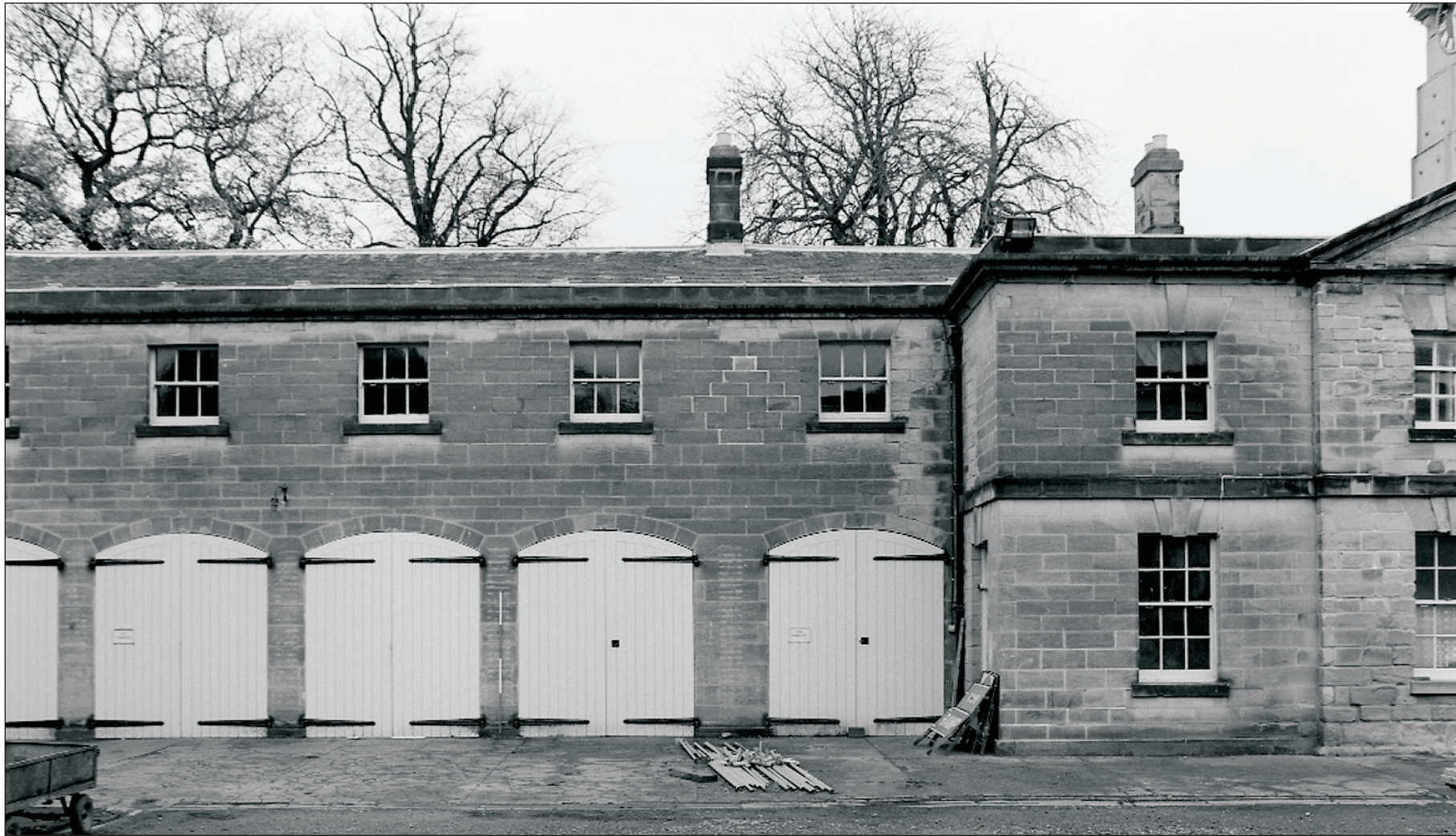
Plate 33: View of the phase 7 west end of the south (courtyard) elevation of the North Range (Film 17.03)
