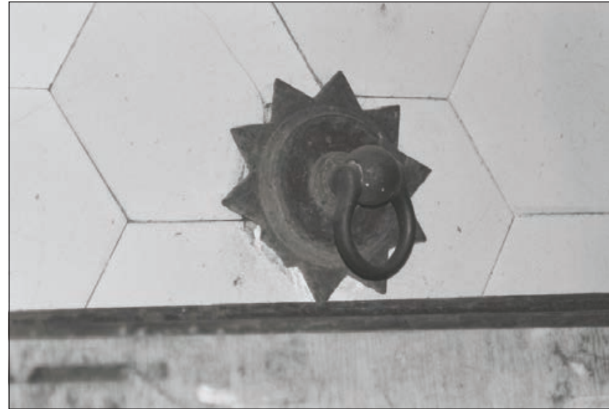
Plate 580: Detail of iron tether hook, G55, East Range (Film 16.29)
