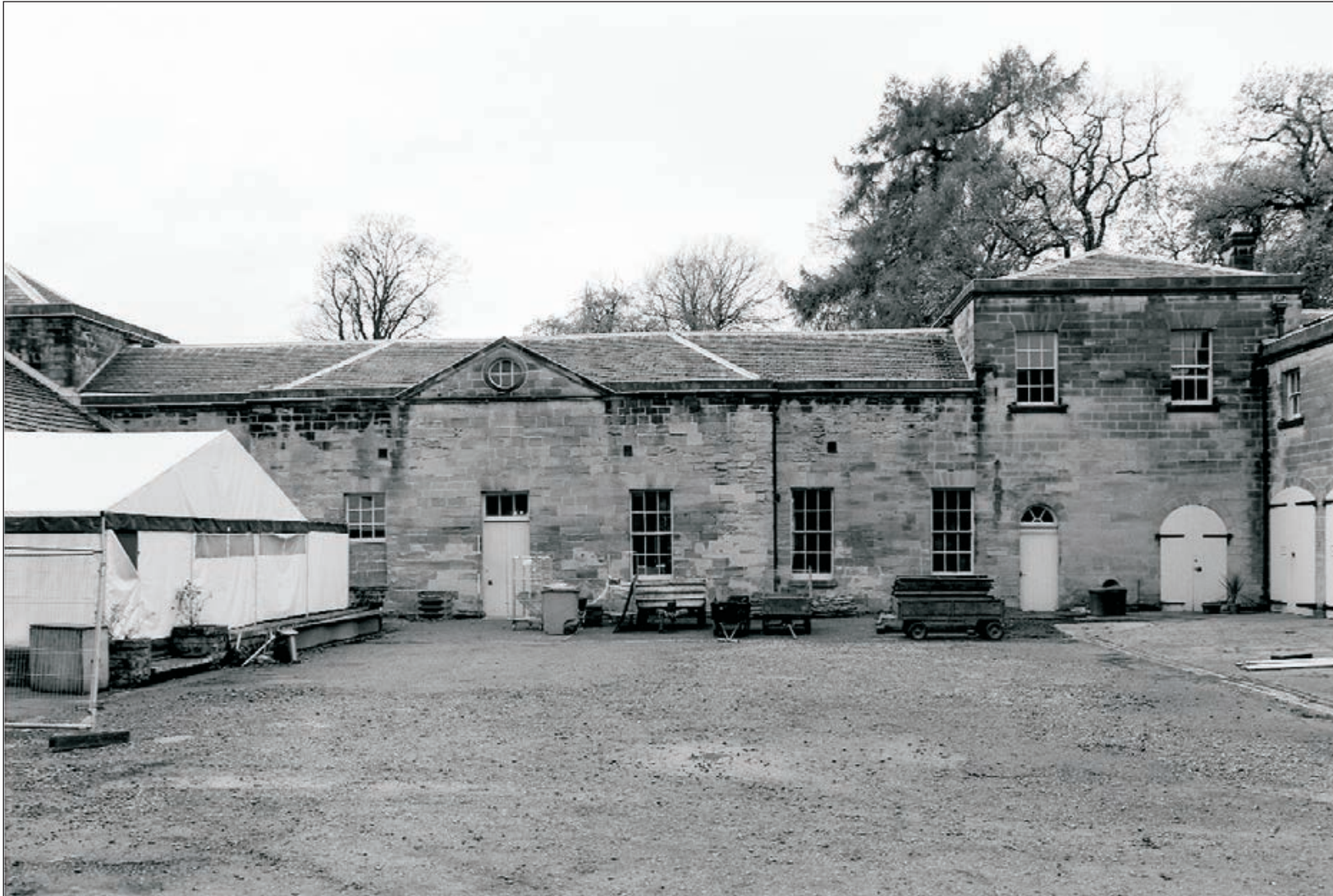
Plate 269: View of the east facing courtyard elevation of the West Range (Film 18.03)
