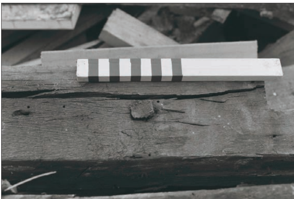
Plate 221: Detail of pegged joint of removed timber joists from room F13, Central Entranceway of the North Range (Film 69.15)
