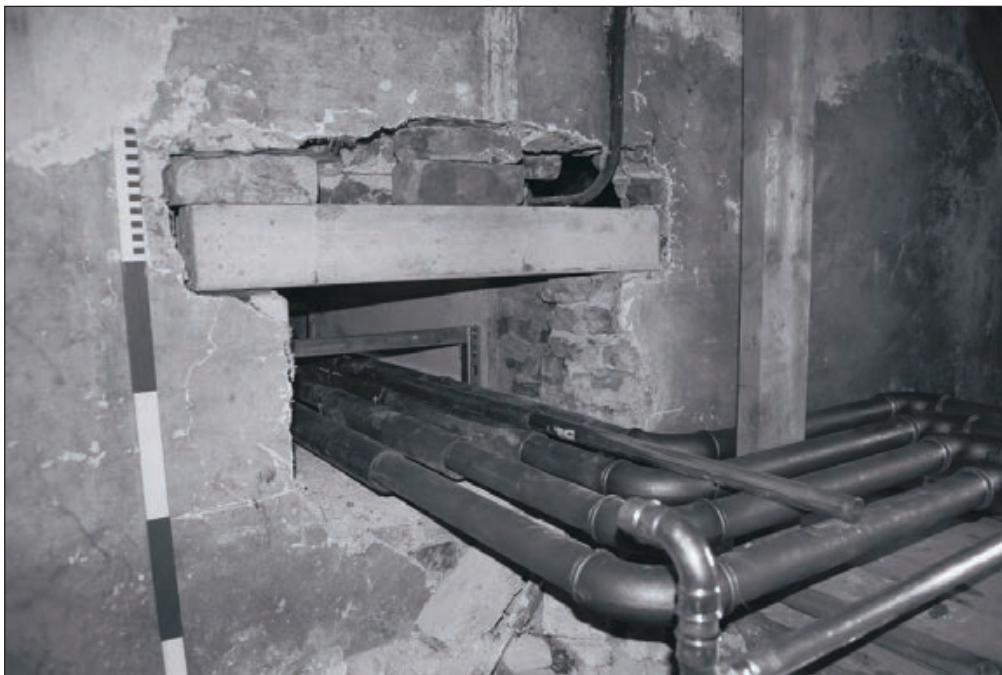
Plate 186: Detail of inserted opening within west wall of F10, Central Entranceway of the North Range, showing exposed brick fabric of wall - OB. 19 (Film 51.34)
