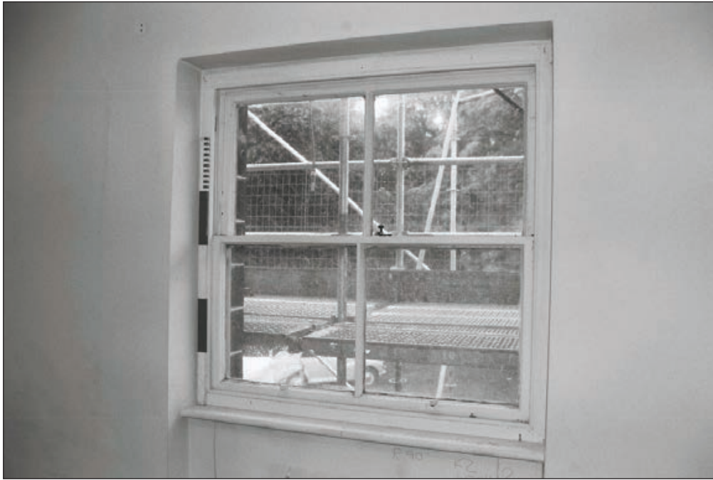
Plate 550: Detail of sash window, F38, South Range - Agent's House (Film 65.12)
