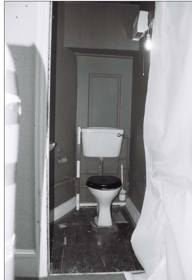
Plate 496: General view of G44, South Range, Agent's House (Film 66.24)
