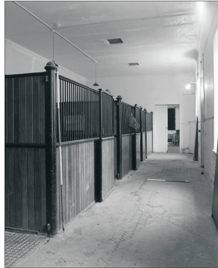
Plate 47: General view of room G2, East Side of the North Range, showing loose boxes (Film 07.05)
