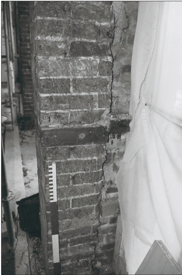
Plate 468: Detail of cut brick of columns, G41, South Range - OB. 106 (Film 73.23)
