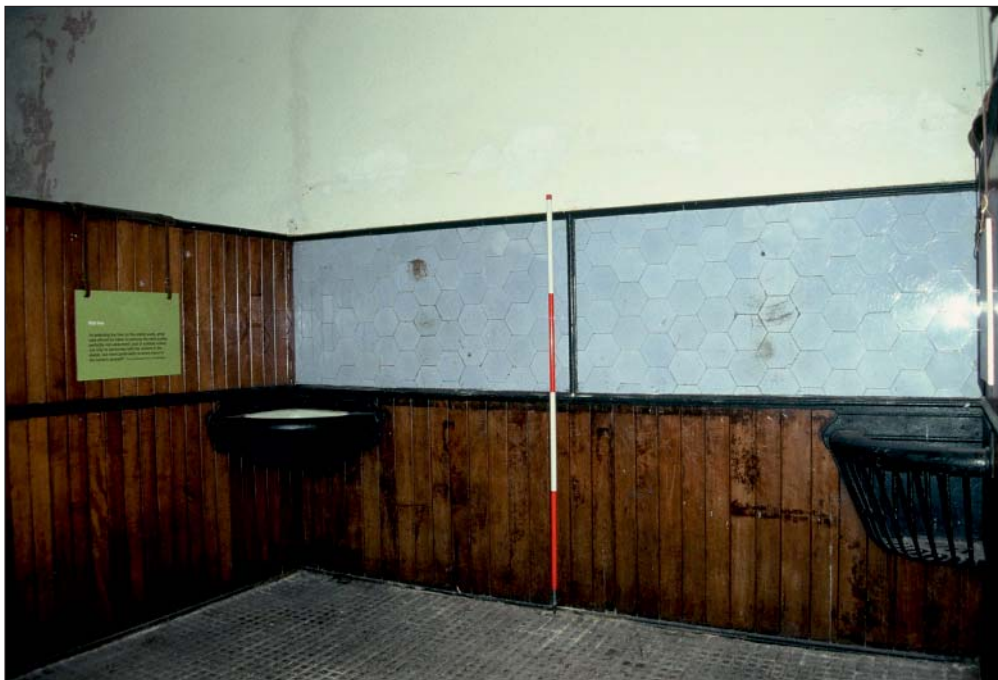
Plate 49: Detail of original loose box within room G2, East Side of the North Range, showing corner manger and trough and coloured hexagonal tiling (Film C.S. 11.)
