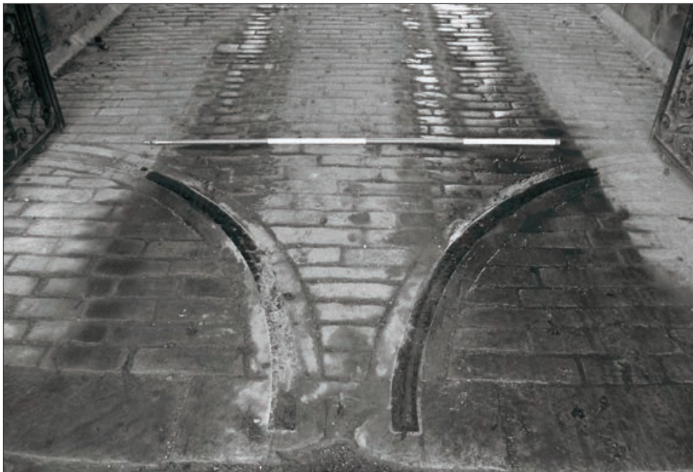
Plate 12: View of stone setted surface of cart passage and gate guides, North Range (Film 20.29)
