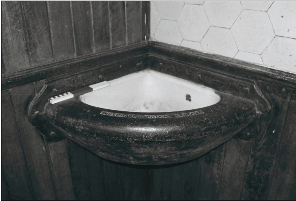
Plate 50: Detail of original Musgrave corner manger, room G2, East Side of the North Range (Film 14.20)
