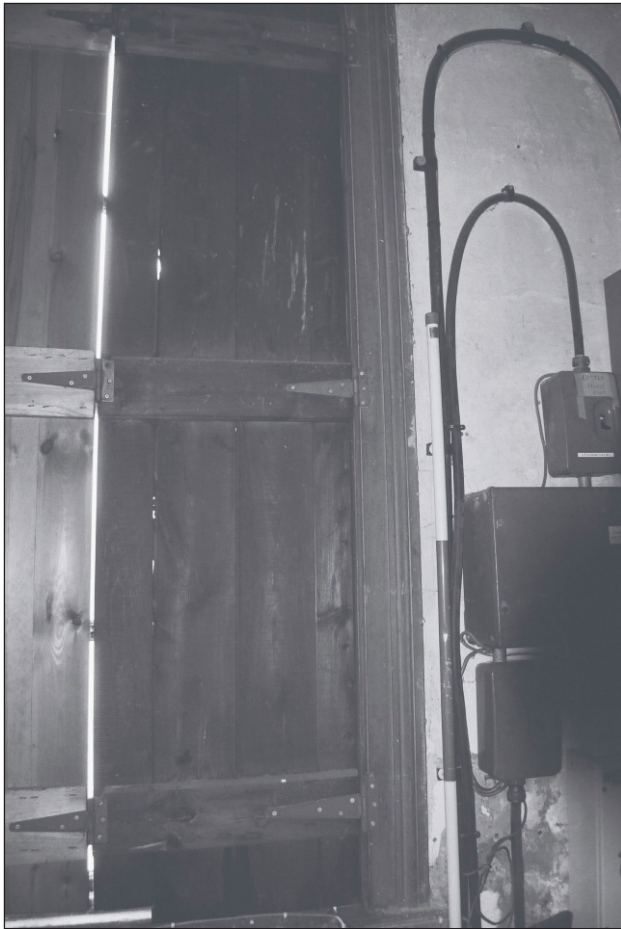
Plate 424: Detail of window shutter, G31, South Range (Film 41.17)
