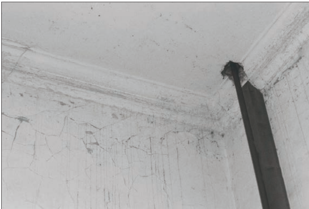
Plate 578: Detail of original cornice, G55, East Range (Film 16.26)
