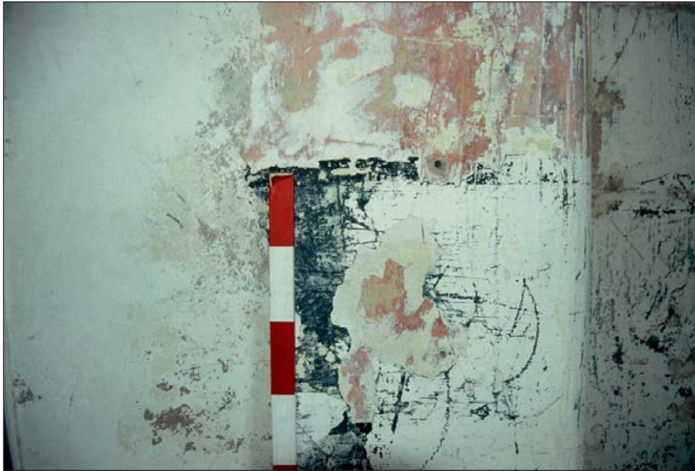
Plate 111: Detail of paint scheme, room G12, West Side of the North Range (Film C.S. 27.)
