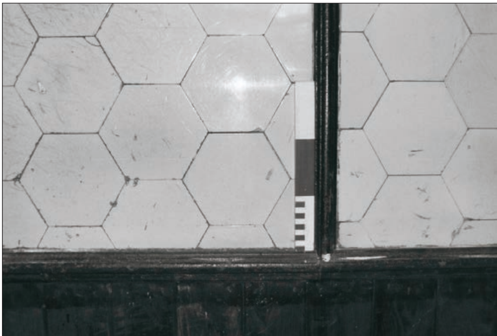
Plate 55: Detail of original stable tiling and cast iron moulded details, room G2, East Side of the North Range (Film 14.24)
