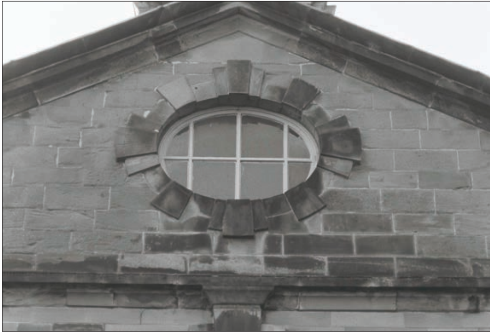
Plate 14: Detail of oeil-de-beuf window, north elevation of the North Range (Film 11.08)
