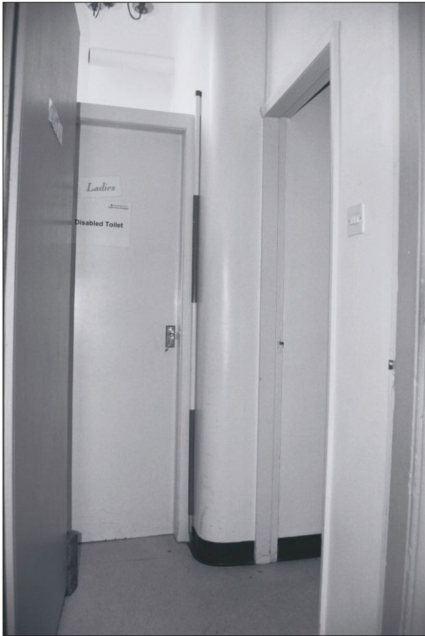
Plate 442: General view of G37, South Range (Film 24.34)
