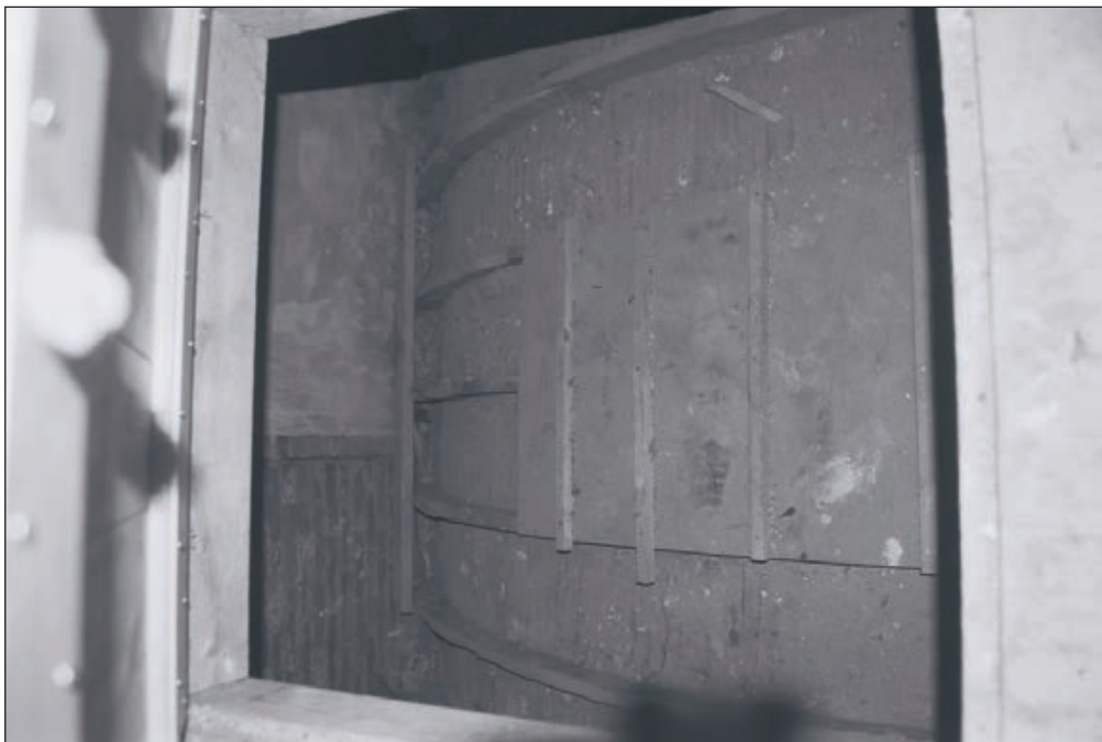
Plate 174: View into F10b down hatch within the floor of F10, Central Entranceway of the North Range, showing inserted arch (Film 42.13)
