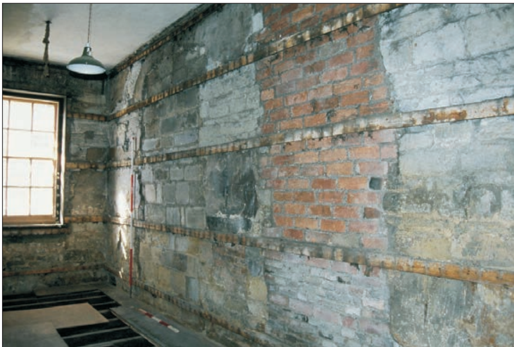
Plate 85: View of room G4, 'Tack Room', Central Entranceway of the North Range, after removal of match boarding, showing blocked openings - OB. 71 & 73 (Film C.S. 34)
