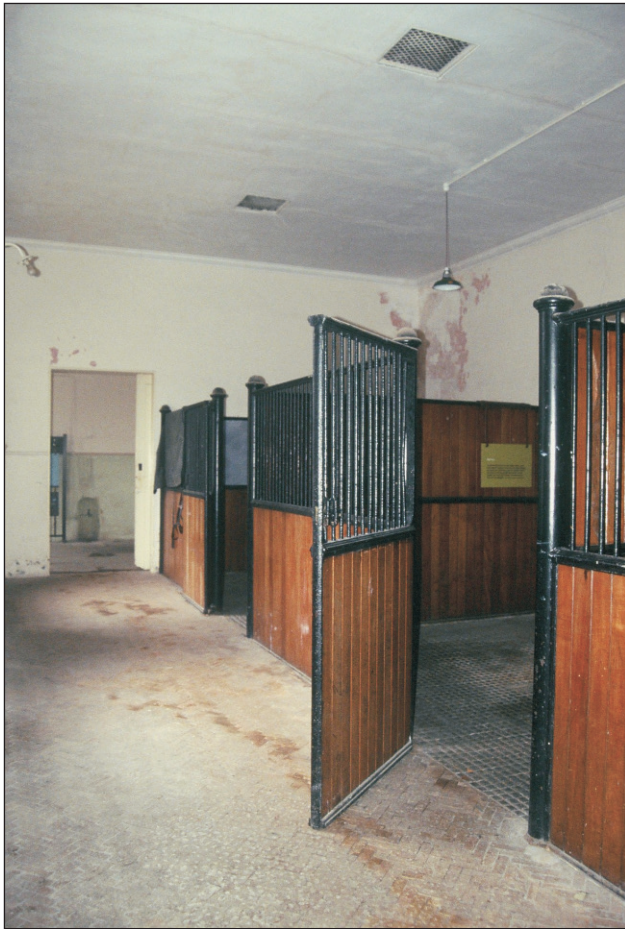
Plate 46: View of room G2 showing original loose boxes, East Side of the North Range (Film C.S. 16)
