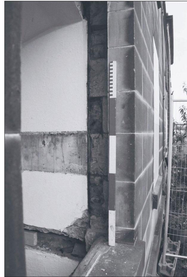
Plate 520: Detail of exposed wall fabric during insertion of door, G52, South Range - Agent's House - OB. 25 (Film 48.29)
