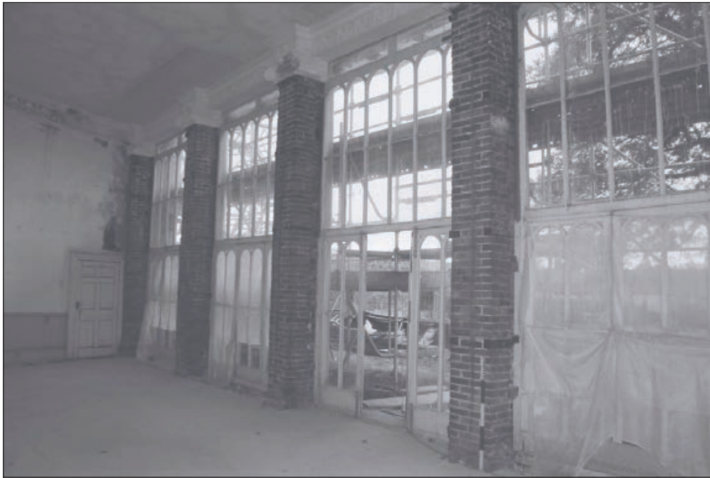
Plate 467: General view of G41, South Range, after removal of timber column surrounds - OB. 106 (Film 74.20)
