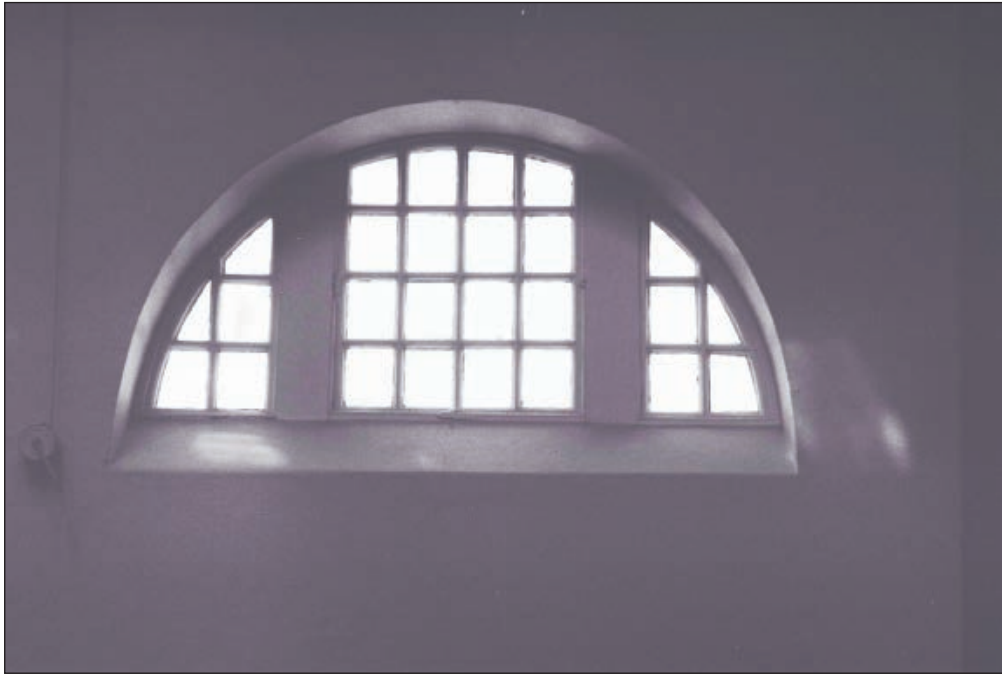
Plate 403: Detail of high window, north wall of G30, South Range (Film 24.18)
