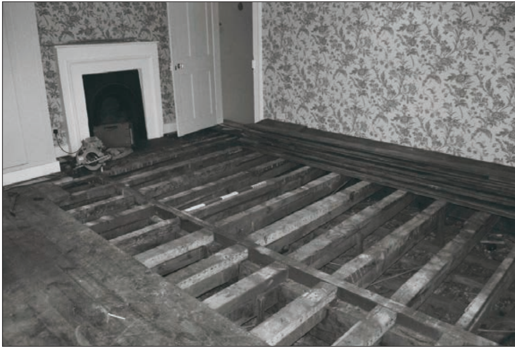
Plate 533: Detail of exposed timber floor and ceiling construction, F35, South Range - Agent's House - OB. 76 (Film 66.19)
