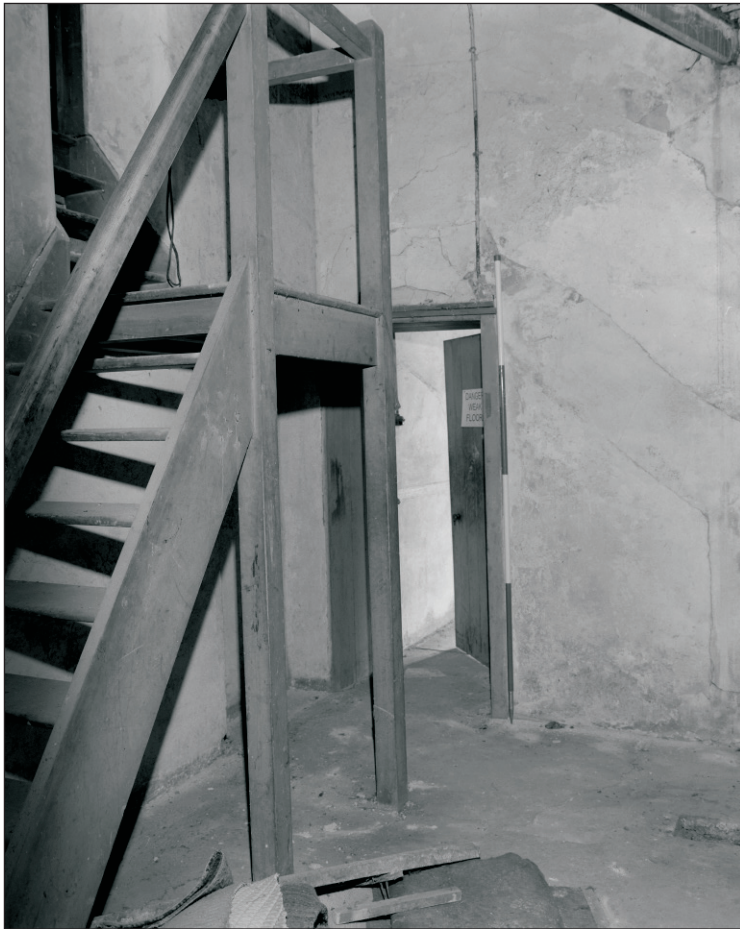
Plate 200: General view of F12, Central Entranceway of the North Range (Film 32.03)
