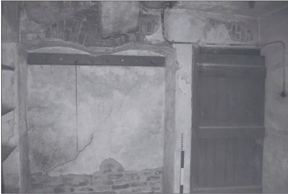
Plate 214: General view of north wall of F13, Central Entranceway of the North Range, showing blocked opening and doorway (Film 74.15)
