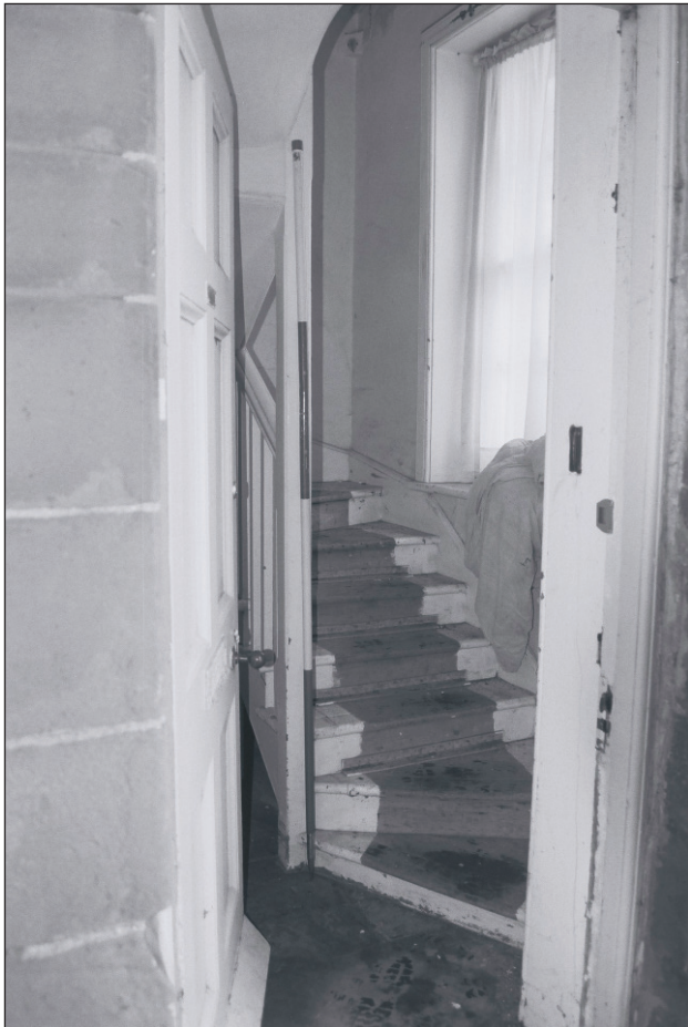
Plate 93: General view of staircase G8, Central Entranceway of the North Range (Film 42.34)
