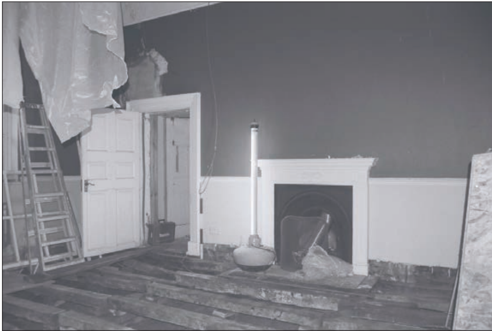
Plate 478: General view of G47, South Range - Agent's House (Film 75.21)
