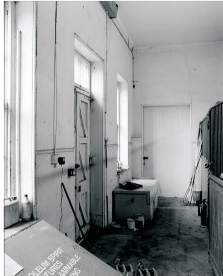
Plate 586: General view of G56, East Range (Film 19.03)
