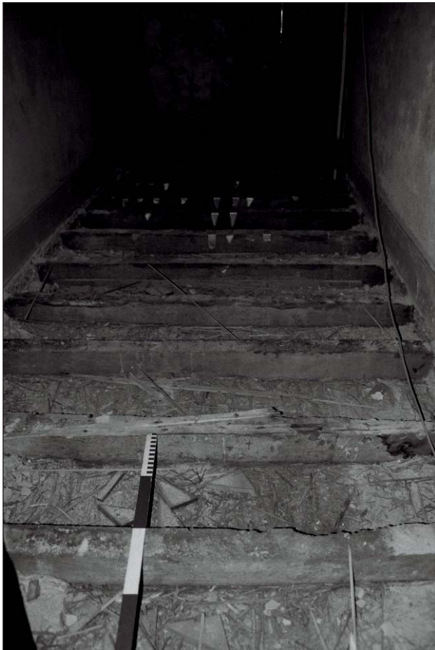
Plate 440: View of exposed timber joists, F30/31, South Range - OB. 90 (Film 70.21)
