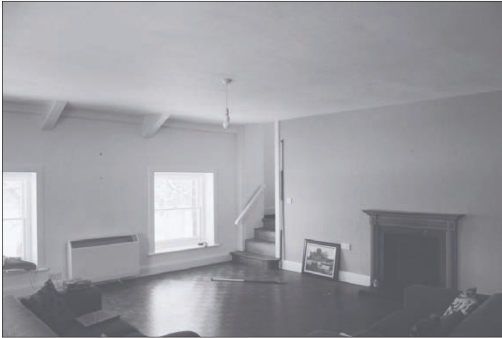
Plate 134: General view of room F1, East Side of the North Range (Film 21.33)
