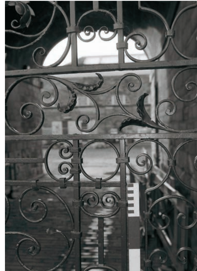
Plate 10: Detail of the North Range cart passage iron gates (Film 12.07)
