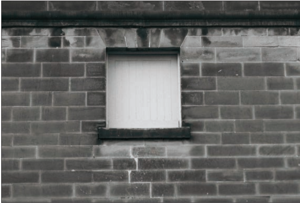
Plate 26: Detail of first floor threshing door within the south elevation of the east end of the North Range (Film 20.37)
