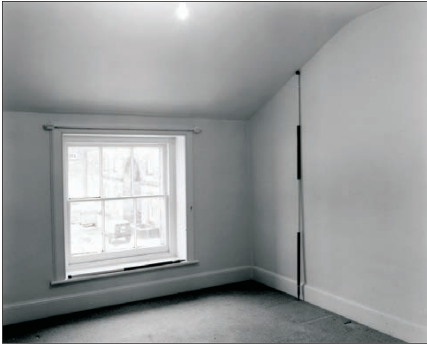
Plate 596: General view of F45, East Range (Film 29.01)
