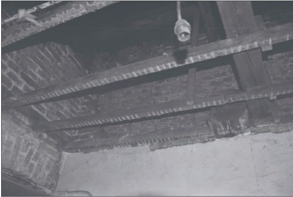
Plate 216: View of exposed ceiling structure, brick fabric of upper walls and timber beams from F10, room F13, Central Entranceway of the North Range (Film 76.19)
