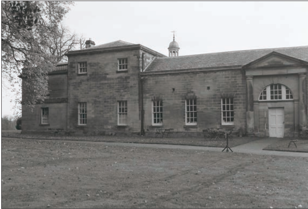
Plate 263: General view of the north end of the west elevation of the North and West Ranges (Film12.21)
