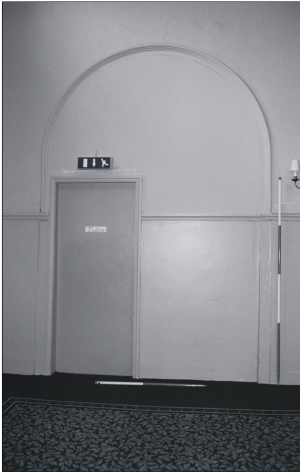
Plate 401: View of blocked arched opening, east wall of G30, South Range (Film 24.22)
