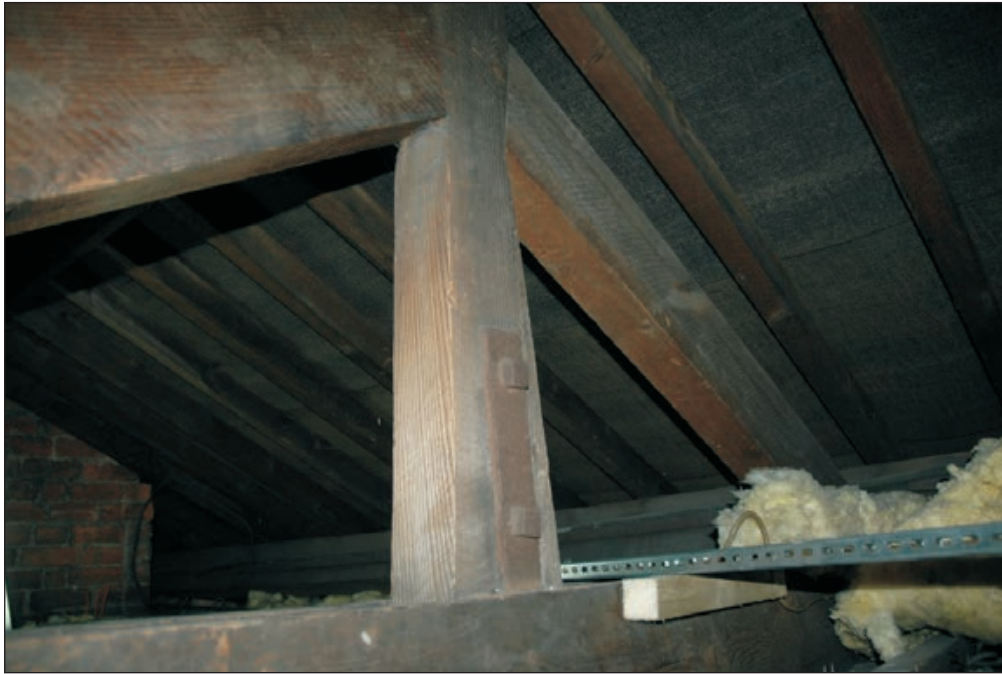
Plate 606: View of timber King-Post roof trusses above East Range, (Film D. 25.02.10 7488)
