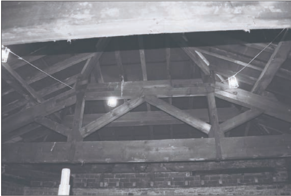
Plate 325: Detail of timber Queen-Post truss, F27, West Range - OB.56 (Film 67.02)
