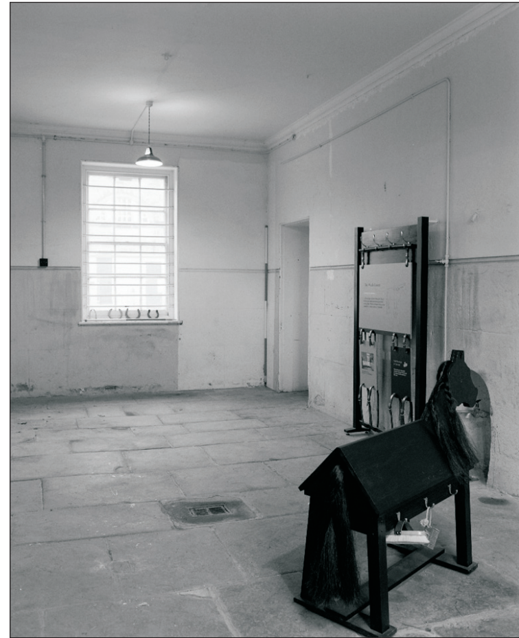
Plate 63: General view of room G3, 'Wash Room', East Side of the North Range (Film 07.09)
