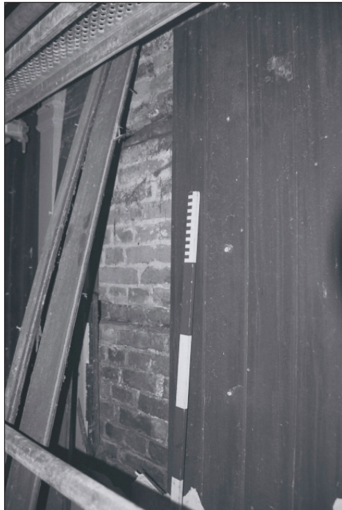
Plate 410: Detail of tongue and groove timber match boarding around lower half of G30 walls, South Range - OB. 69 (Film 56.32)
