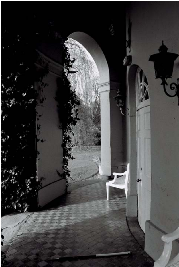
Plate 351: View of bowed/curved loggia (G34), of the south elevation of the Riding House, South Range, looking south-west (Film 13.08)
