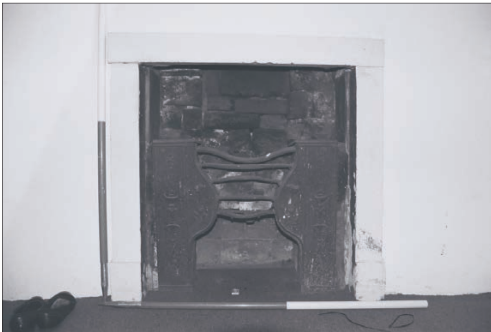
Plate 384: Detail of fireplace, east wall of F28, South Range (Film 22.20)
