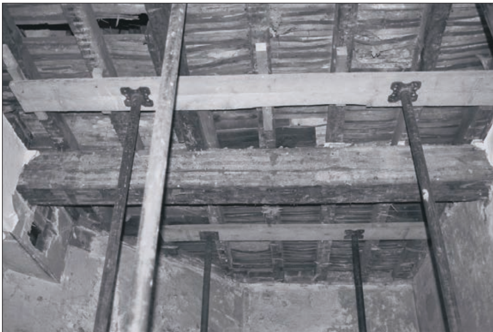
Plate 104: Detail of exposed reused timber beam and joists of floor above room G9/10, Central Entranceway of the North Range (Film 54.27)
