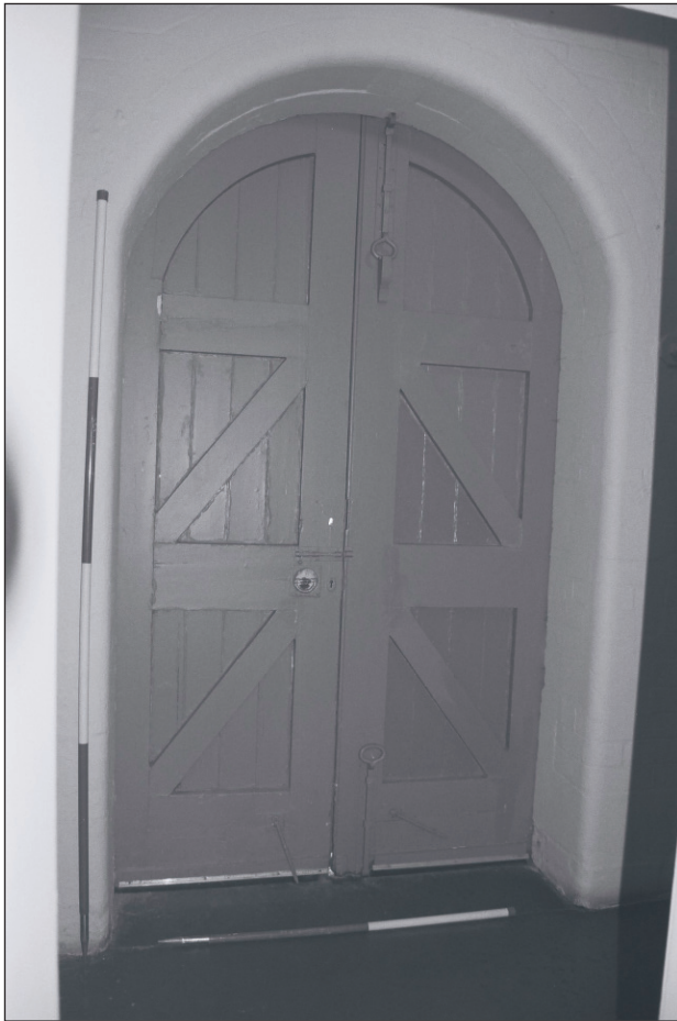
Plate 276: General view doorway, east wall of G19, West Range (Film 23.05)
