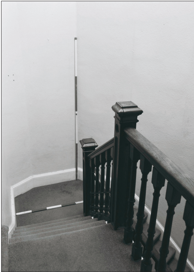
Plate 524: General view of staircase, F34 to G45, South Range - Agent's House (Film 64.07)
