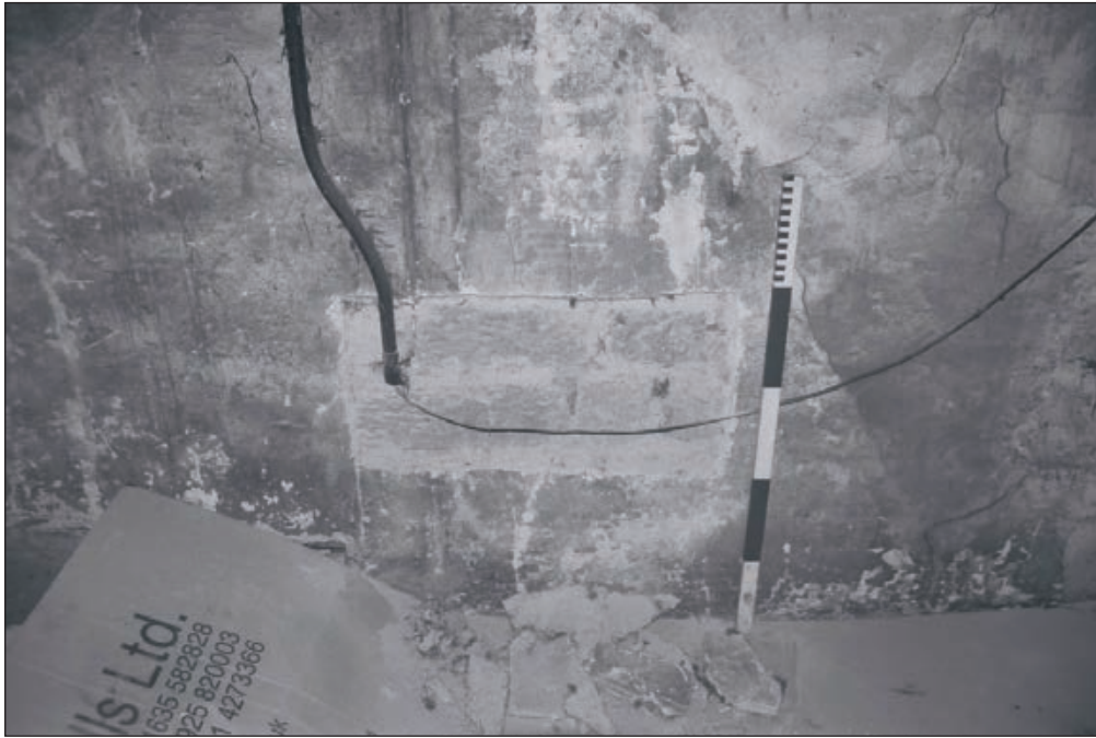
Plate 183: Detail of removed plaster on east wall of F10, Central Entranceway of the North Range, showing exposed stone fabric of wall - OB. 20 (Film 47.23)
