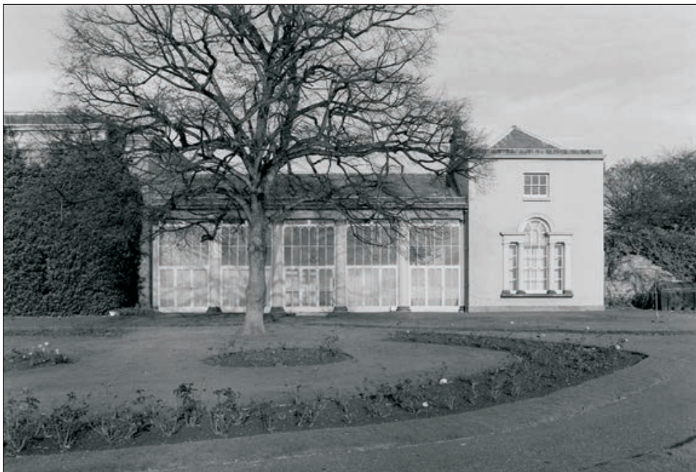
Plate 354: View of the east end of the south elevation of the South Range, showing the Greenhouse and East Pavilion (Film 02.06)
