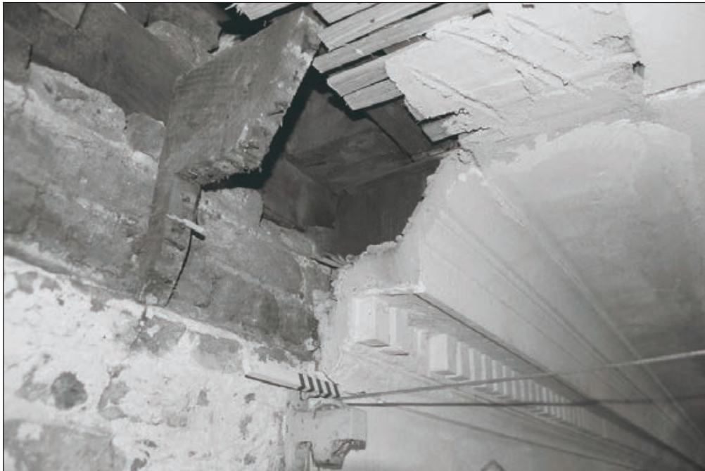
Plate 408: Detail of cornice structure, G30, South Range - OB. 104 (Film 72.12)
