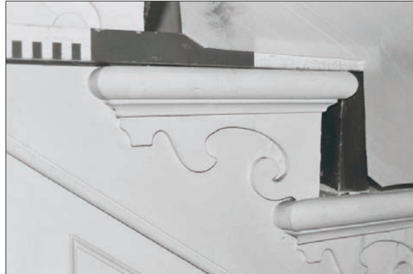
Plate 494: Detail of moulded stair ends, G45, South Range, Agent's House (Film 65.17)
