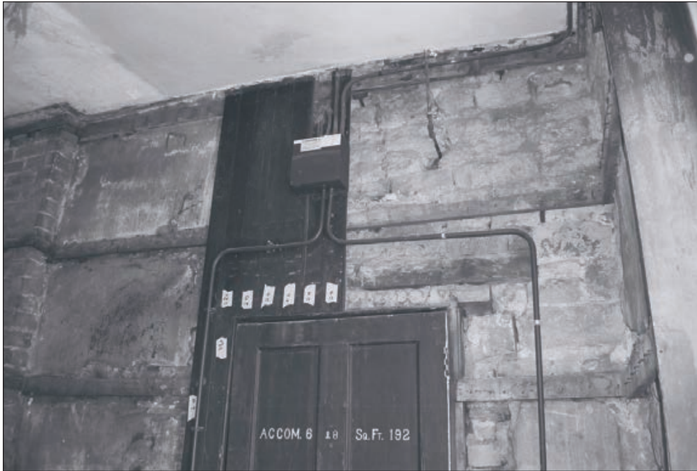
Plate 88: Detail of the south end of east wall showing phase 2 stonework, room G4, 'Tack Room', Central Entranceway of the North Range - OB. 71 & 75 (Film 57.15)
