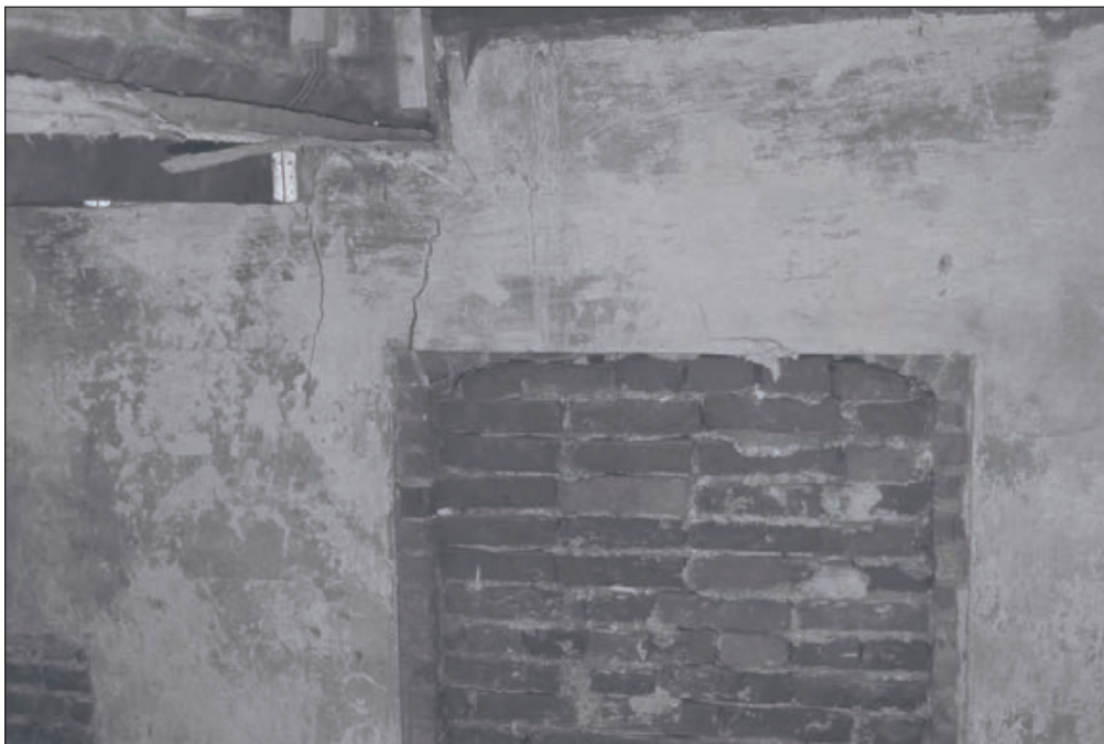
Plate 166: View of blocked doorway with F11 in west wall of F10b, Central Entranceway of the North Range - OB. 87 (Film 75.29)
