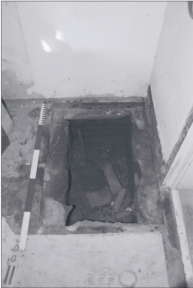
Plate 515: Detail of floor construction, G51, South Range - Agent's House - OB. 88 (Film 68.07)
