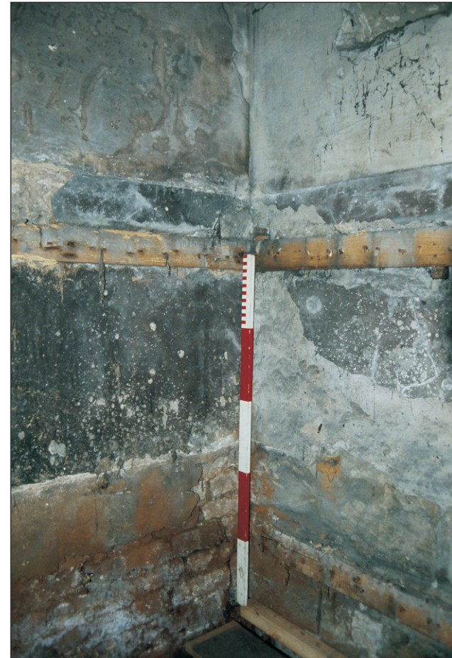
Plate 91: Detail of phase 2 paint scheme on exposed plastered walls of room G4, 'Tack Room', Central Entranceway of the North Range - OB. 73 & 76 (Film C.S. 37)
