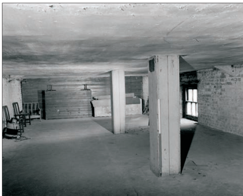
Plate 137: General view of room F2, East Side of the North Range (Film 05.10)
