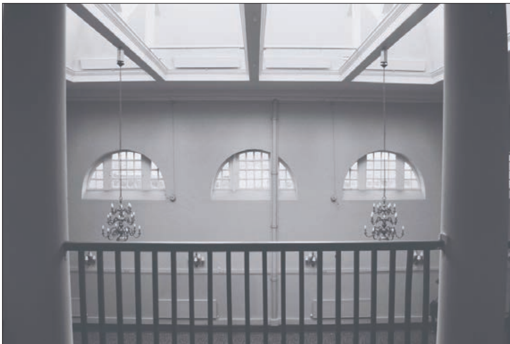
Plate 435: General view of G30 from balcony F32, South Range (Film 46.34)
