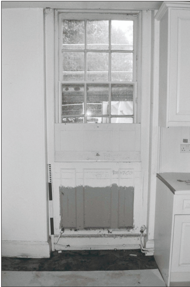
Plate 513: Detail of sash window with lifting shutter, east wall of G51, South Range - Agent's House (Film 65.29)
