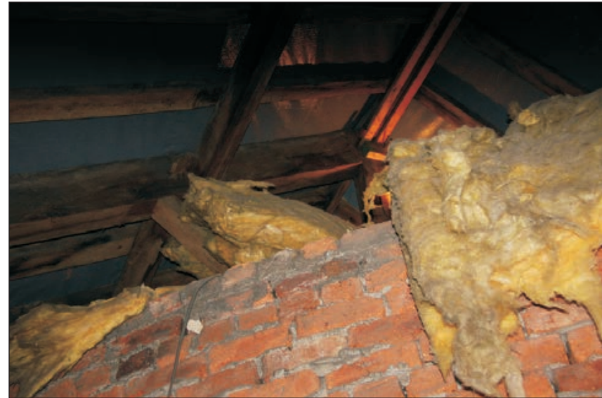
Plate 476: View of curved brick wall and timber King-Post roof trusses above, from roof void above G36, South Range - OB. 111 (Film D. 21.10.11 5051)
