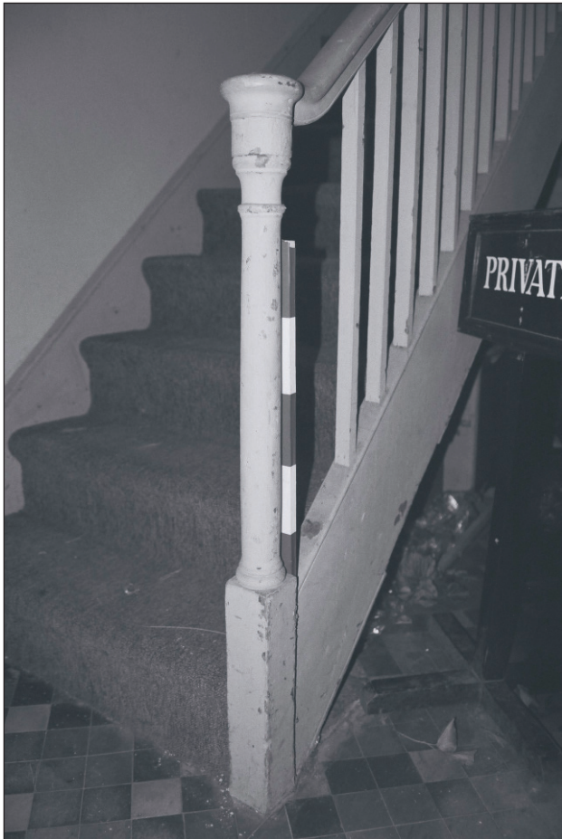
Plate 426: Detail of staircase, G35, South Range (Film 41.10)
