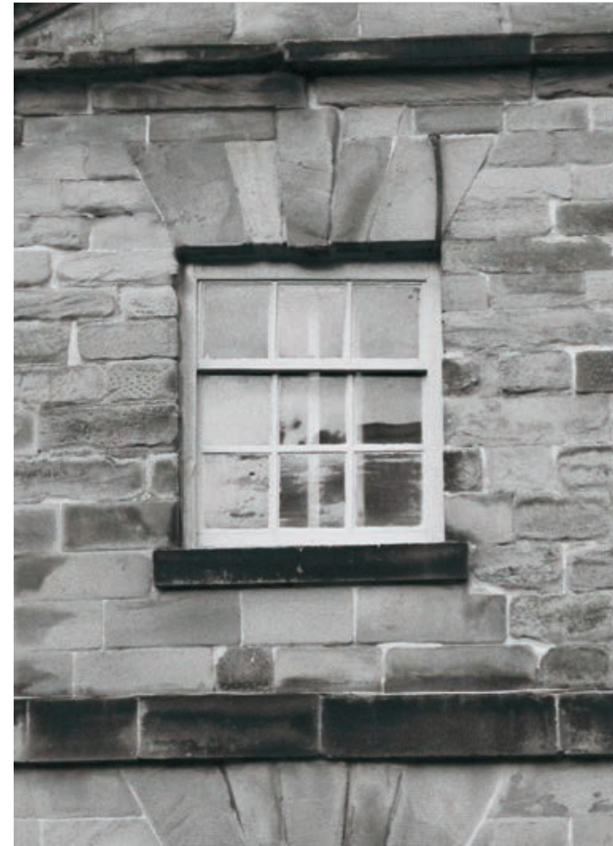
Plate 17: Detail of first floor window, south elevation of North Range (Film 16.35)
