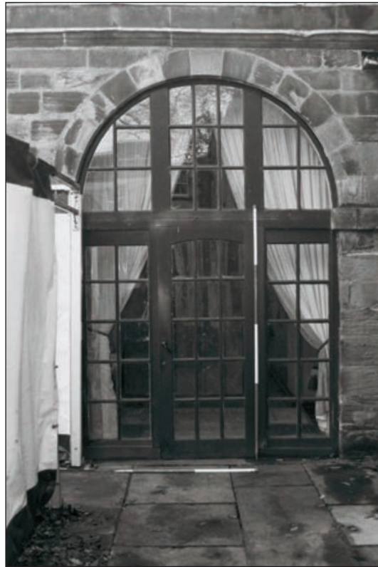
Plate 360: Detail of archway and modern glazing within the north courtyard elevation of the Garden Room, South Range (Film 20.17)
