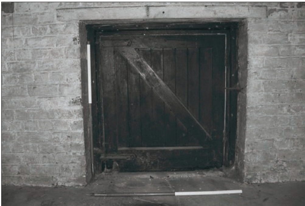
Plate 141: Detail of threshing door, room F2, East Side of the North Range (Film 16.14)
