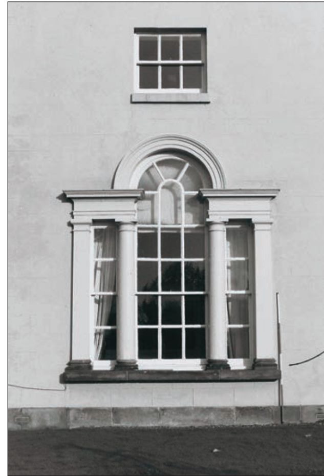
Plate 358: Detail of the fenestration of the south elevation of the East Pavilion, South Range (Film 13.12)
