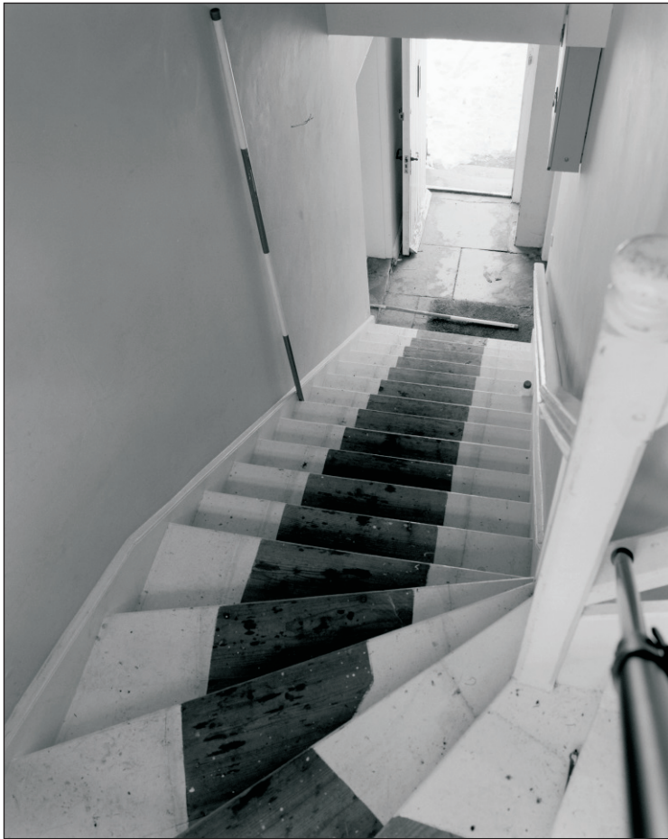
Plate 589: General view of staircase leading from F42 to G53, South/East Range (Film 30.01)
