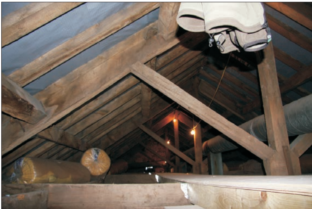
Plate 392: General view of roof void above G28, South Range, showing timber King-Post trusses - OB. 112 (Film D. 21.10.11 5072)
