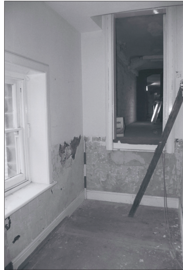
Plate 153: View of room F5, East Side of the North Range, showing break in limeash floor - OB. 124 (Film 77.10)
