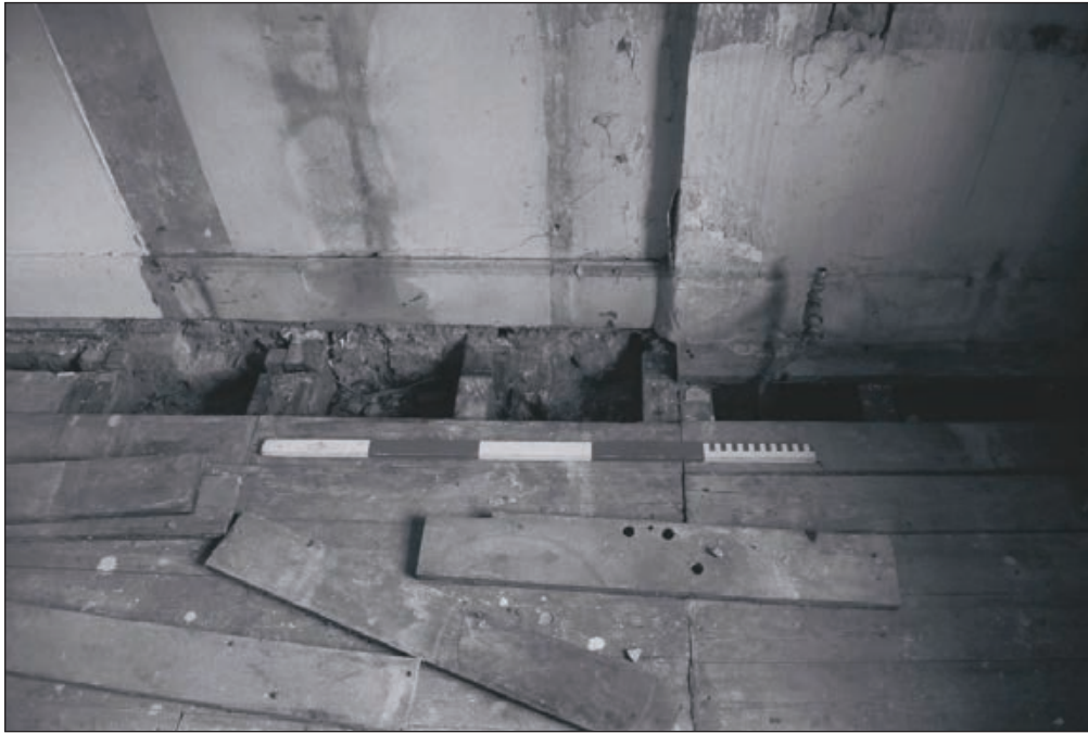
Plate 162: Detail of removed floorboards, exposed timber joists and east wall, room F9, Central Entranceway of the North Range - OB. 122 (Film 77.13)
