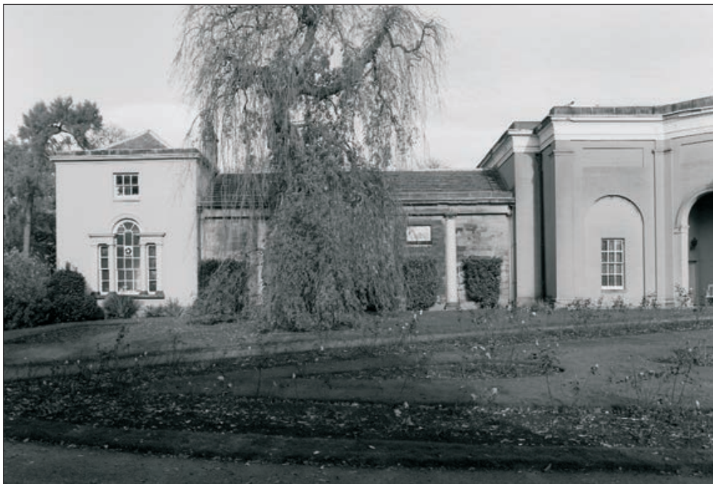
Plate 338: View of the west end of the south elevation of the South Range (Film 02.07)
