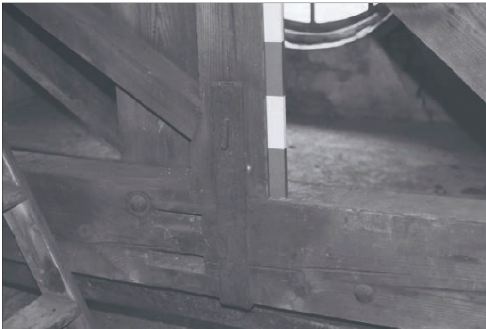
Plate 176: Detail of iron strapping and former joint in timbers of clock tower structure, F10, Central Entranceway of the North Range (Film 42.18)
