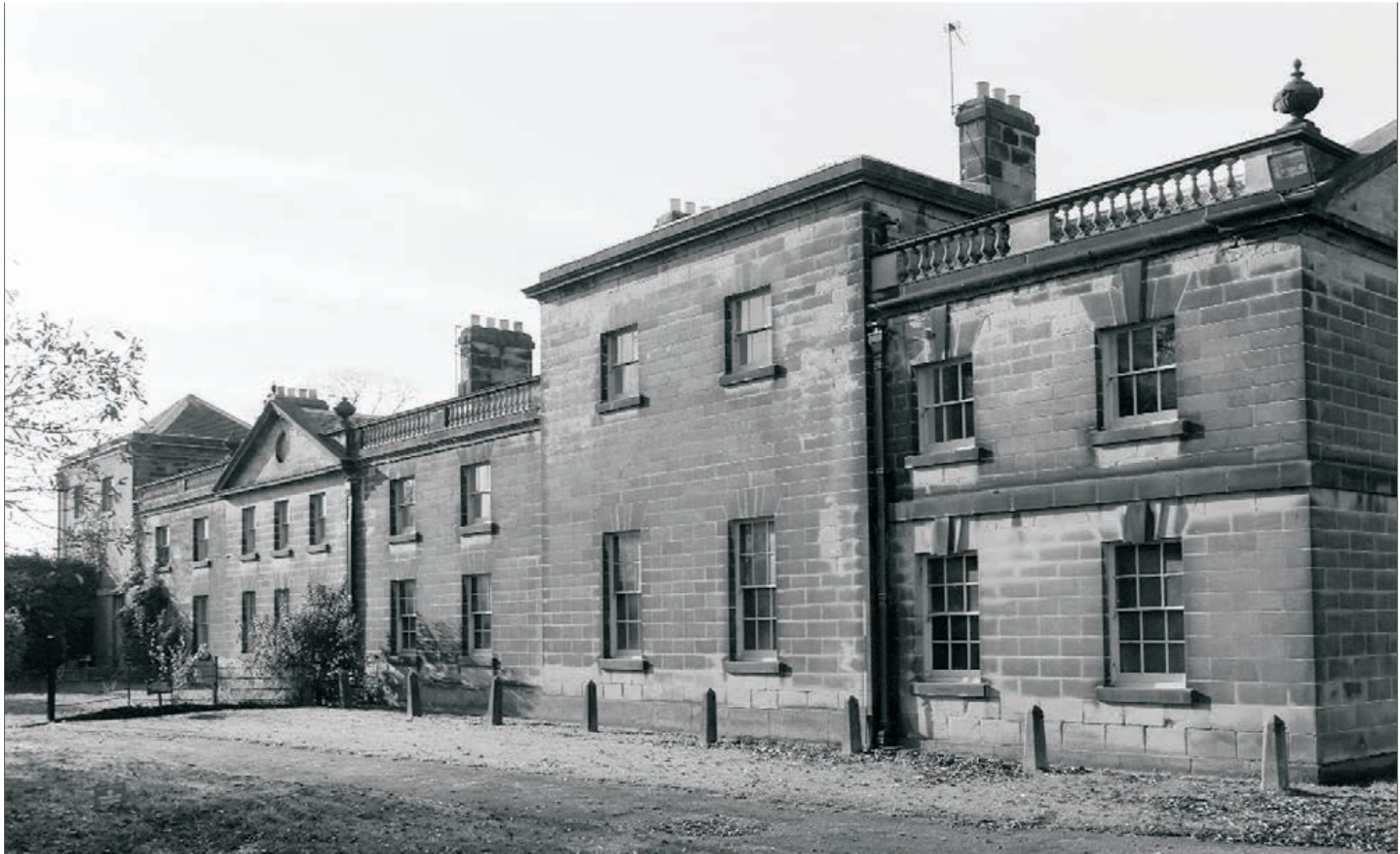
Plate 561: General view of the east elevation of the South, East and North Ranges, looking southwest (Film 01.06)
