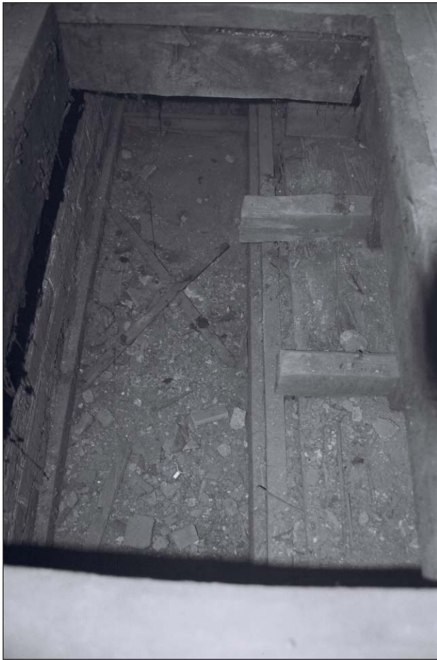
Plate 331: View of into hatch in floor of Roof Void 8, West Range - OB. 98 - showing ceiling construction and former chute (Film 78.17)
