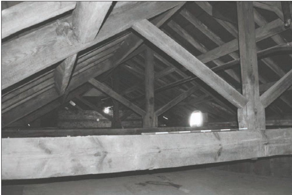
Plate 326: General view of Roof Void 8, West Range - OB. 98 (Film 71.19)
