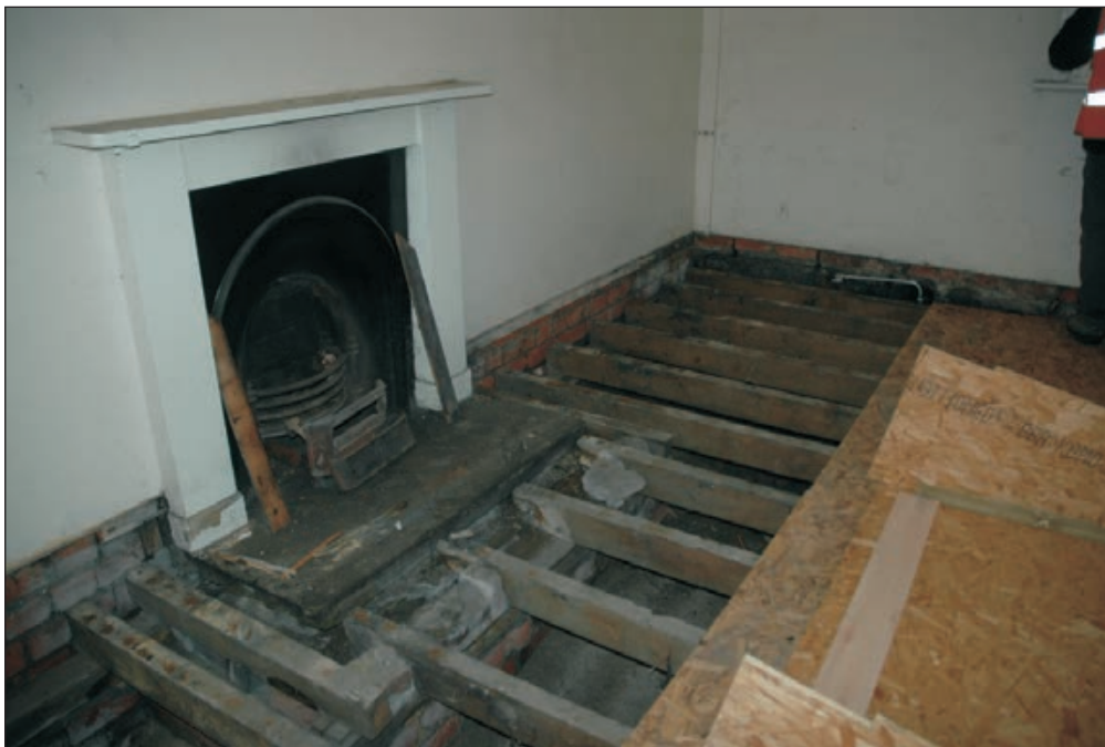
Plate 574: Detail of exposed timber joists, G54, East Range (Film D.03.03.10 7626)
