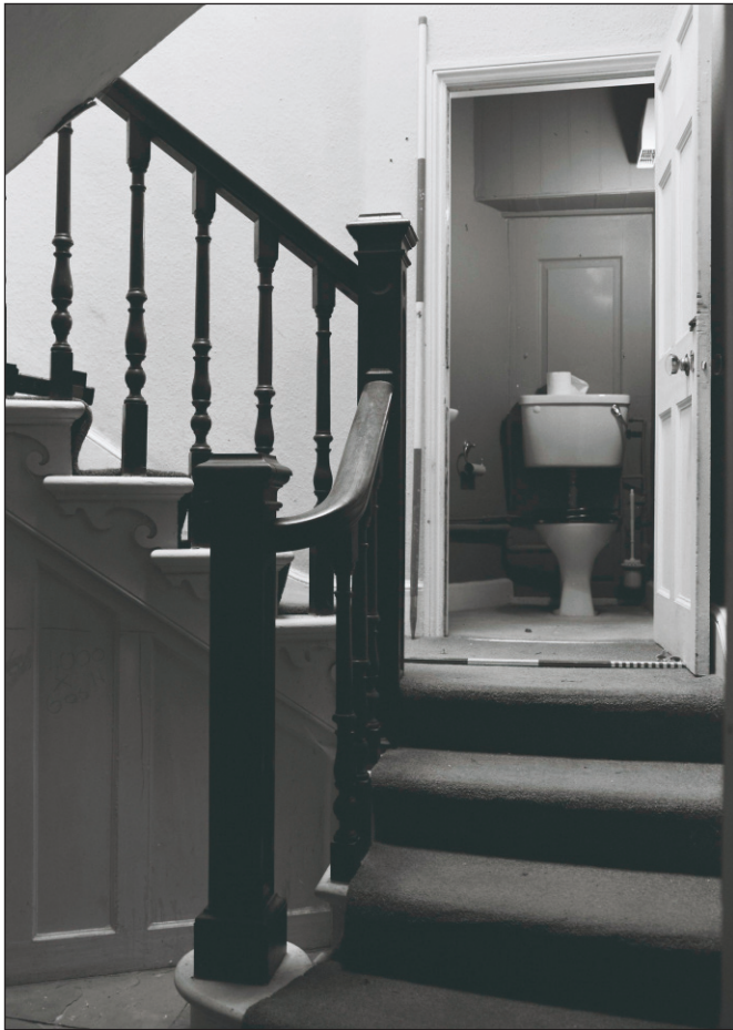
Plate 491: General view of staircase G45, South Range - Agent's House, with G44 beyond (Film 61.05)
