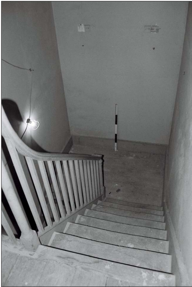
Plate 430: View of staircase from F33, South Range, showing timber treads and half landing ,South Range (Film 70.17)
