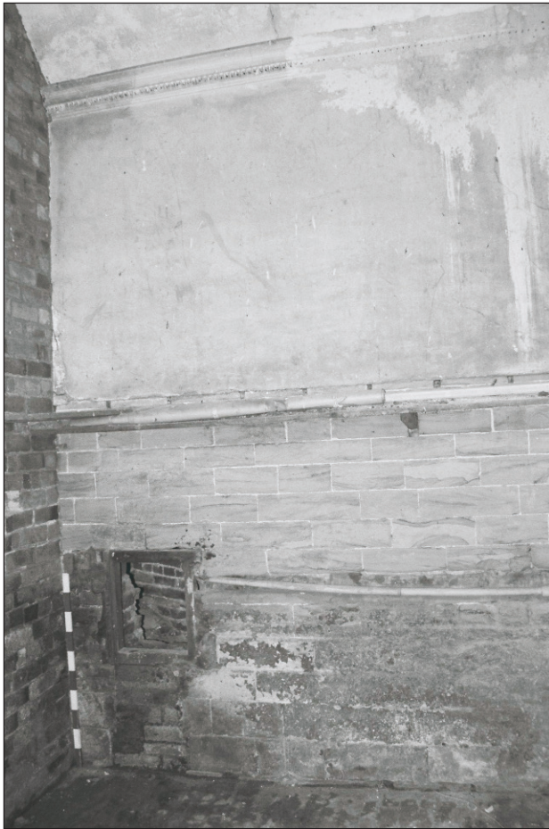
Plate 448: General view of G42, South Range, showing small inserted opening within the south wall - OB. 45 (Film 71.36)
