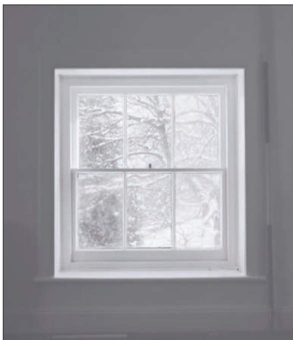
Plate 136: Detail of sash window, room F1, East Side of the North Range (Film 21.29)
