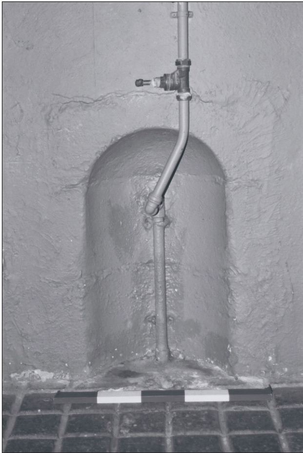
Plate 301: Detail of recessed drain, north wall of G23, West Range (Film 23.28)
