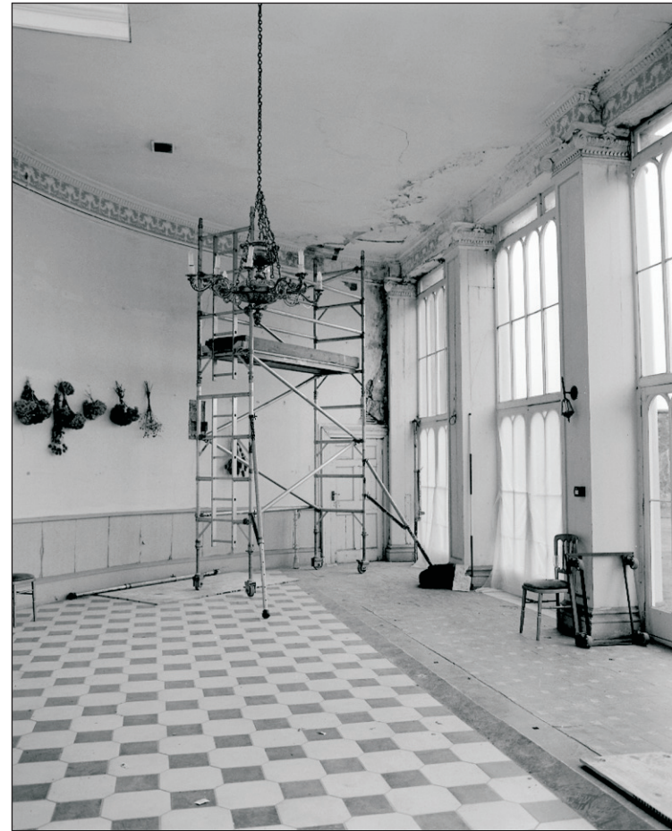
Plate 457: General view of G41, South Range (Film 08.10)
