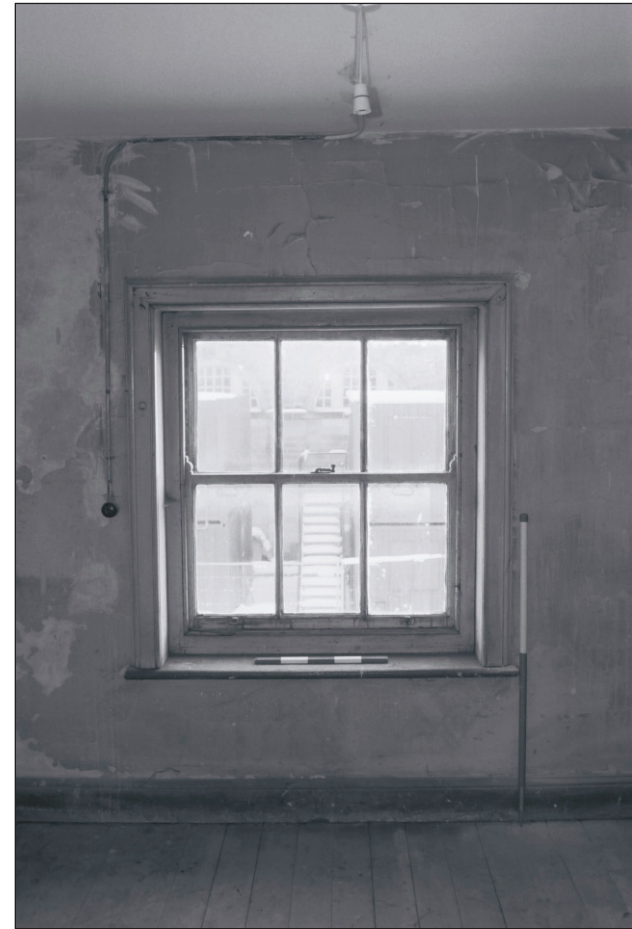
Plate 229: Detail of sash window in south wall of room F15, West Side of the North Range (Film 25.22)
