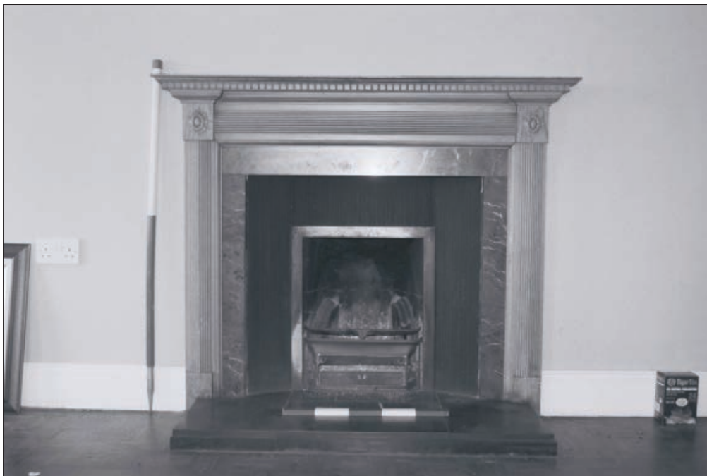
Plate 135: Detail of fireplace, room F1, East Side of the North Range (Film 21.30)
