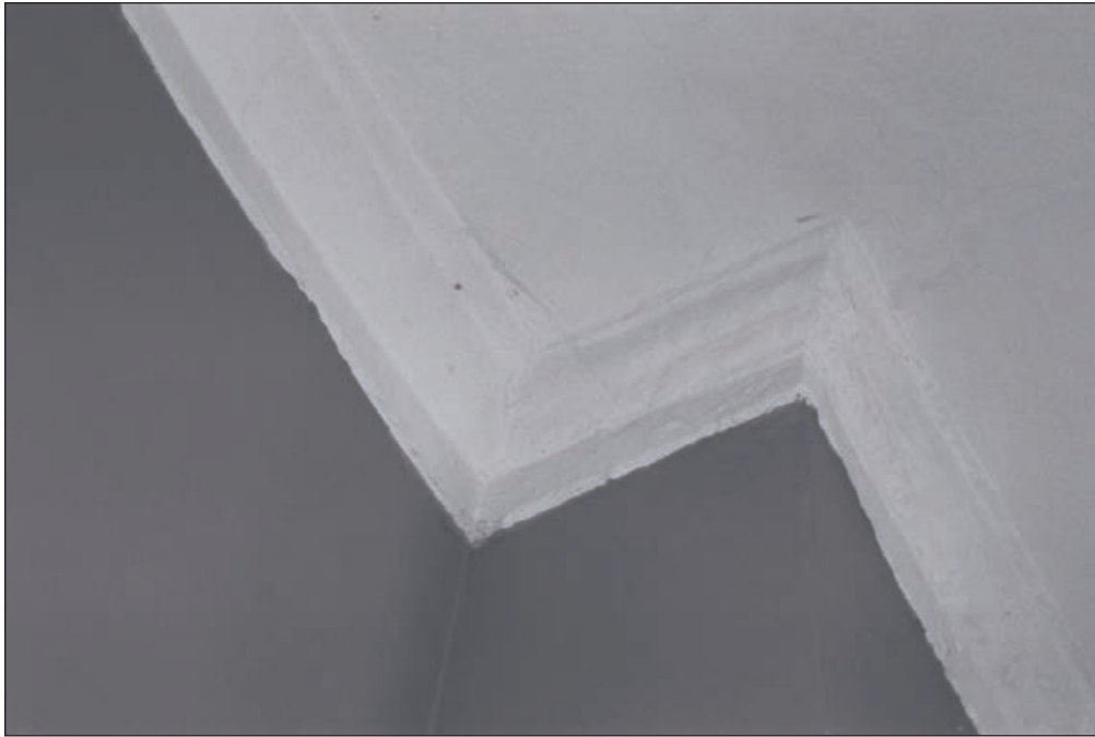
Plate 307: Detail of cornice, G24, West Range (Film 22.10)
