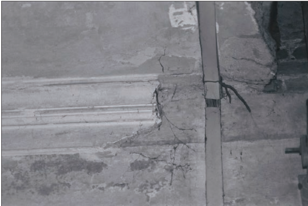
Plate 423: Detail of original cornice, G31, South Range (Film 41.15)
