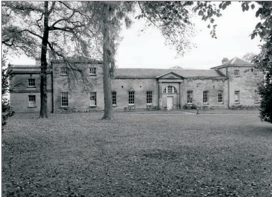
Plate 6: General view of west elevation of West Range from the northwest (Film 03.02)
