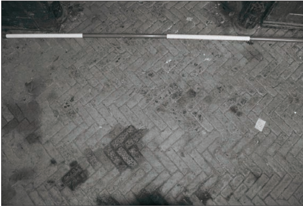
Plate 577: Detail of herringbone brick floor, G55, East Range (Film 16.20)
