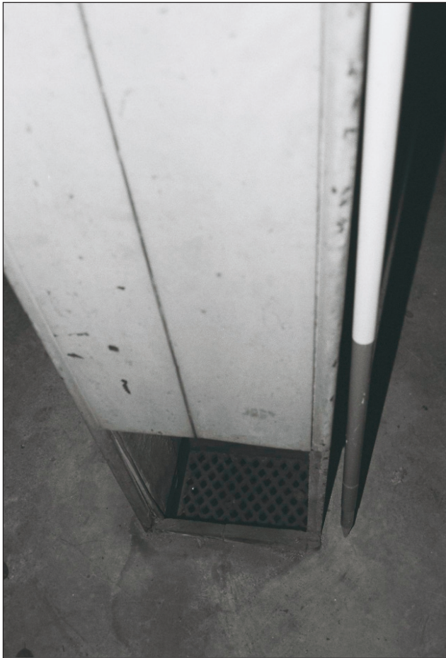
Plate 142: Detail of vent from ceiling of G2 through room F2, East Side of the North Range (Film 16.16)
