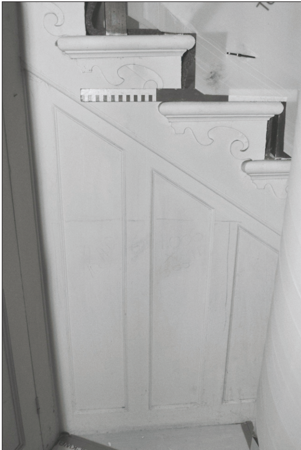
Plate 493: Detail of decorative panels and stair-ends of staircase, G45, South Range - Agent's House (Film 65.16)
