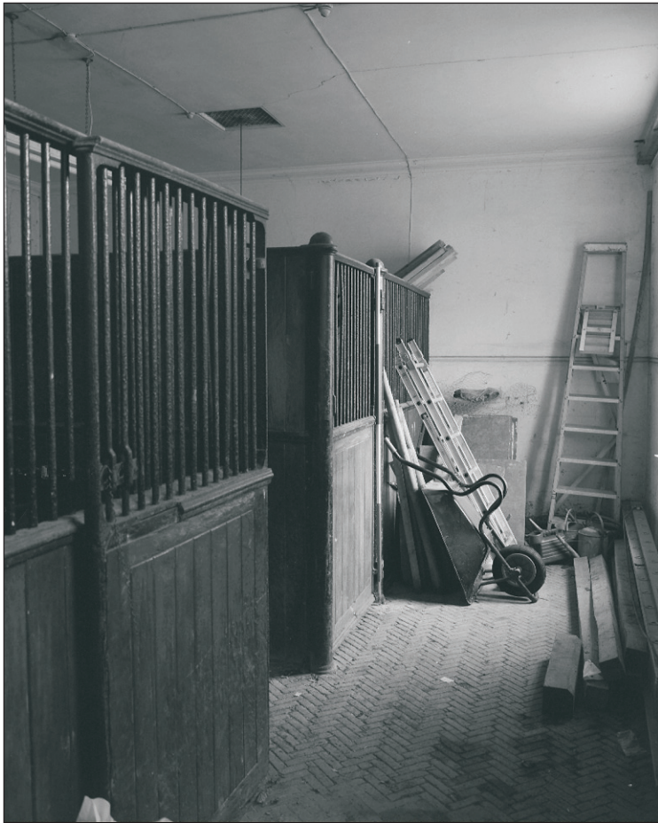
Plate 575: General view of G55, East Range (Film 19.06)
