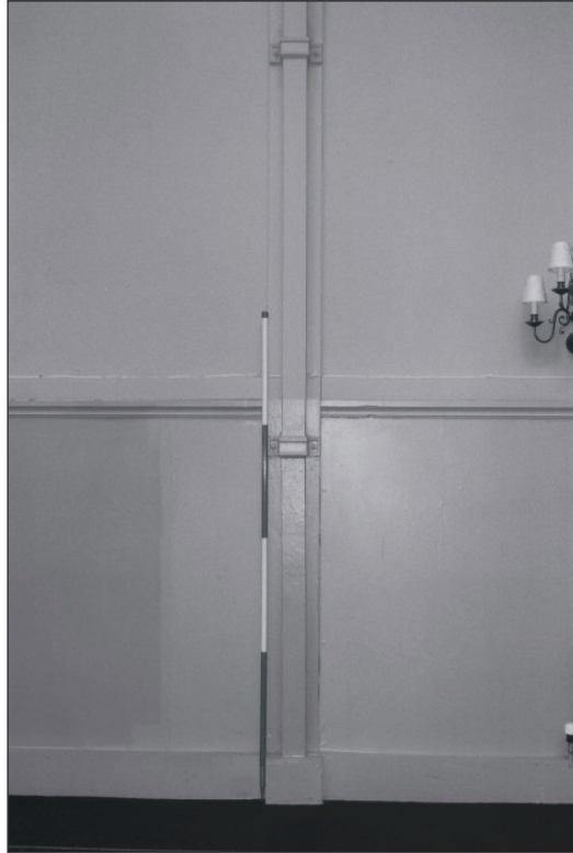
Plate 405: Detail of internal downpipe, north wall of G30, South Range (Film 24.13)
