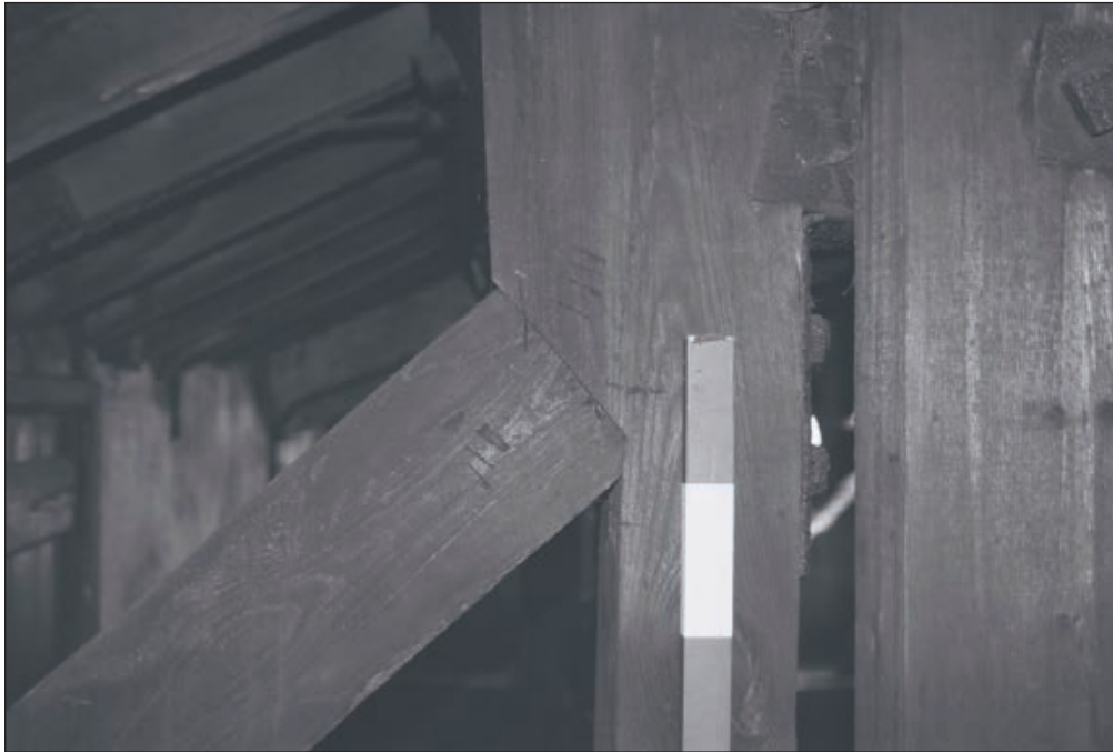
Plate 179: Detail of construction marks on timber clock tower structure, F10, Central Entranceway of the North Range (Film 42.26)
