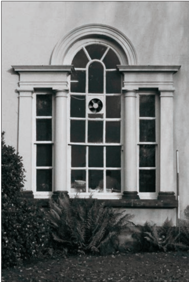
Plate 340: Detail of ground floor window with blind outer lights, south elevation of the West Pavilion of the South Range (Film 12.27)
