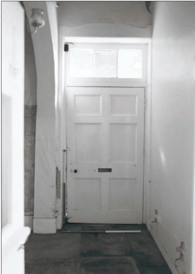
Plate 97: General view of corridor G10, Central Entranceway of the North Range, showing primary doorway from cart passage G7 (Film 50.02)
