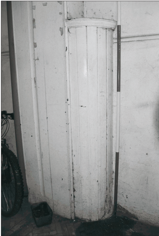
Plate 587: Detail of timber casing, south-west corner of G56, East Range (Film 16.31)
