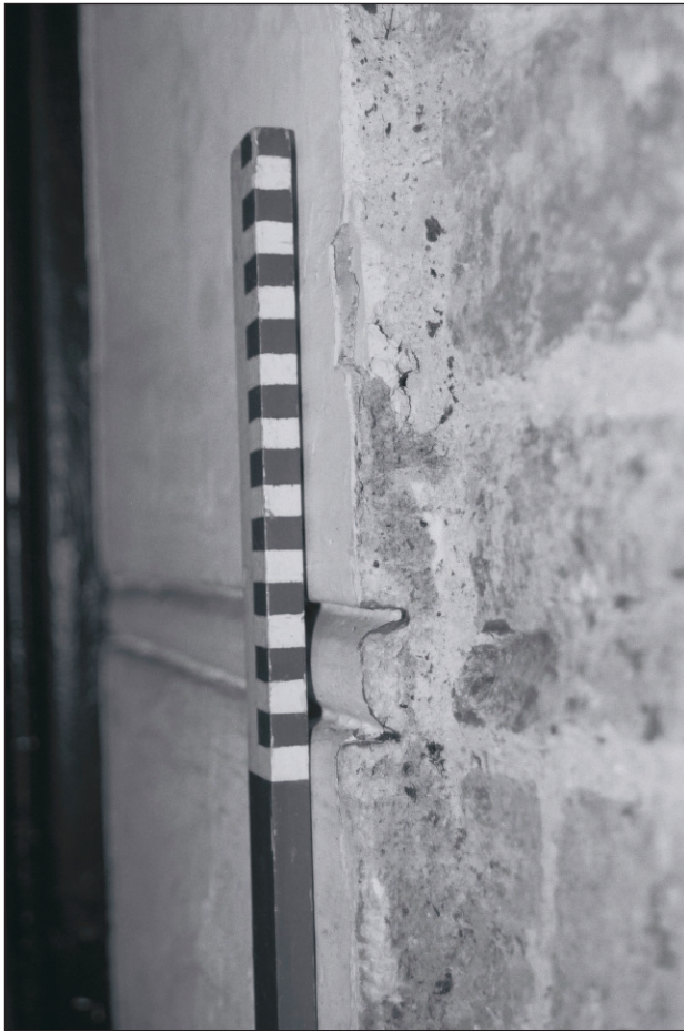
Plate 583: Detail of moulded wall plaster, G55, East Range (Film 45.33)
