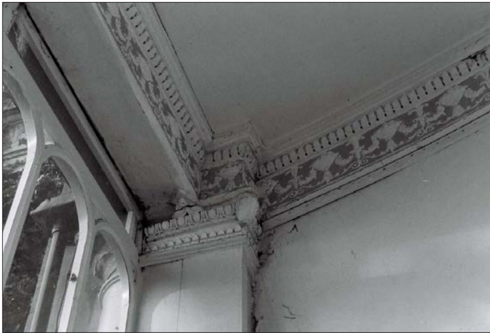
Plate 464: Detail of original cornice and column head, G41, South Range (Film 13.19)
