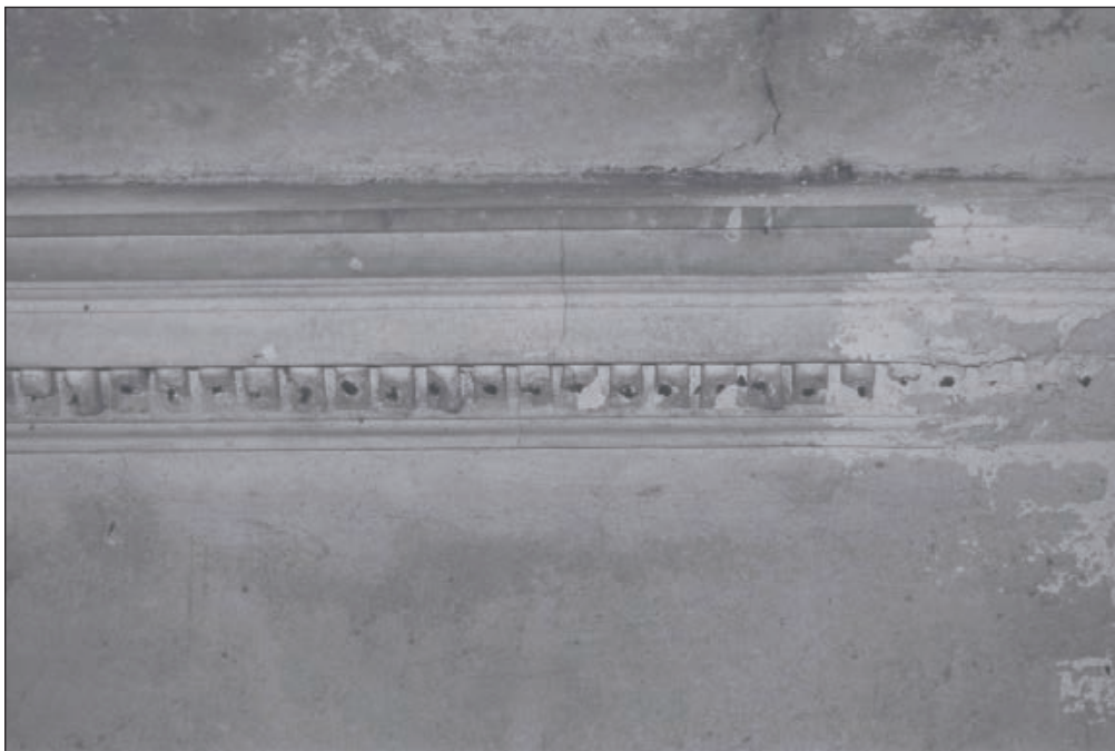
Plate 453: Detail of original cornice, G42, South Range (Film 74.33)
