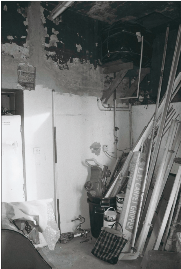
Plate 473: General view of G36, South Range (Film 13.26)
