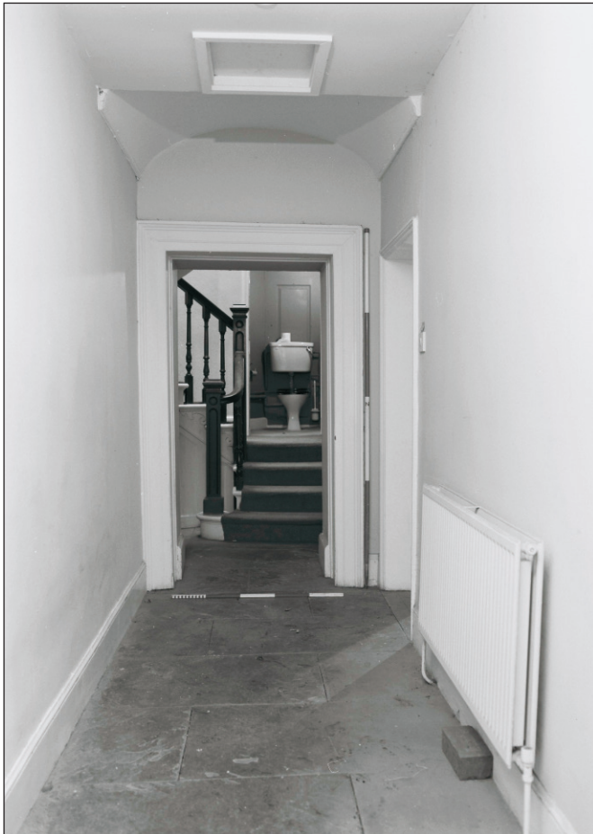
Plate 487: General view of corridor G48, South Range - Agent's House (Film 60.03)
