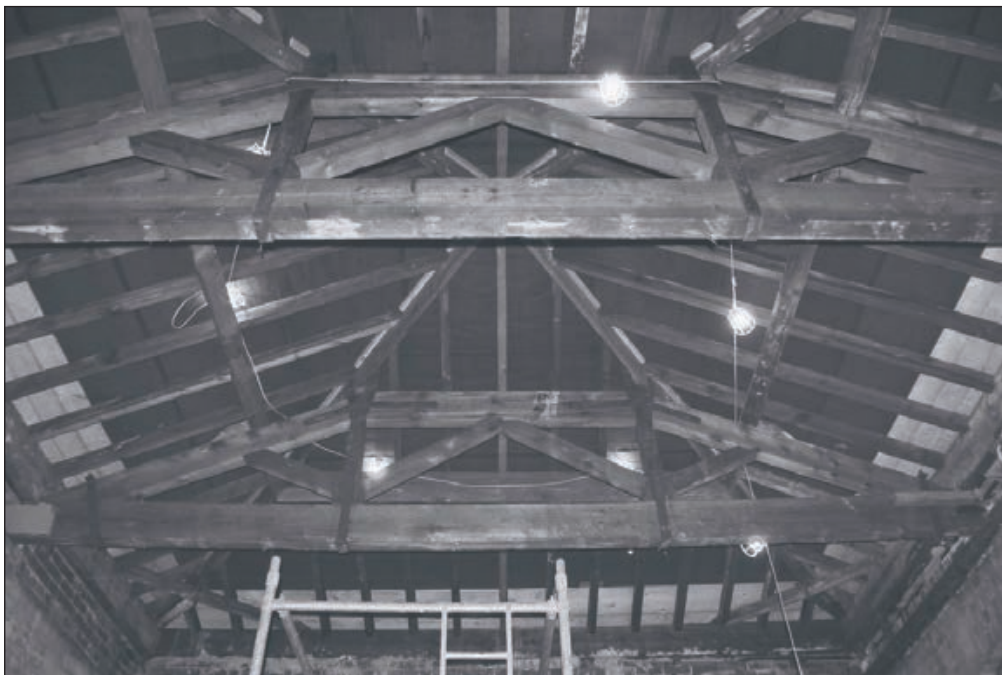
Plate 324: General view of exposed timber Queen-Post trusses, F27, West Range - OB. 56 (Film 67.08)
