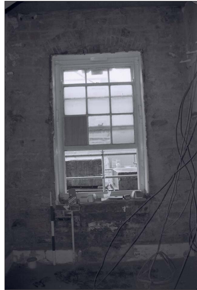
Plate 108: Detail of exposed stonework & raised sill of window, south wall of G11, Central Entranceway of the North Range - OB. 116 (Film 76.31)
