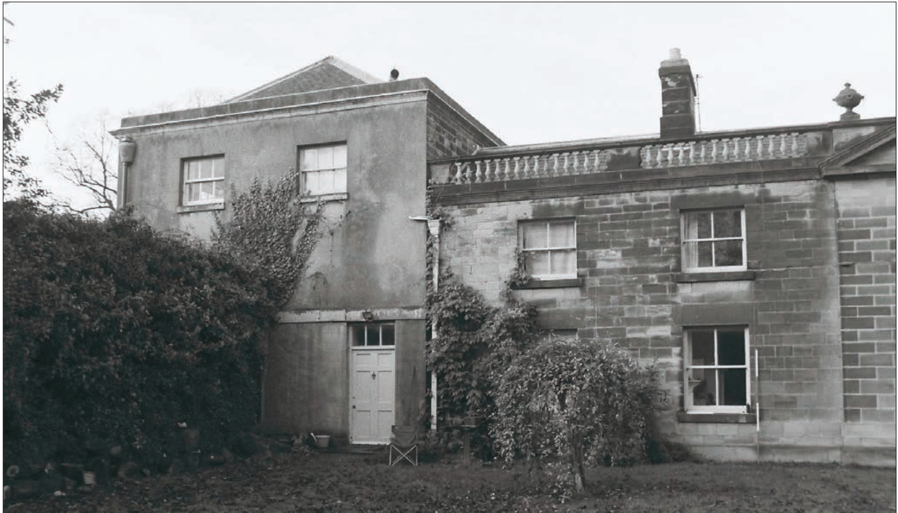
Plate 366: General view of the south end of the east elevation of the South and East Ranges (Agent's House), looking southwest (Film 11.34)
