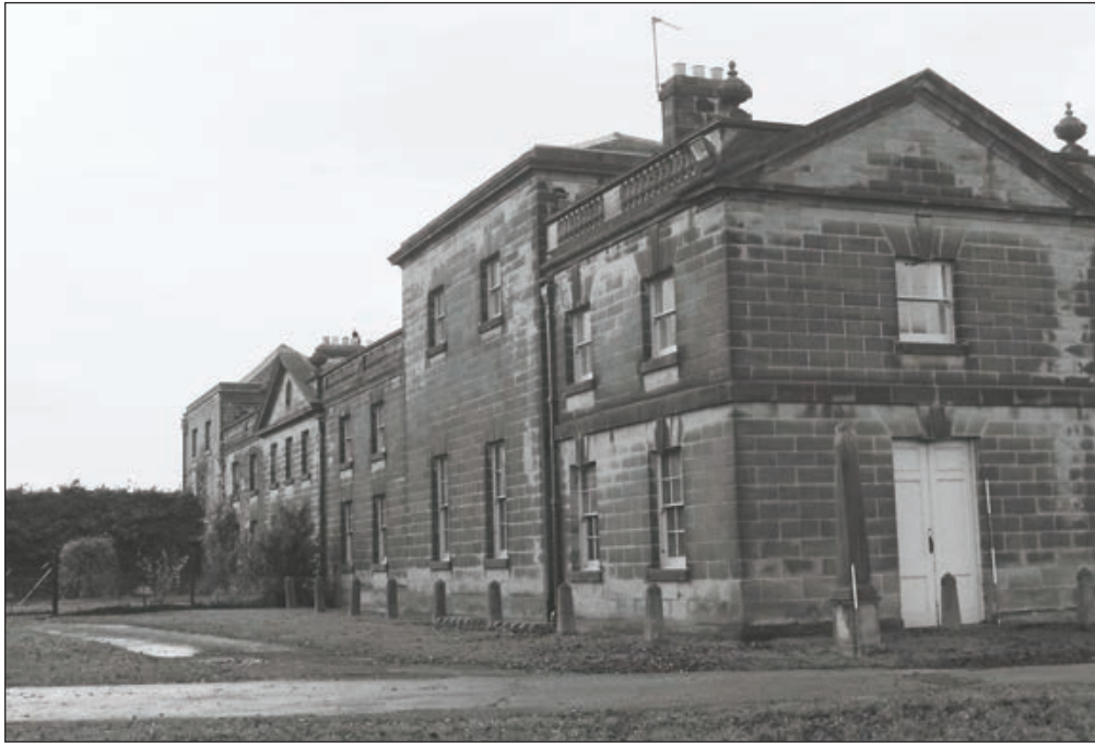
Plate 3 : General view of the east elevation of the East Range and northeast corner of the North Range from the northeast (Film 11.24)
