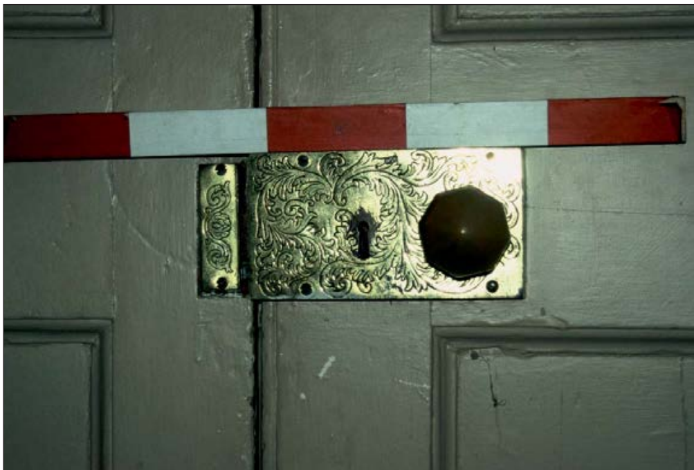
Plate 419: Detail of decorative etched box lock on doorway in south wall of G33, South Range (Film C.S. 20.)
