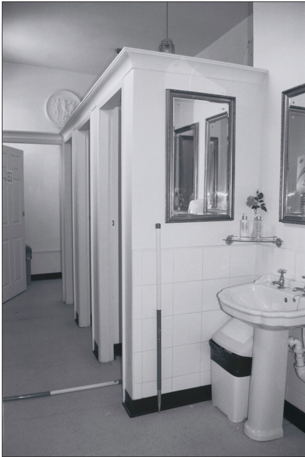
Plate 446: General view of G39, South Range (Film 24.26)
