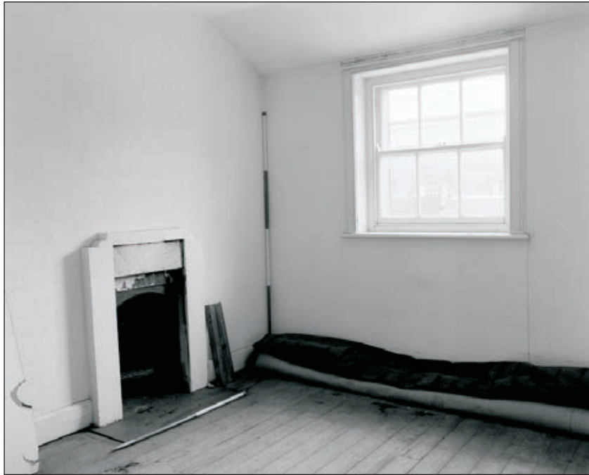
Plate 240: General view of room F17, West Side of the North Range (Film 34.01)
