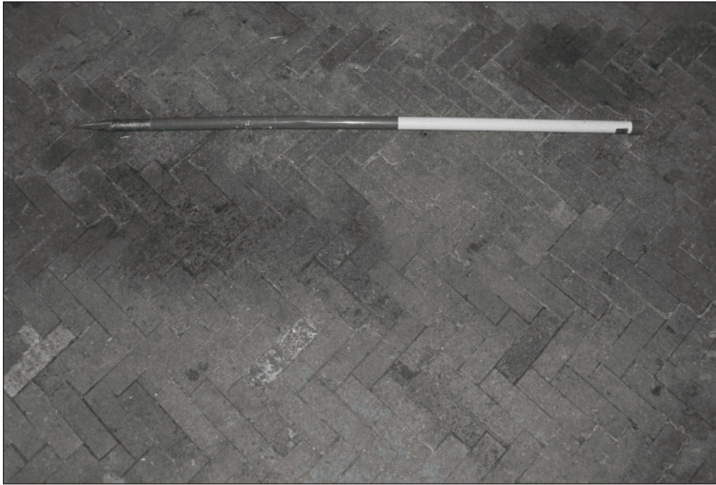
Plate 52: Detail of original herringbone brick floor of the southern half of room G2, East Side of the North Range (Film 14.14)
