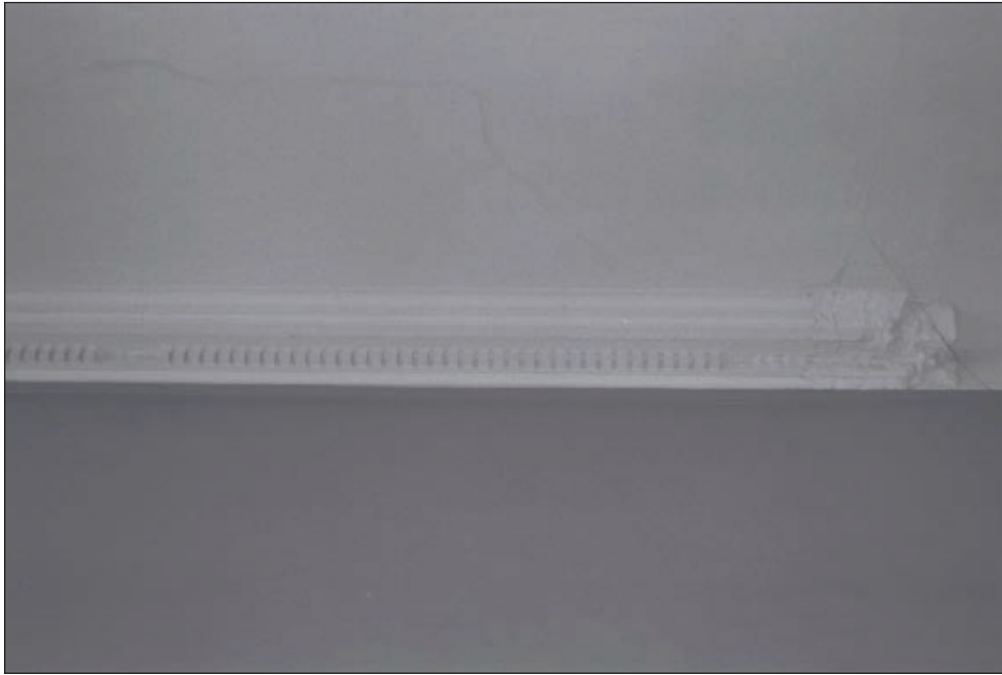
Plate 407: Detail of original cornice, east wall of G30, South Range (Film 24.15)
