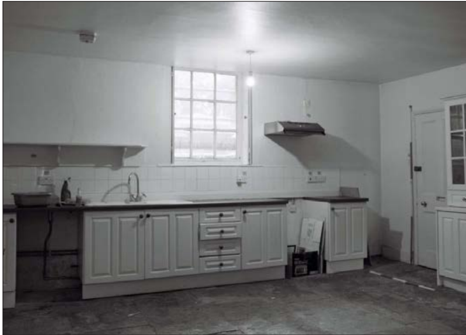
Plate 511: General view of G51, South Range - Agent's House (Film 59.05)
