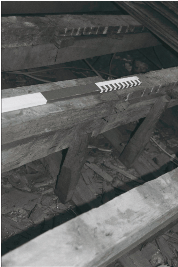
Plate 534: Detail of exposed timber floor and ceiling construction, F35, South Range - Agent's House - OB. 76 (Film 66.12)
