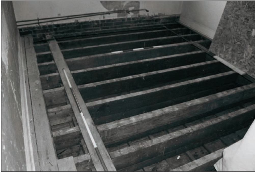
Plate 252: View of exposed timber and RSJ floor structure of room F20, West Side of the North Range - OB. 40 (Film 53.35)
