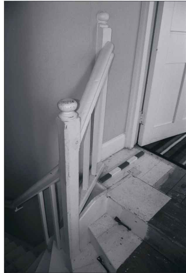
Plate 590: Detail of truncated and moved newel post at top of staircase, F42, East Range (Film 22.34)
