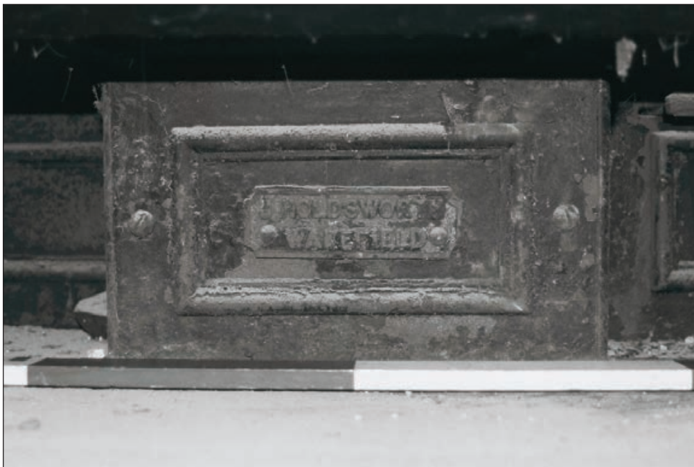
Plate 100: Detail of 'J. Holdsworth, Wakefield' name plate on corner fireplace, room G9, Central Entranceway of the North Range (Film 52.17)
