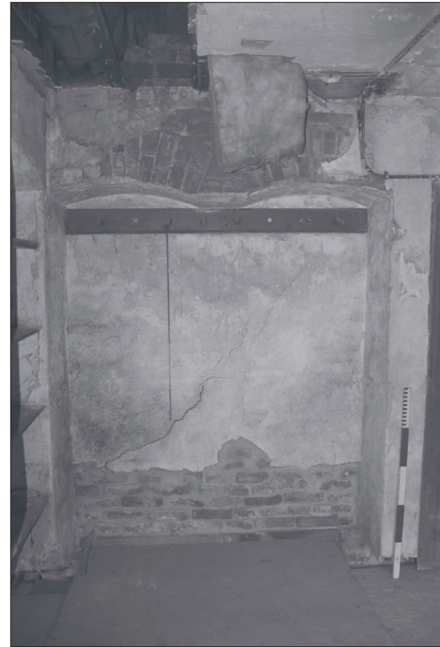
Plate 213: View of the north wall of F12, Central Entranceway of the North Range, showing blocked opening (Film 74.12)
