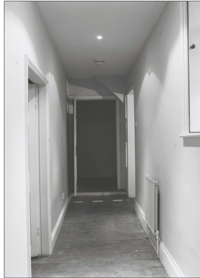
Plate 498: General view of G50, South Range, Agent's House (Film 59.07)
