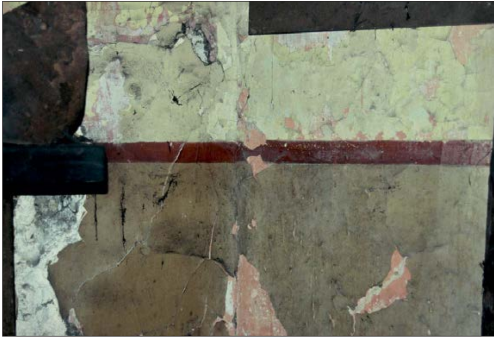
Plate 101: Detail of paint scheme, north wall of room G9, Central Entranceway of the North Range (Film C.S. 25.)
