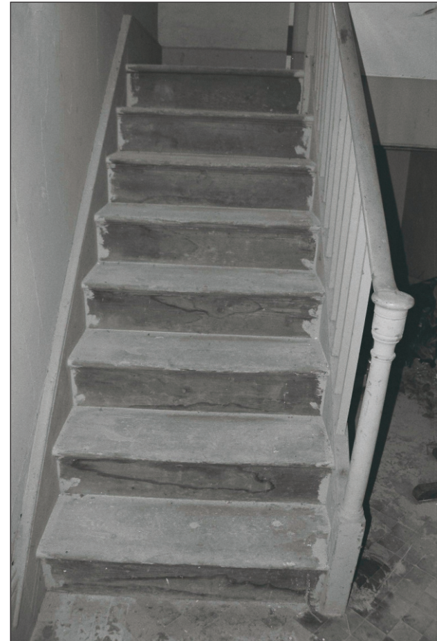
Plate 427: General view of staircase, G35, South Range, showing timber treads (Film 70.15)
