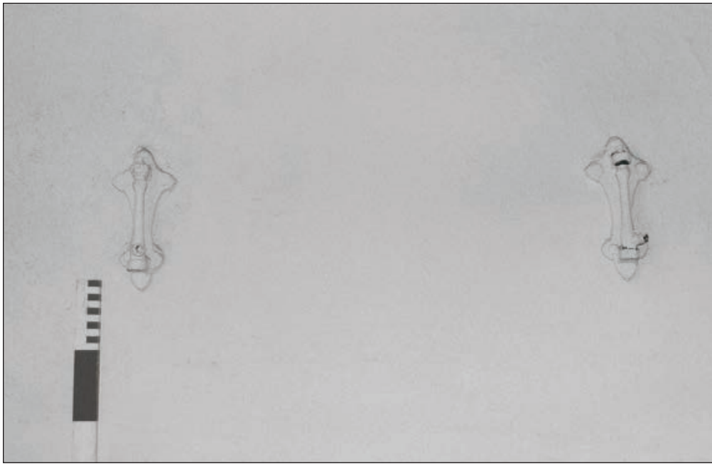
Plate 66: Detail of original Musgrave folding brackets, east wall of room G3, 'Wash Room', East Side of the North Range (Film 15.09)
