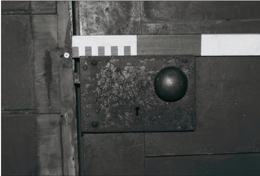
Plate 148: Detail of box lock on door between F3 and F4, East Side of the North Range (Film 16.09)
