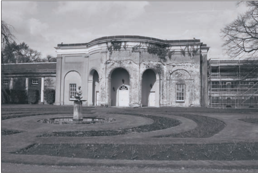
Plate 344: View of the south elevation of the South Range after the removal of vegetation, exposing the fabric of the building - OB. 32 (Film 51.16)
