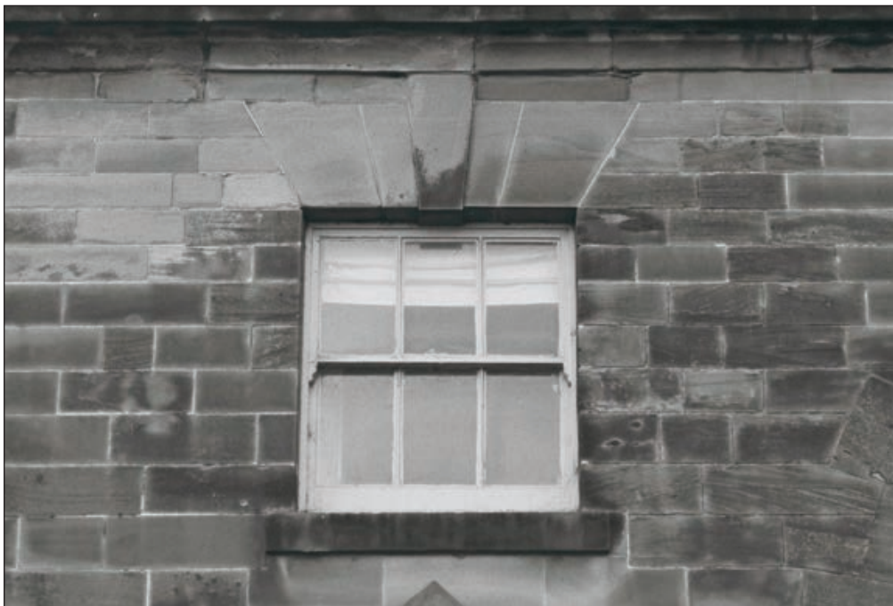
Plate 15: Detail of first floor window, north elevation of North Range (Film 11.06)
