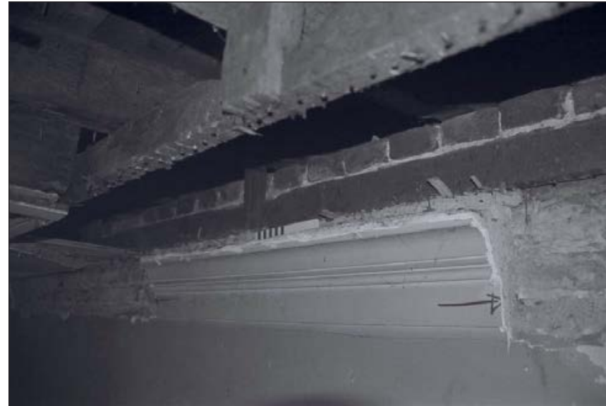
Plate 441: Detail of cornice and ceiling structure, F30/31, South Range - OB. 109 (Film 74.28)
