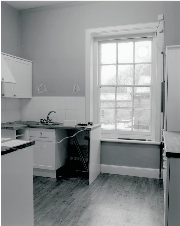
Plate 604: General view of F51, East Range (Film 27.08)
