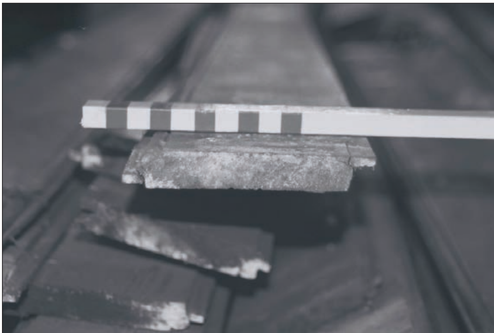
Plate 89: Detail of match boarding of room G4, 'Tack Room', Central Entranceway of the North Range - OB. 71 (Film 56.05)
