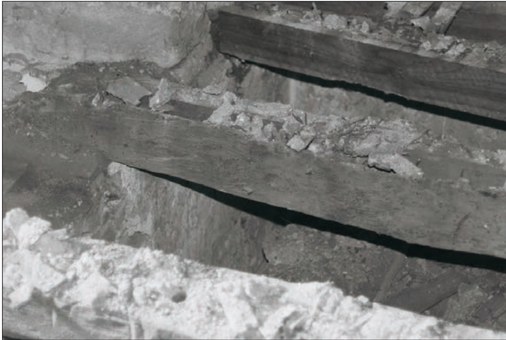
Plate 218: Detail of exposed timber floor joists, room F13, Central Entranceway of the North Range, after removal of limeash, showing construction marks (Film 69.30)
