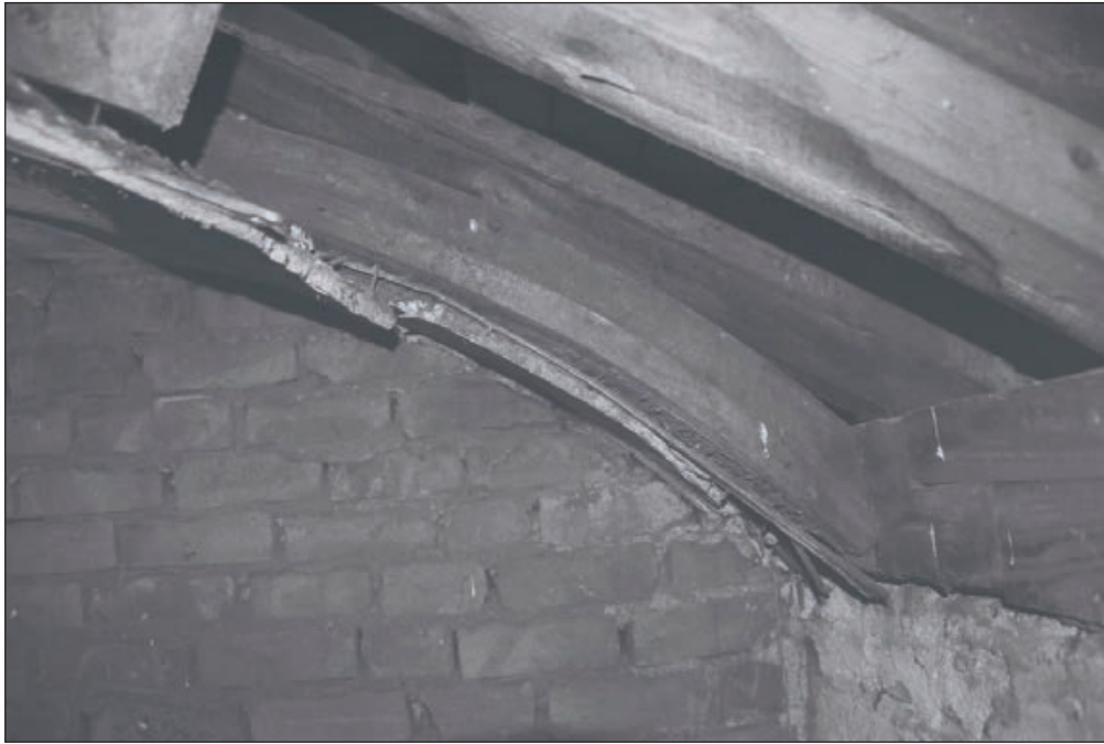
Plate 454: Detail of original ceiling construction, G42, South Range - OB. 97 (Film 74.31)
