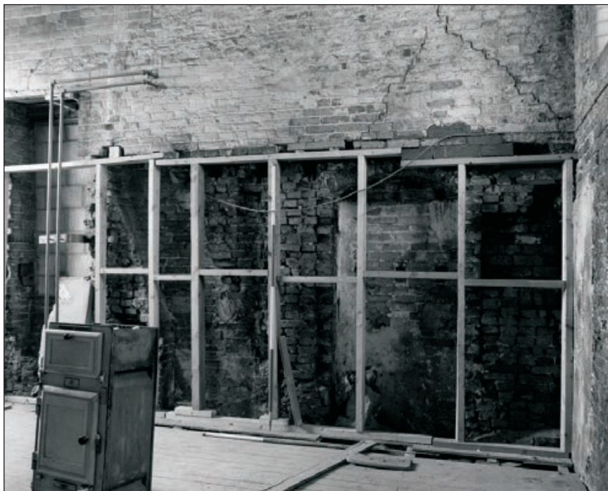
Plate 316: General view of earlier south wall of F27, West Range, showing blocked door and flue (Film 36.06)
