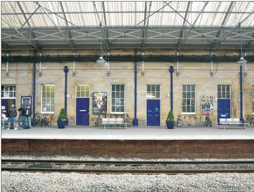
Plate 55: General view of west elevation of the South Wing.
