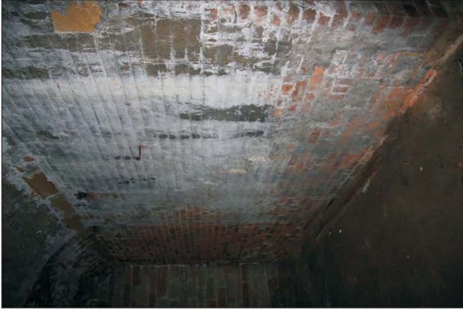
Plate 37: Detail of scar from former staircase in basement, looking northwest.
