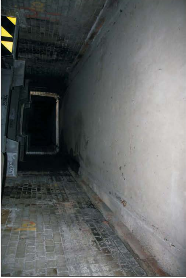
Plate 38: General view of disused goods subway, looking west.
