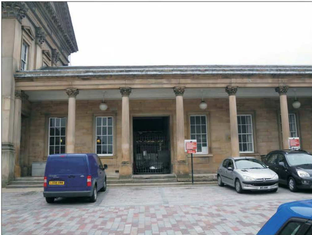
Plate 23: General view of colonnade on eastern elevation of the North Wing.
