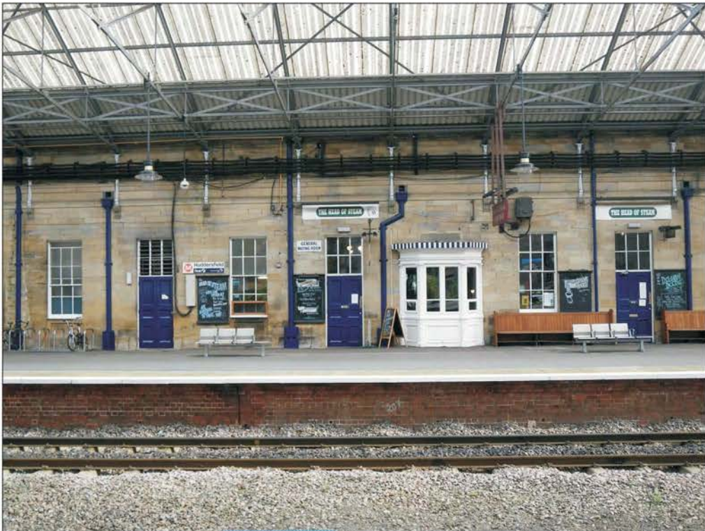
Plate 54: General view of the west elevation of the southern pavilion.
