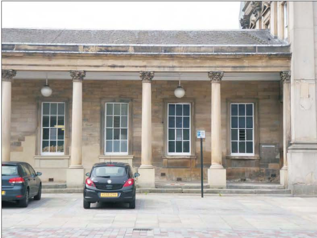
Plate 48: General view of eastern elevation of South Wing.
