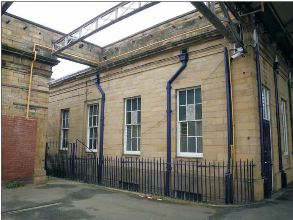
Plate 26: General view of the northern elevation of the northern pavilion.
