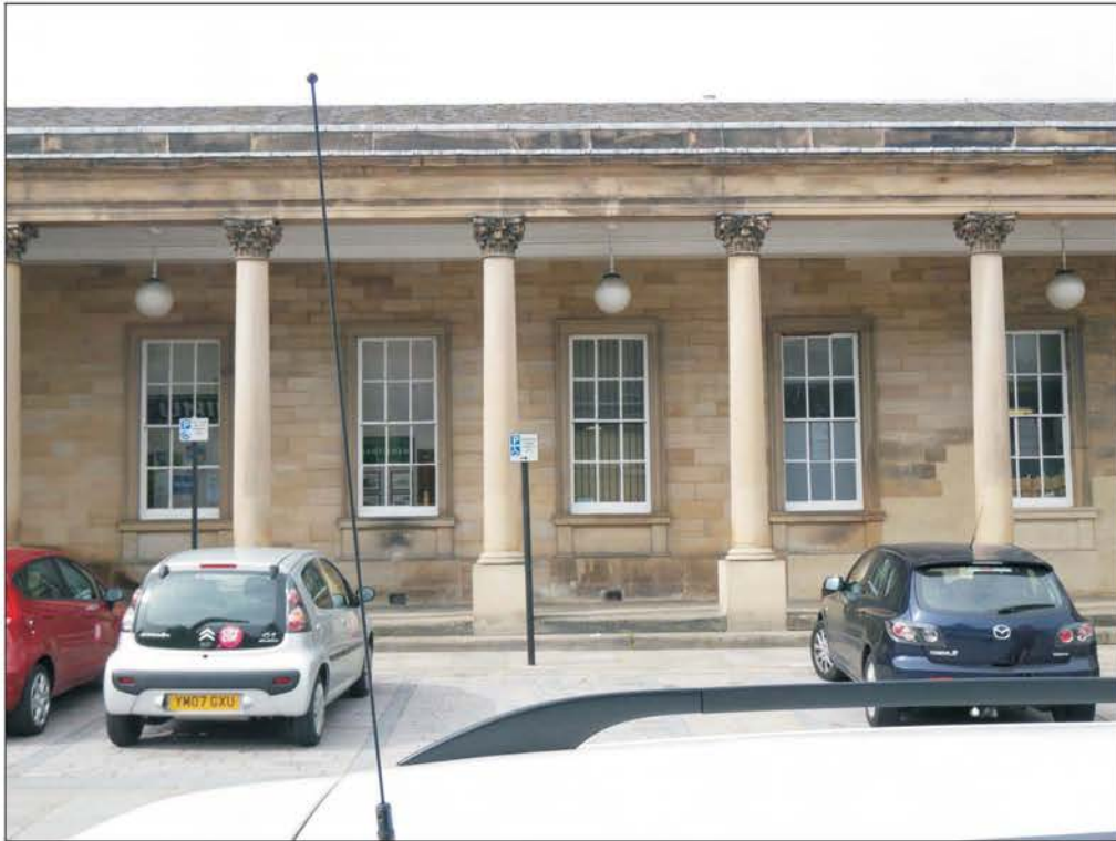
Plate 49: General view of eastern elevation of South Wing.
