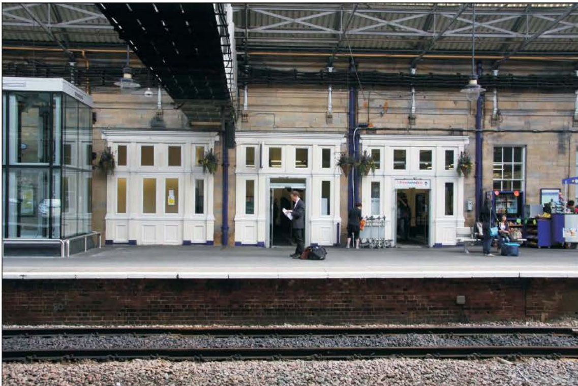
Plate 8: General view of west elevation of centre of Central Block.
