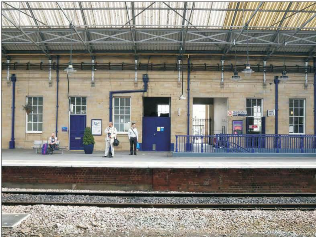
Plate 28: General view of the western elevation of the North Wing.
