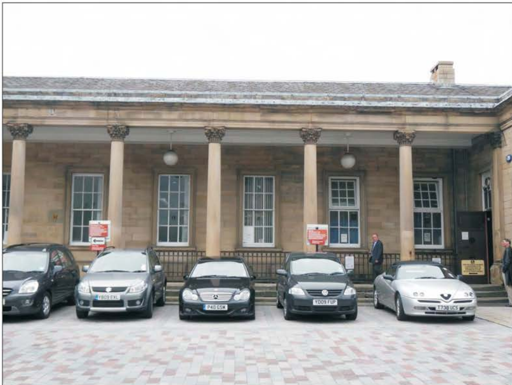
Plate 24: General view of colonnade on eastern elevation of the North Wing.
