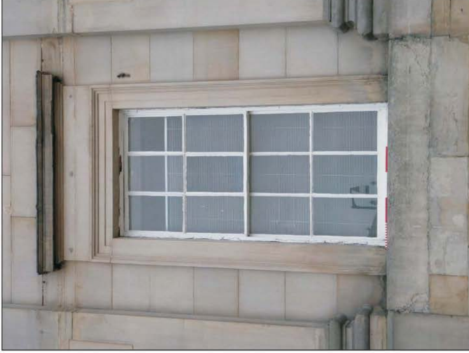
Plate 4: Detail of ground floor window in east elevation of Central Block.
