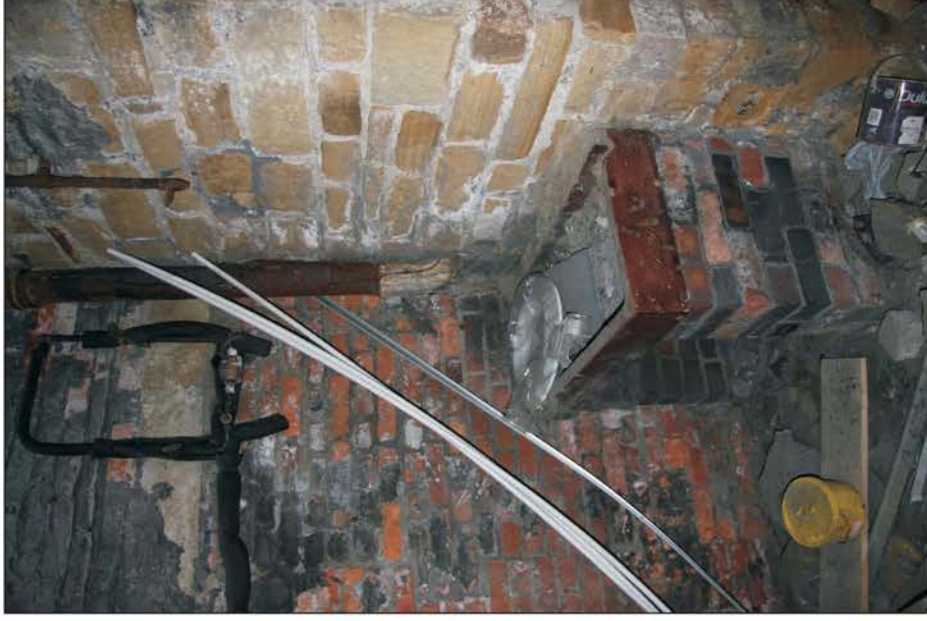
Plate 36: Detail of ceramic basin in basement, looking northeast.
