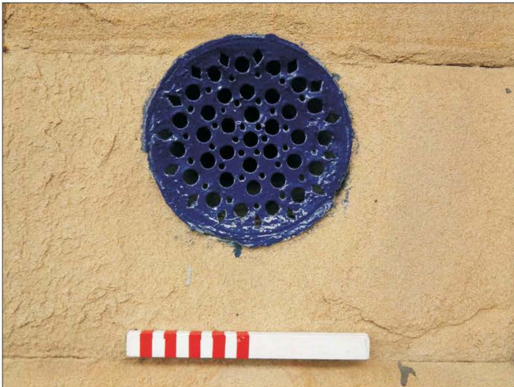
Plate 32: Detail of circular vent in west elevation of pavilion.
