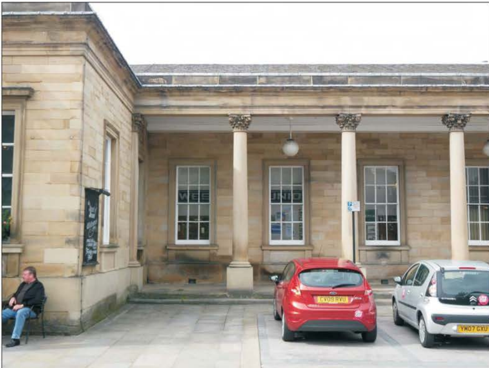
Plate 50: General view of eastern elevation of South Wing.
