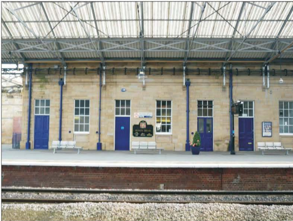
Plate 27: General view of western elevation of the northern pavilion.
