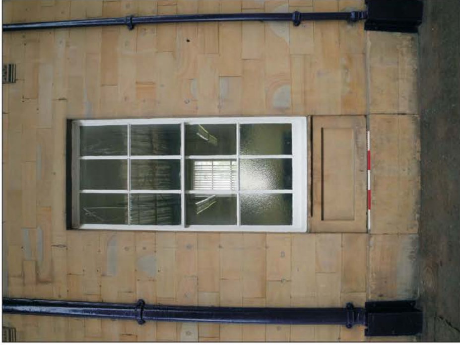
Plate 10: Detail of inserted window in west elevation.
