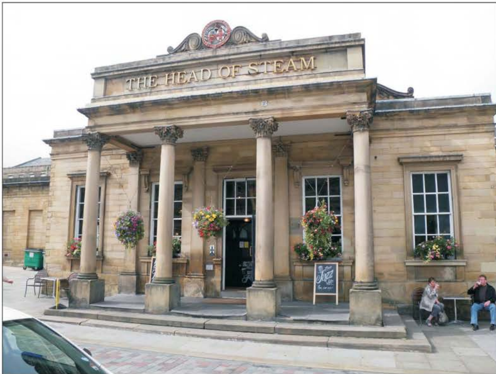
Plate 51: General view of east elevation of the southern pavilion.
