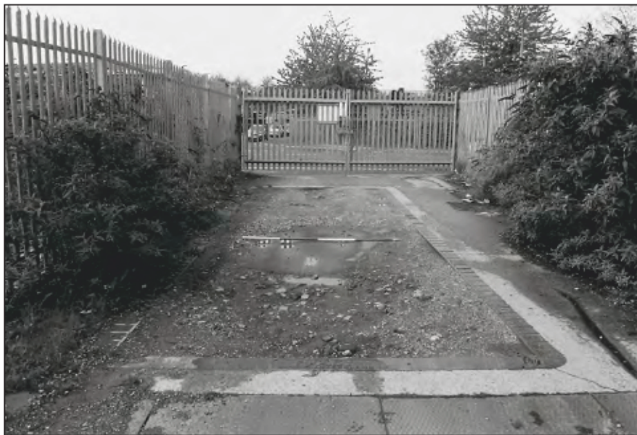
Plate 4: Detail of eastern Weedon Street site entrance with weighbridge. (film 6.35)
