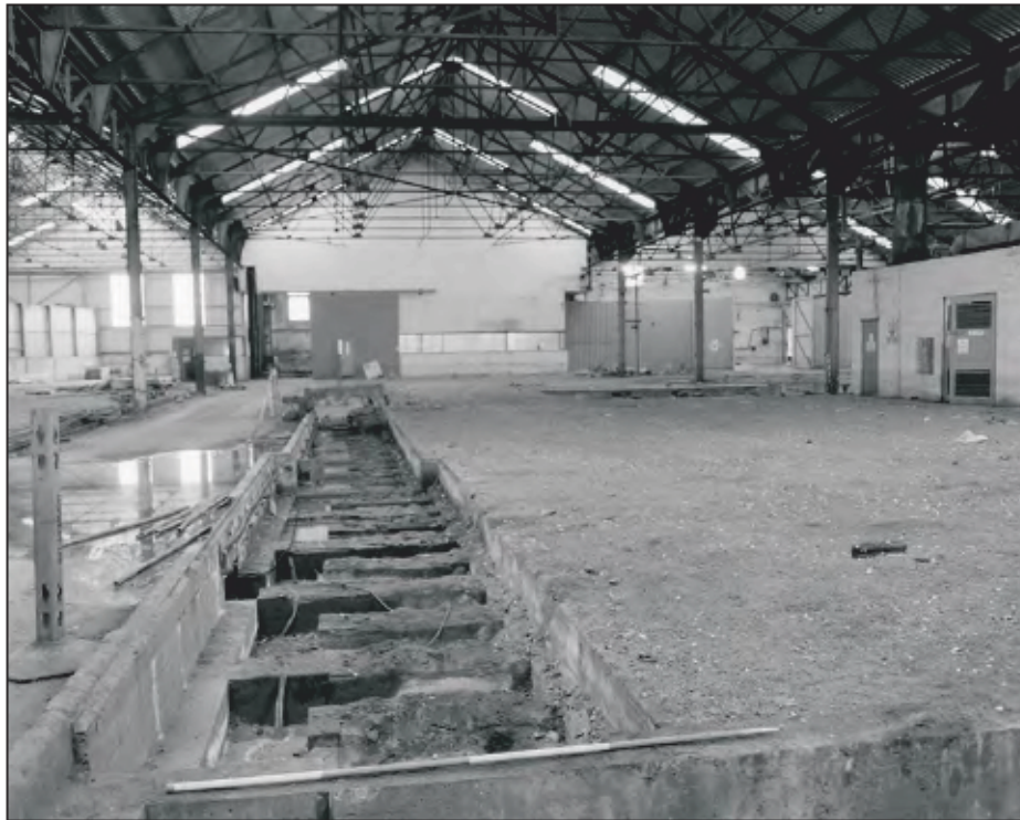
Plate 59: General view of foundation trench for run-out rolls from the final stand of the 10.5" Double Duo Mill. (film 23.06)
