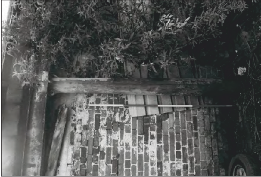
Plate 79: Detail of cast iron column in west elevation of Building 17. (film 6.20)
