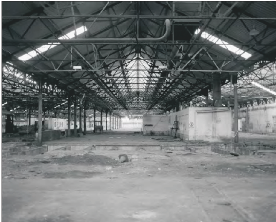
Plate 35: General view looking south down the second range of Building 11. (film 21.04)
