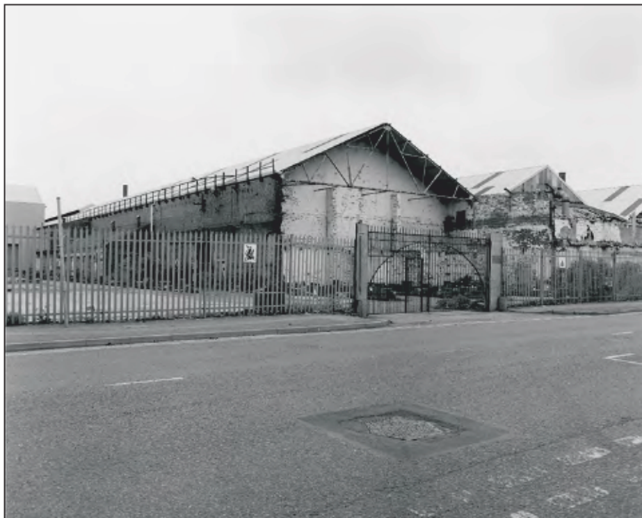
Plate 28: General view of Building 11 from the southwest, showing demolished southern ranges. (film 14.07)
