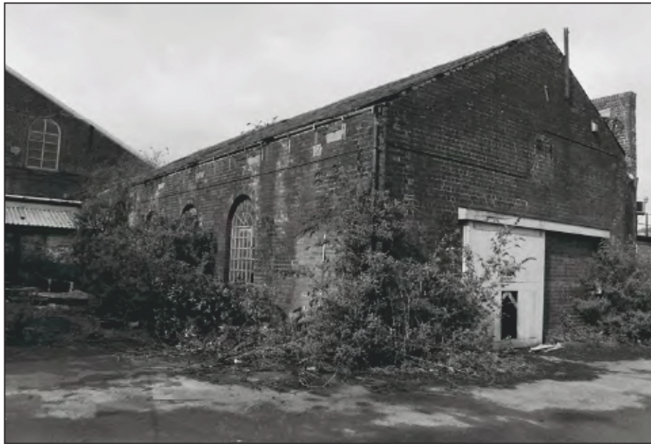
Plate 69: General view of Building 13, looking from the northeast. (film 6.02)
