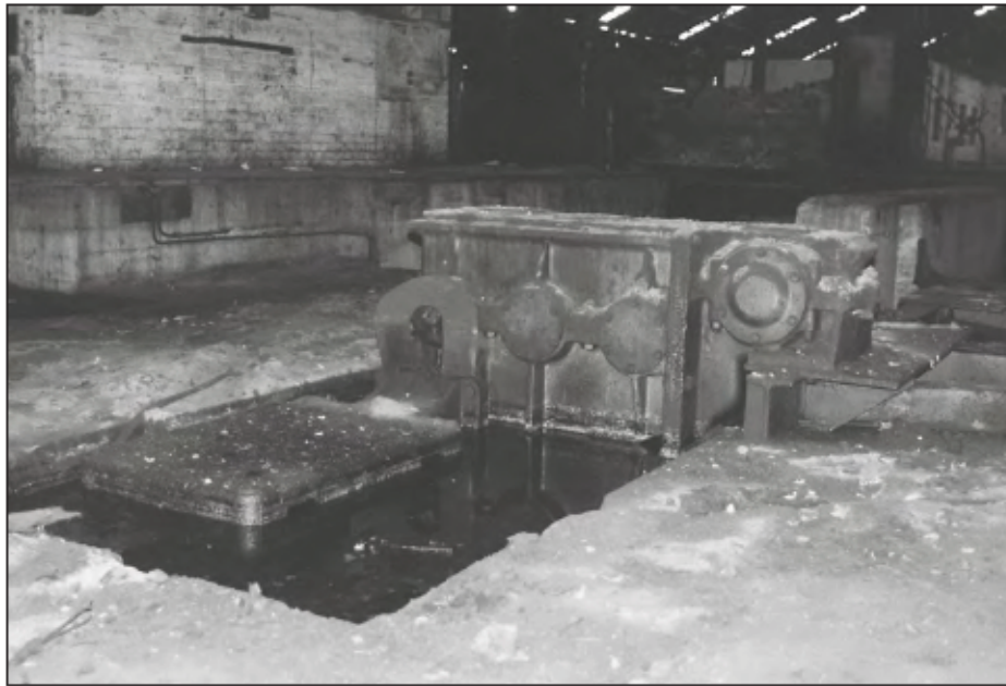
Plate 53: Detail of motor base and gear box from the run-out rolls of the second intermediary stand of the 18" Rolling Mills. (11.10)
