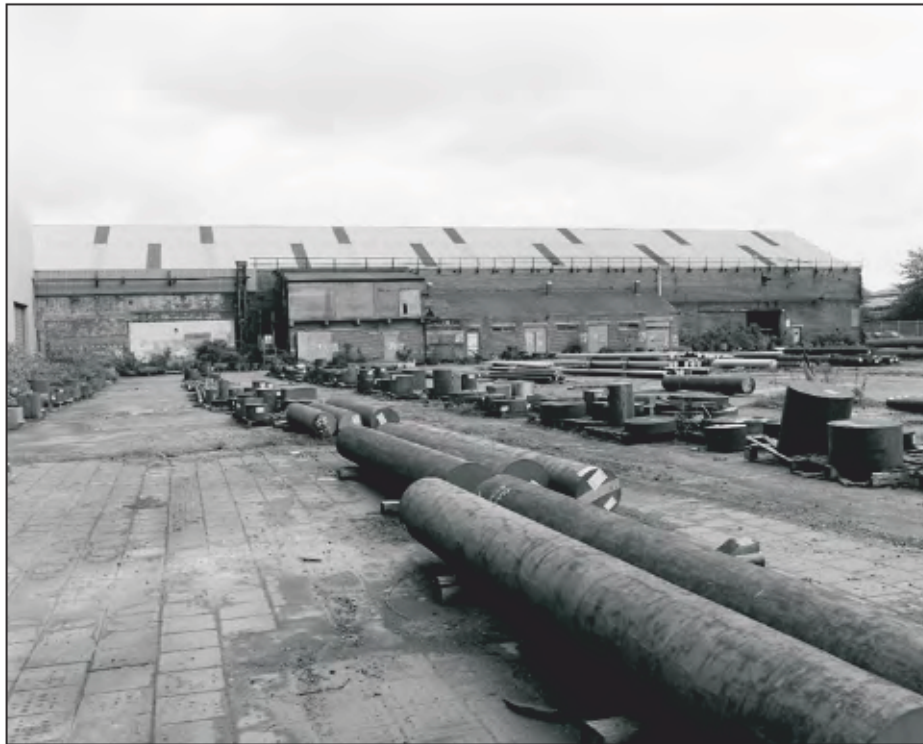
Plate 29: General view of western elevation of Building 11. (film 24.05)
