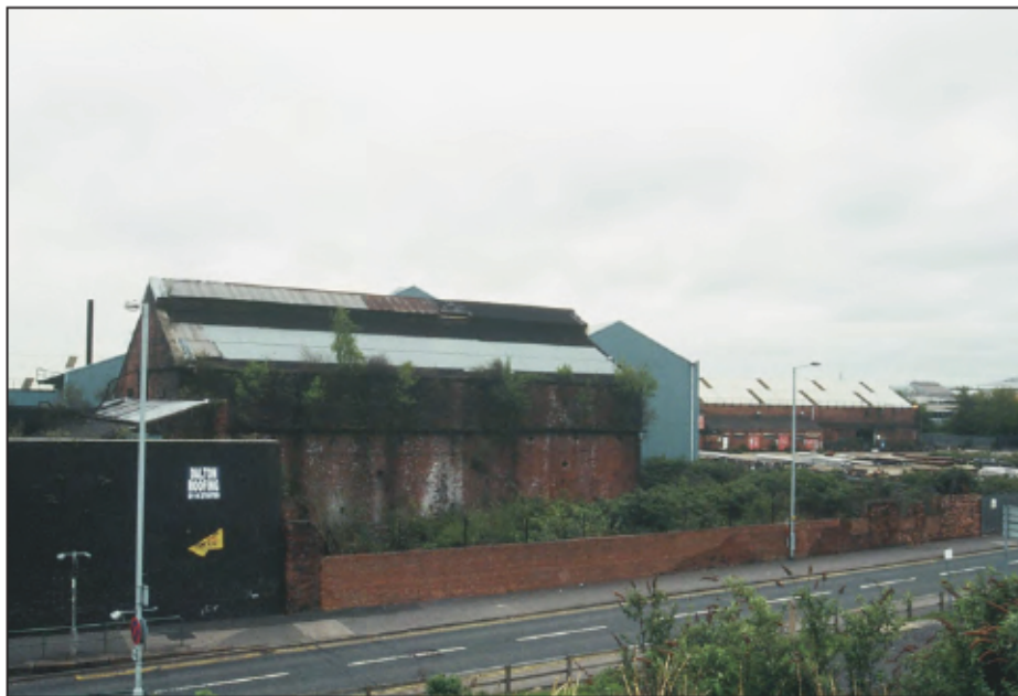
Plate 8: General view of Building 10 showing the demolished remains of the former boiler house between Vulcan Street and the turbine hall. (colour slide 18)
