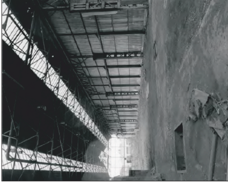
Plate 84: General view of interior of Building 18, looking east. (film 4.07)
