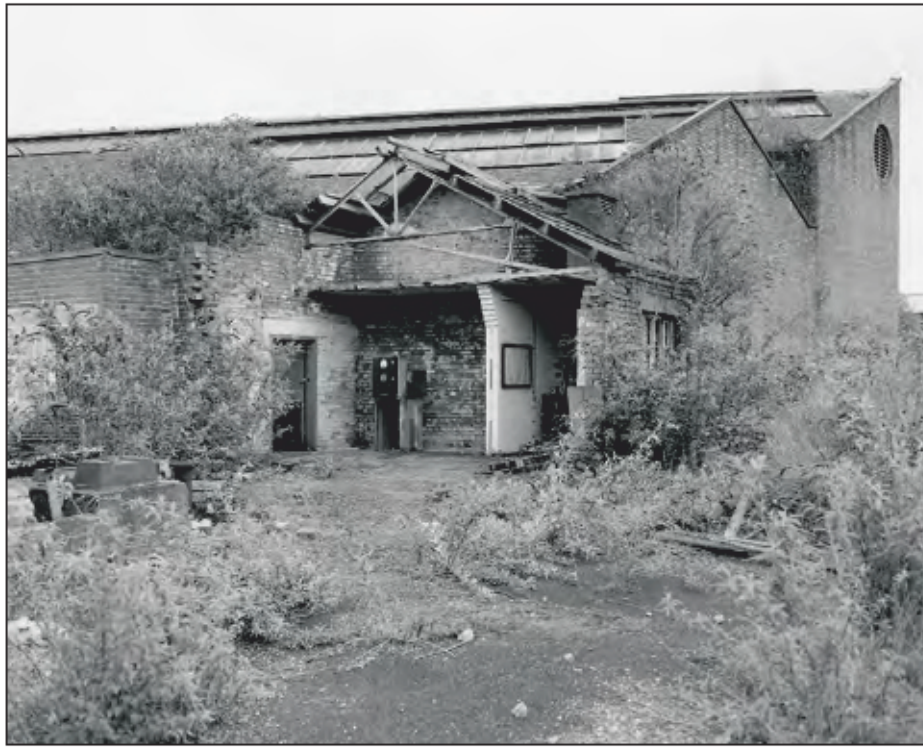
Plate 87: General view of Building 19, looking south. (film 15.03)
