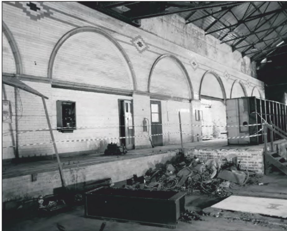
Plate 21: General view showing blocked arches in east wall of Building 10. (film 17.09)
