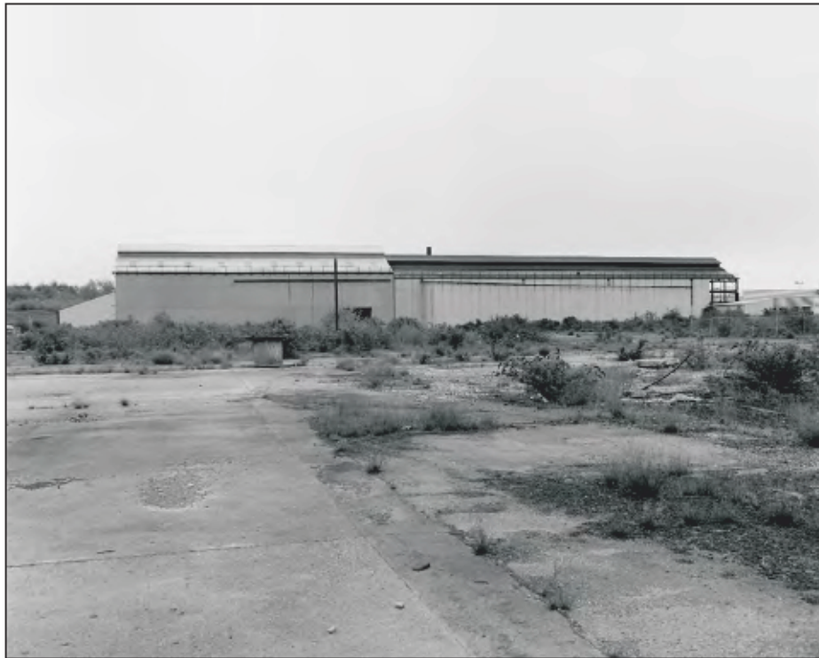
Plate 81: General view of Building 18, looking north. (film 15.05)
