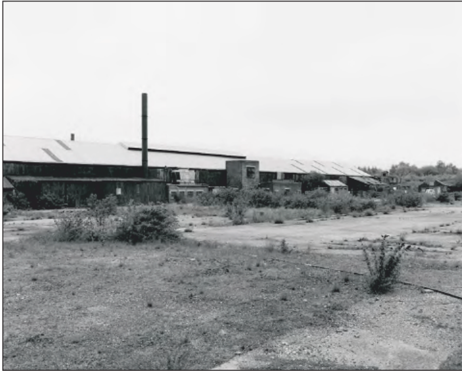
Plate 33: General view of eastern elevation of Building 11. (film 15.01)
