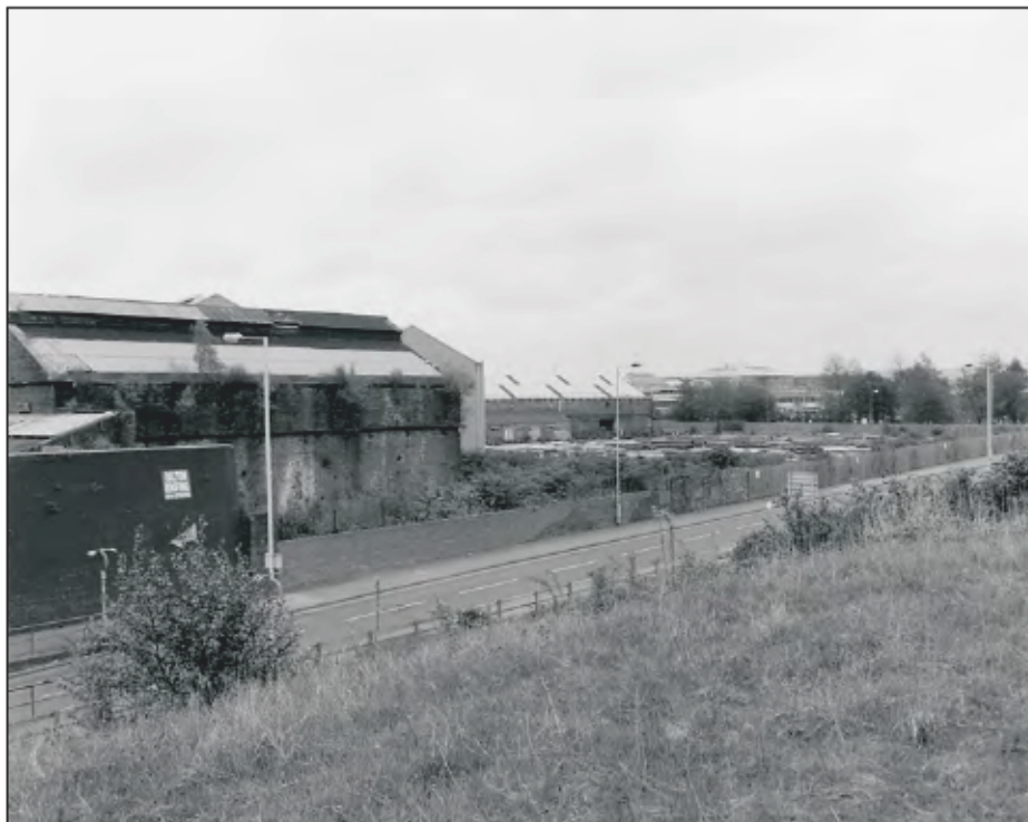
Plate 2: General view across the Works from the northwest. (film 14.05)
