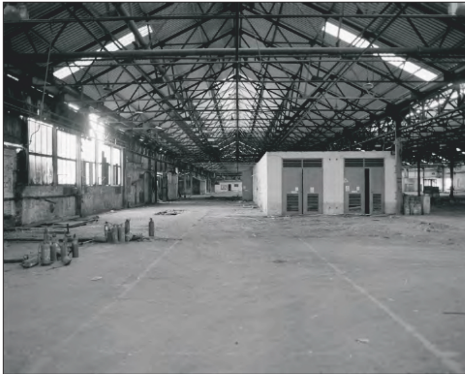
Plate 37: General view looking south down the fourth range of Building 11. (film 21.08)
