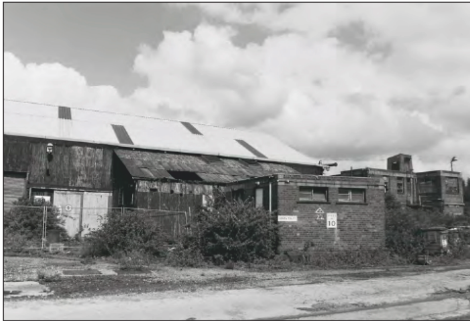
Plate 77: General view of Building 16, looking northwest. (film 8.20)
