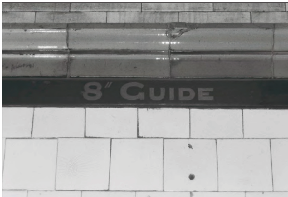
Plate 22: Detail of name plate above blocked arch in Building 10. (film 26.10)
