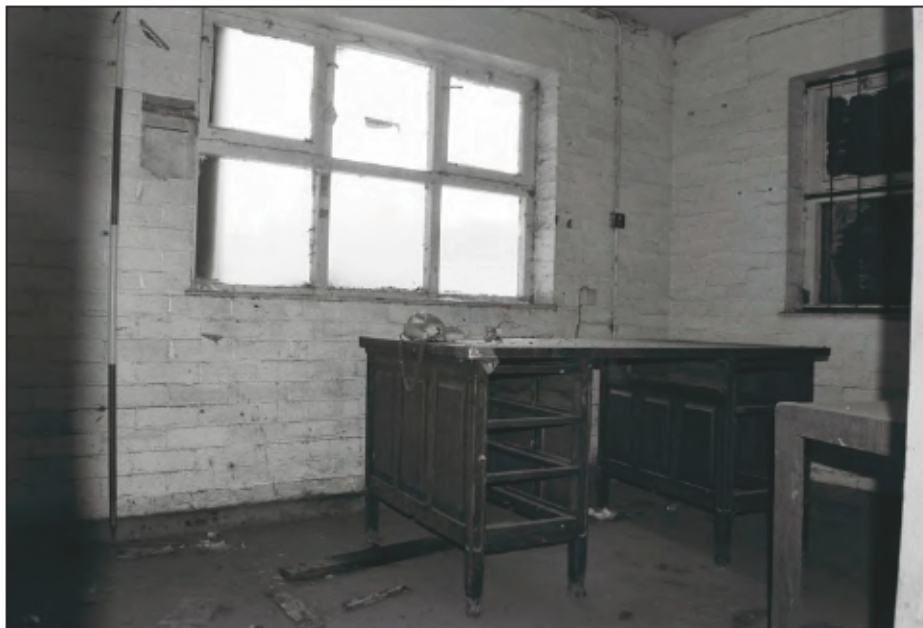
Plate 86: General view of interior of office in Building 18. (film 5.11)
