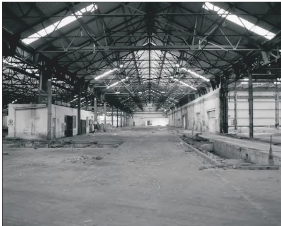
Plate 34: General view looking south down the first range of Building 11. (film 21.02)
