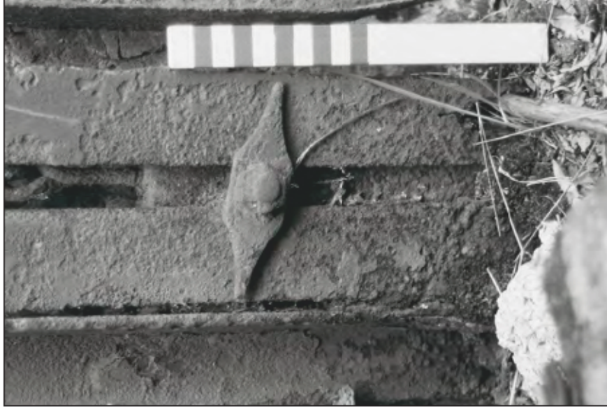
Plate 14: Detail of former depth gauge on water tower of Building 10. (film 27.08)
