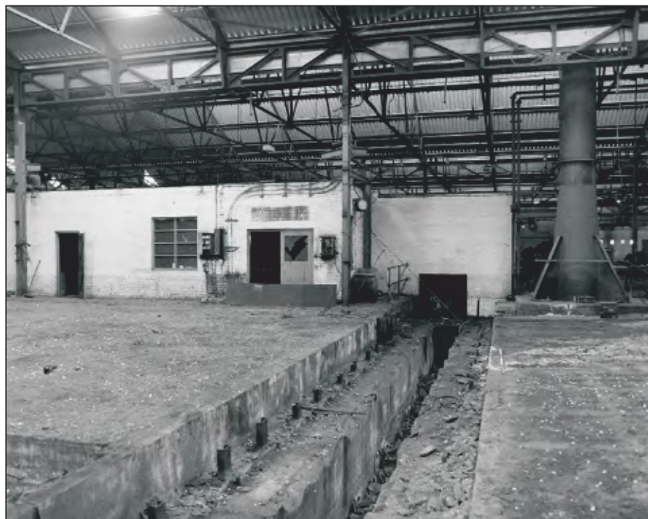
Plate 58: General view of foundation trench for the 6 stand mill arrangement of the 10.5" Double Duo Mill. (film 23.04)
