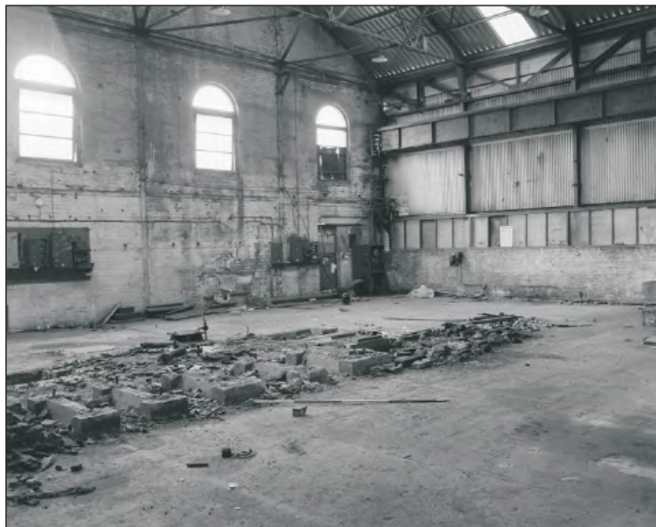
Plate 38: General view of turning workshop in northwest corner of Building 11. (film 20.09)
