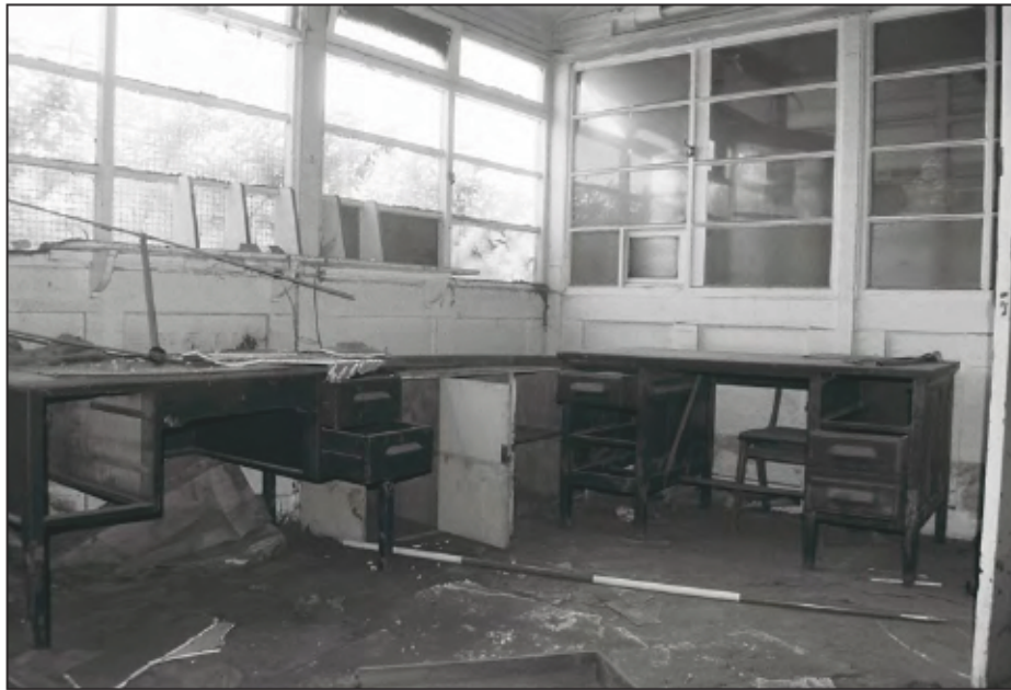
Plate 43: General view within office situated on the east elevation of Building 11. (film 13.29)
