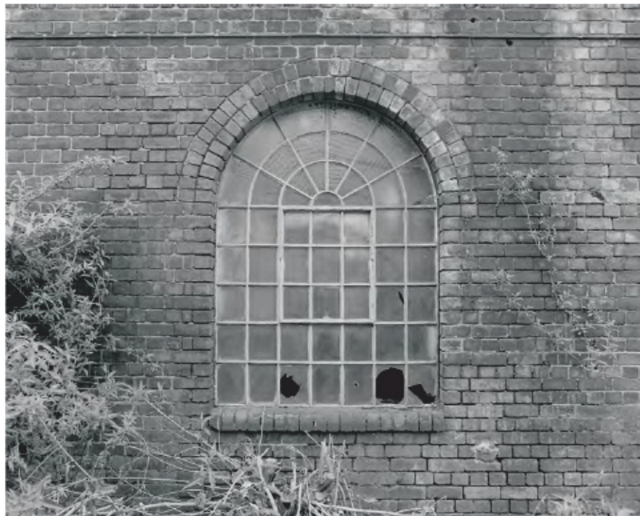
Plate 70: Detail of window in the east elevation of Building 13. (film 16.08)
