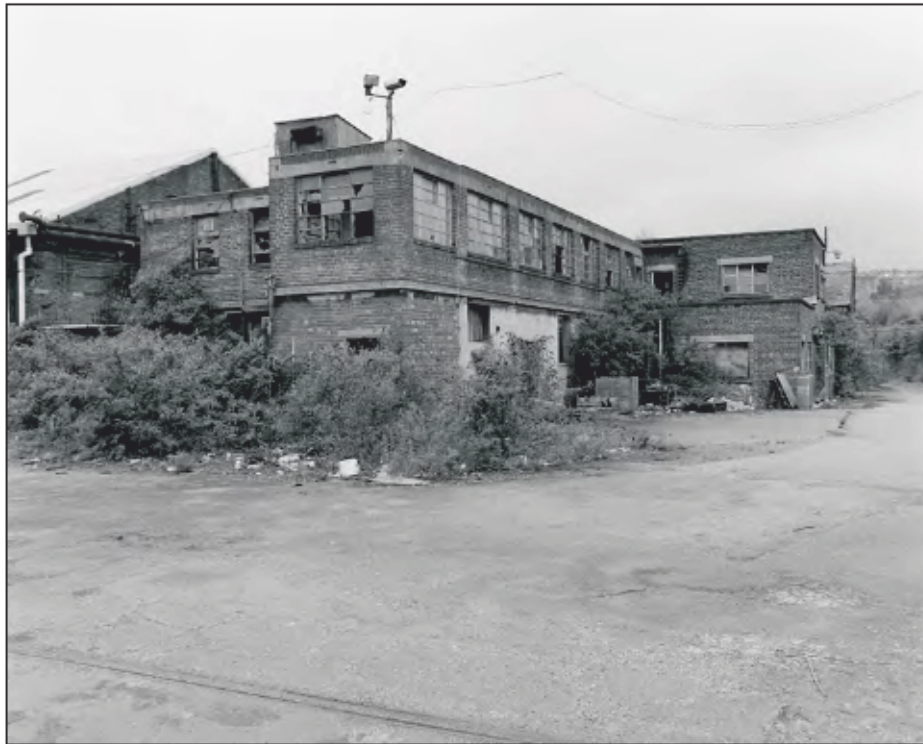
Plate 75: General view of Building 15, looking southwest. (film 16.01)
