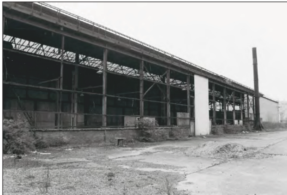
Plate 82: General view of Building 18, looking southwest. (film 4.10)
