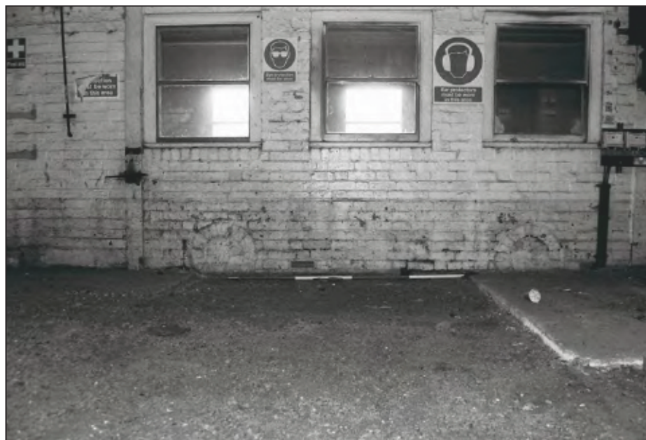
Plate 40: Detail of blocked circular openings in north wall of the third range of Building 11. (film 9.01)
