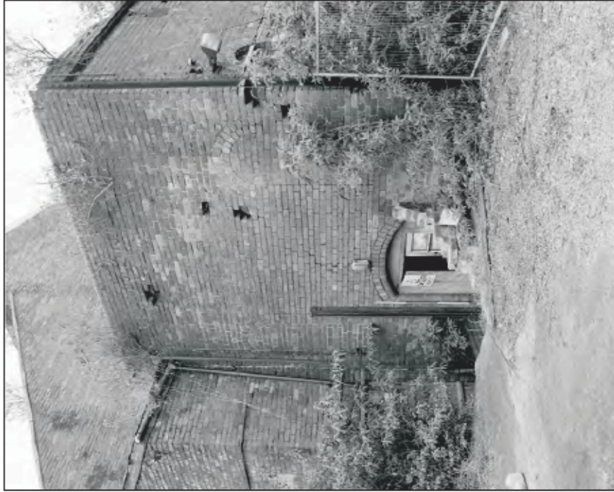
Plate 13: General view of water tower, noting integrated iron framework. (film 17.07)
