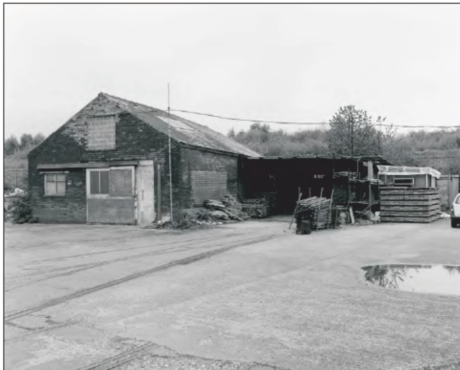
Plate 78: General view of Building 17, looking north. (film 16.03)
