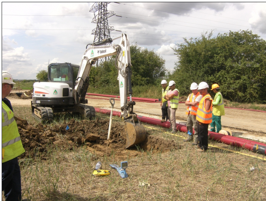
Plate 6: Opening of Trench 31, view from the south-east
