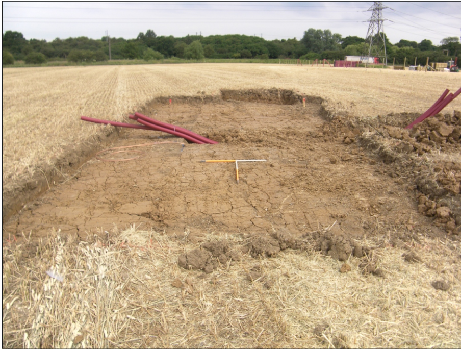
Plate 1: View of Foundation Trench 1
