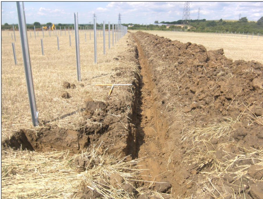
Plate 4: View of Trench 17 from the east
