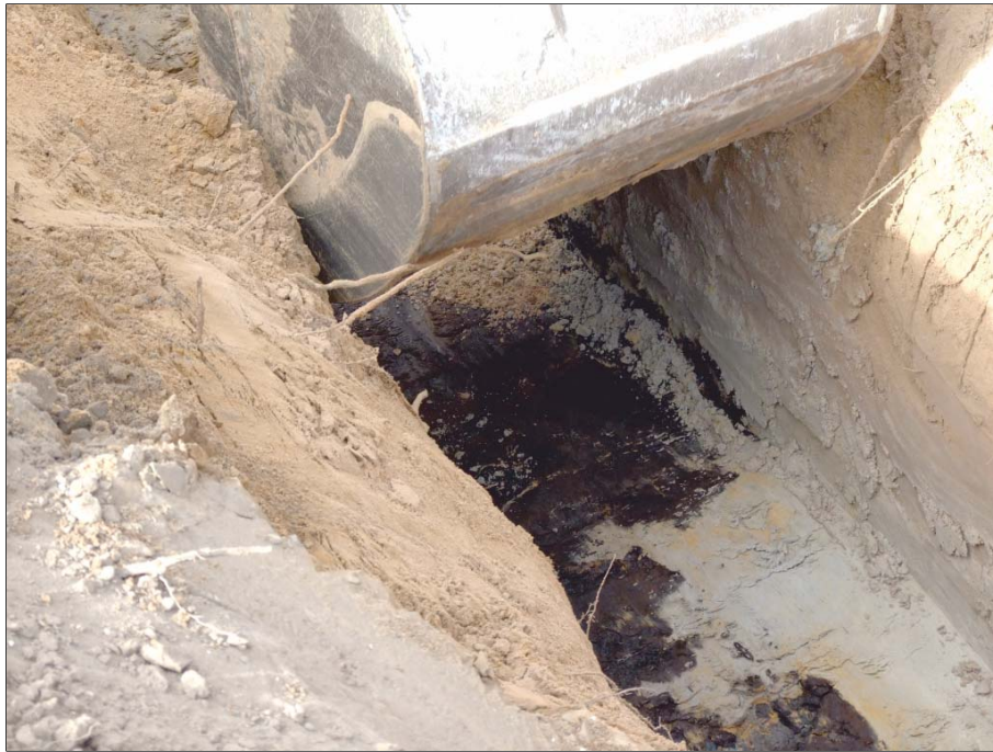
Plate 7: Working shot machining down into peat layer 1406
