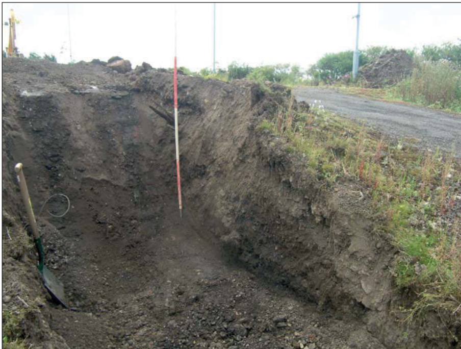
Plate 2: General shot of Trench 2
