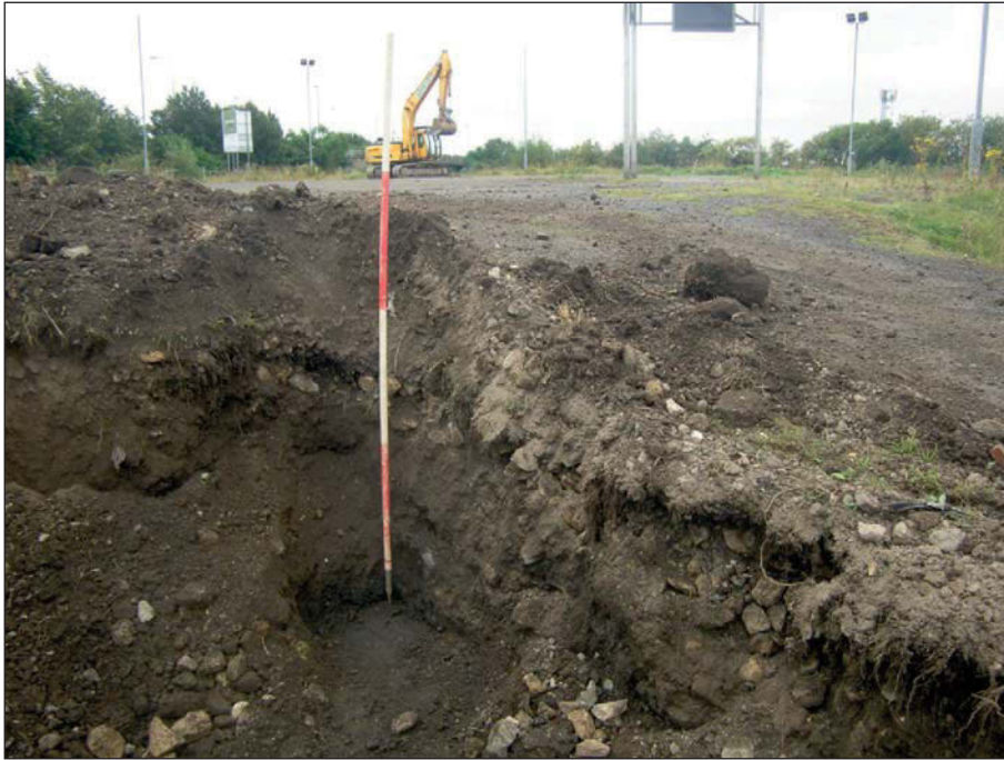
Plate 1: General shot of Trench 1
