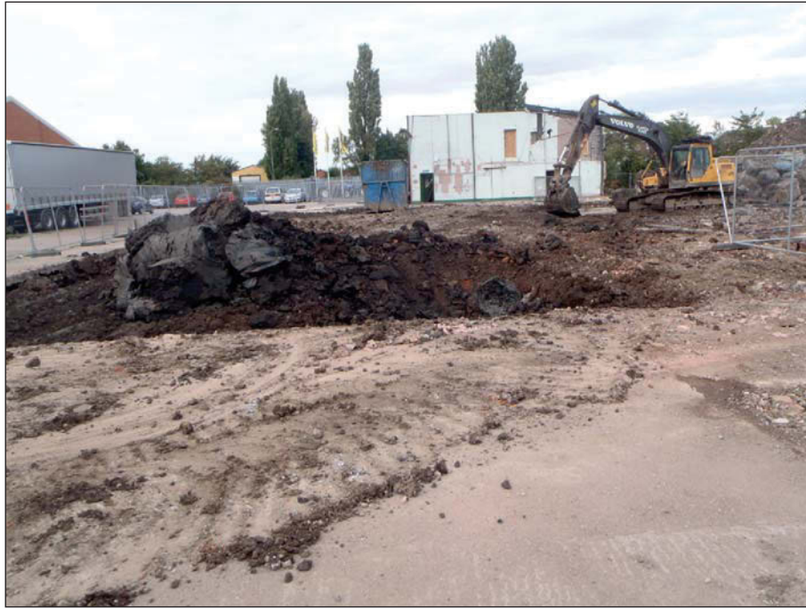
Plate 5: General shot of Trench 5 during excavation
