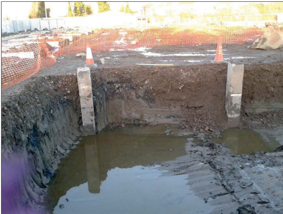
Plate 8: General shot of Trench 7, access road strip
