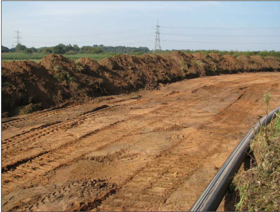
Plate 5: Topsoil strip of Area C
