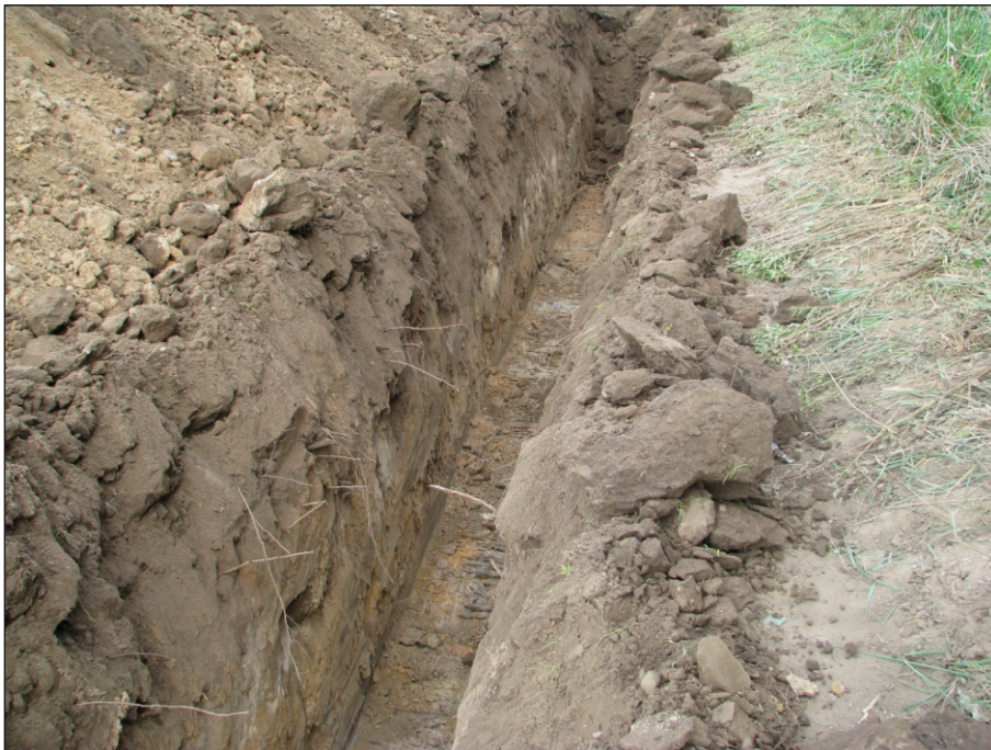
Plate 4: Trenching in Area B
