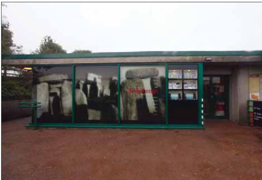
Plate 46: Shop north elevation
