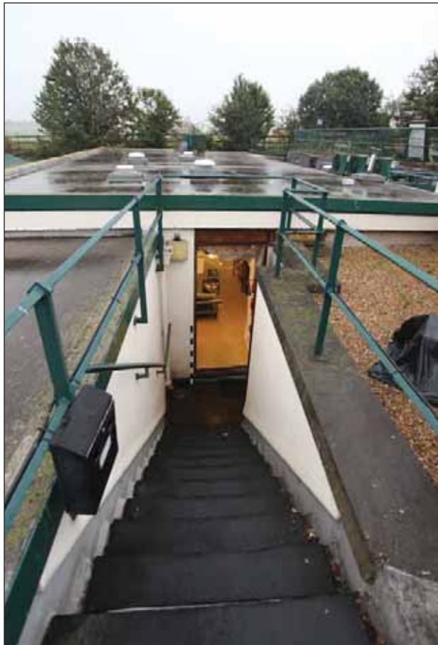
Plate 35: Entrance to kitchen and server areas viewed from the west
