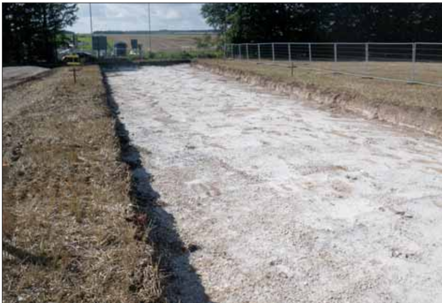
Plate 10: Excavation of road realignment, north of Airman's Corner
