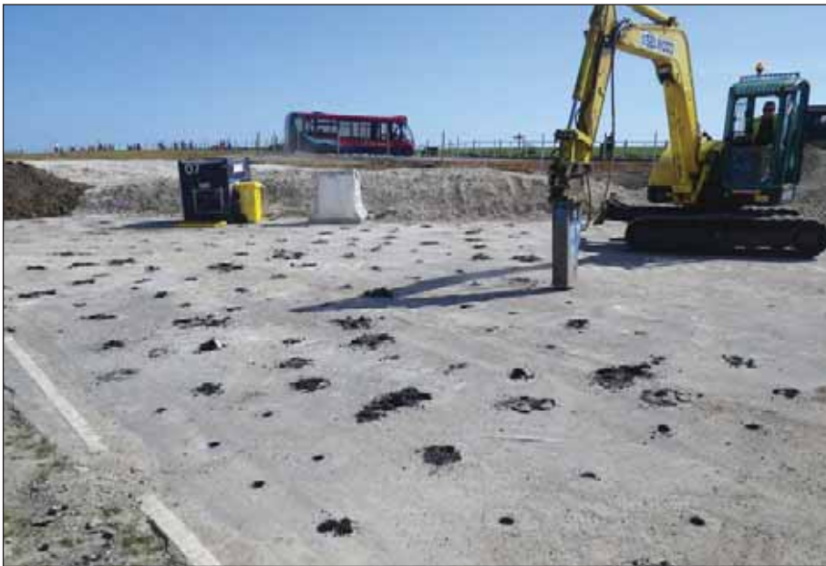
Plate 26: Puncturing of former car park surface, viewed from the west.
