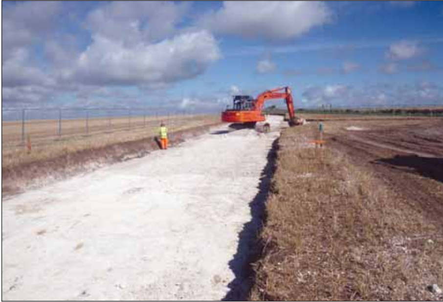
Plate 11: Further excavation of road realignment, north of Airman's Corner
