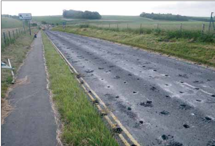
Plate 17: Puncturing the tarmac along the A344 following its closure
