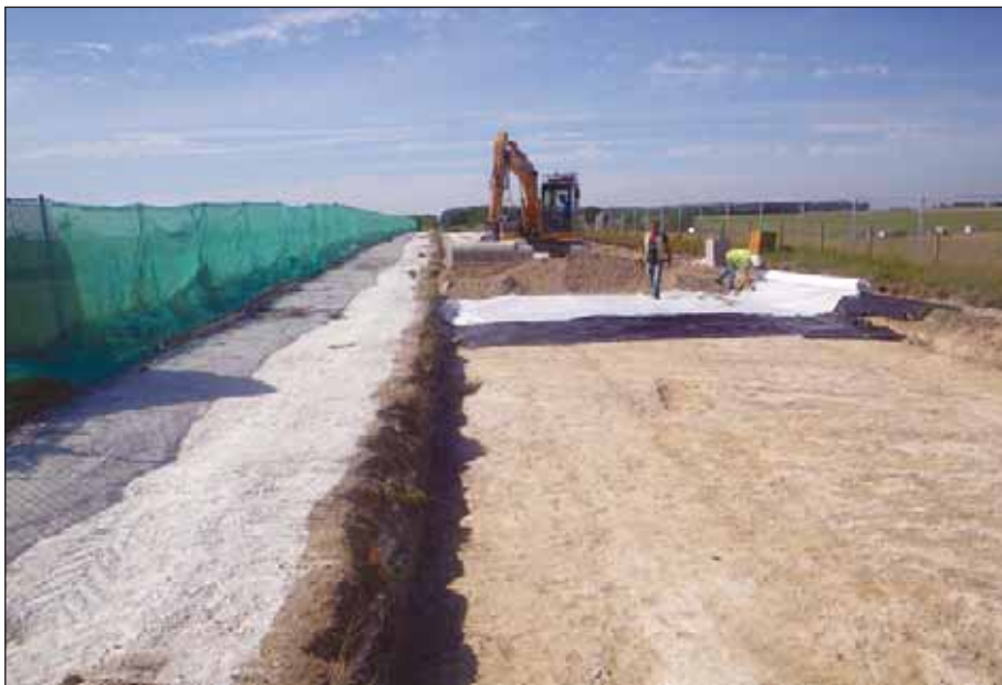
Plate 18: Laying of geotextile over Phase 3 area
