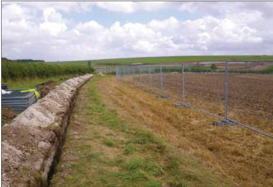
Plate 13: Excavation of drainage trenches during Phase 2 works
