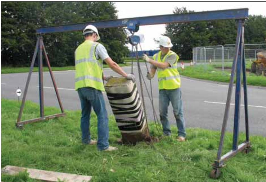
Plate 8: Lifting of the milestone at Airman's Corner
