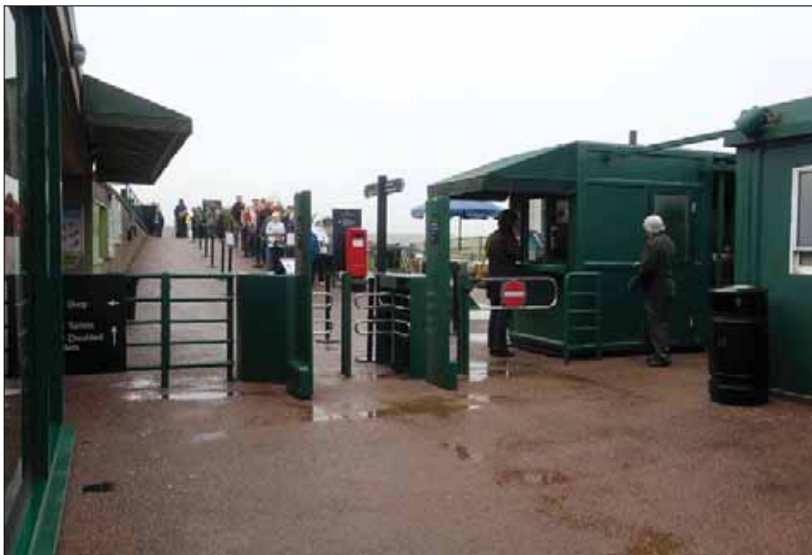
Plate 36: Entrance ramp viewed from the east. Ticket booth and turnstiles in the foreground
