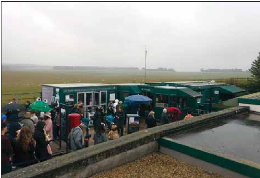
Plate 34: Visitor facilities ticket booths viewed from the south-west at car park level. The roof of the kitchen and servery are shown in the foreground
