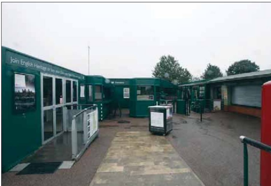
Plate 44: Ticket booths and turnstiles viewed from the west. A postbox at the base of the entrance ramps is to the right of the photograph
