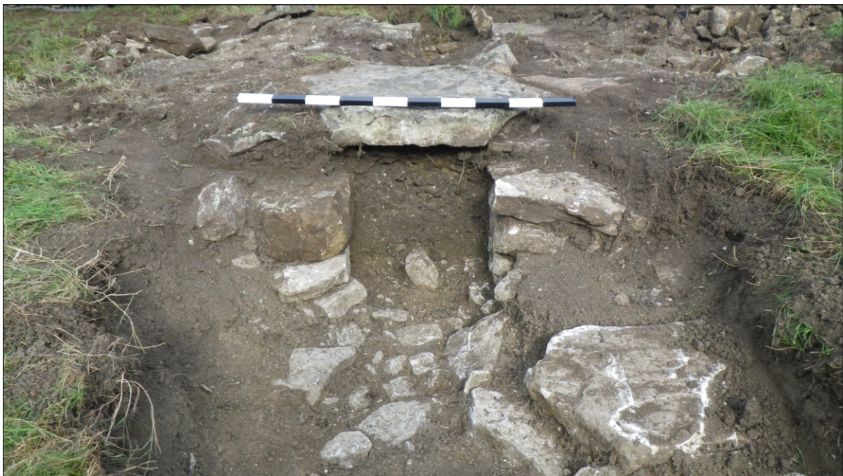
Plate 4: Detail showing culvert profile at south end. Scale 1m
