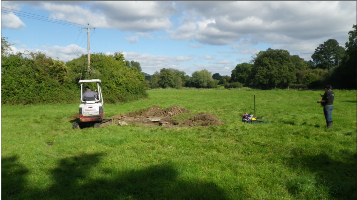
Plate 1: Showing location of culvert in relation to shallow drainage ditch
