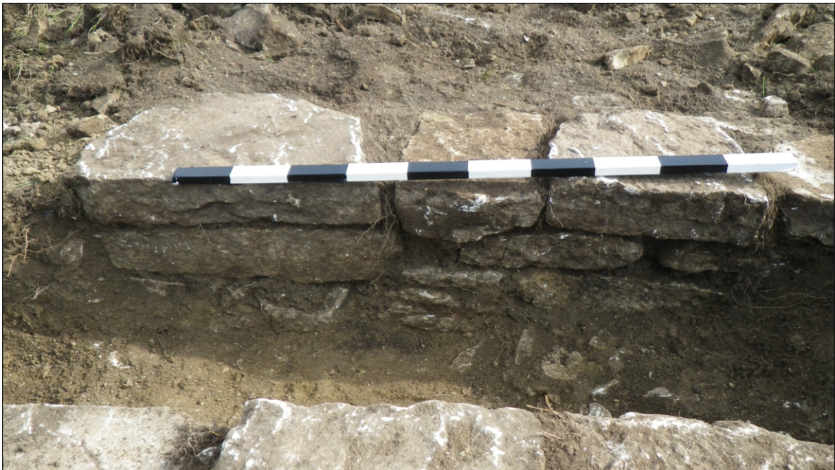
Plate 2: Detail of culvert wall construction. Scale 1m
