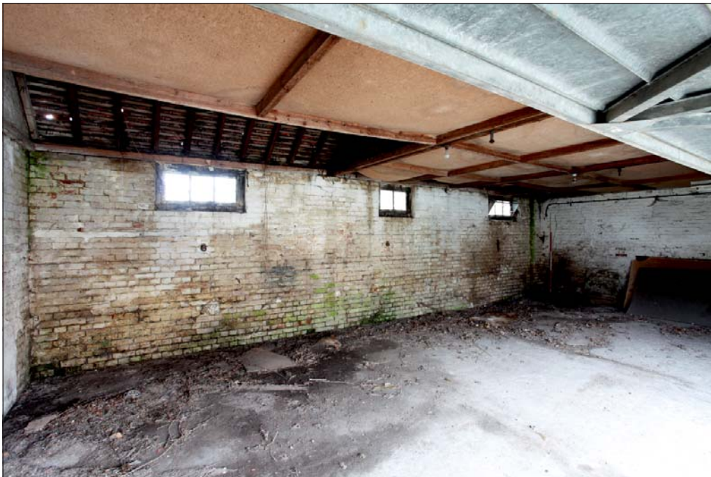
Plate 18: Manor Barn centre section interior
