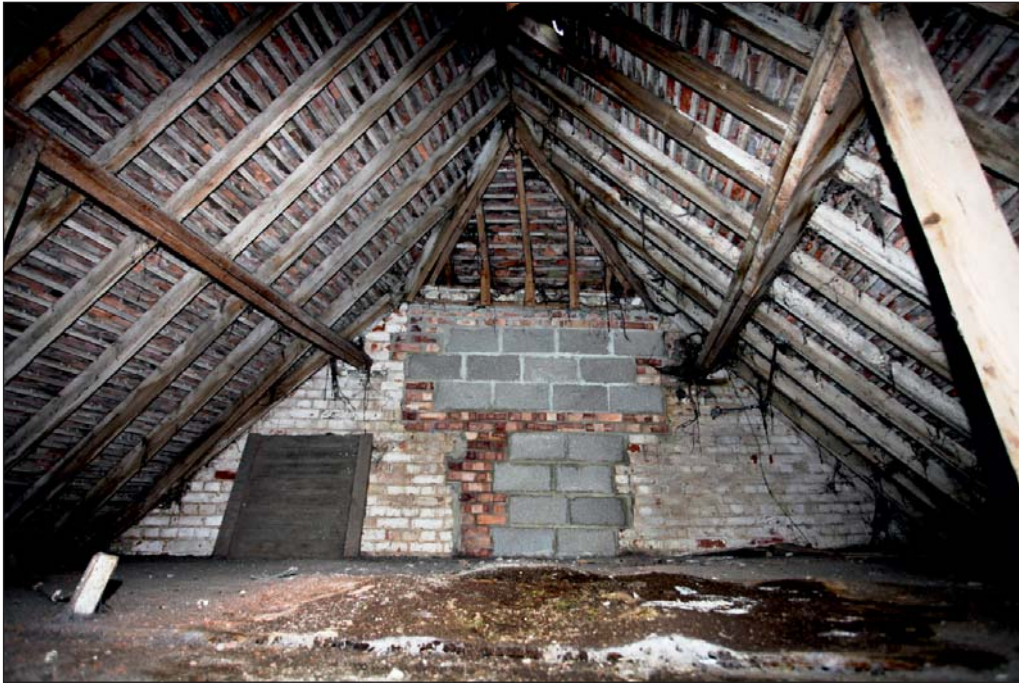
Plate 25: Old Bank roof view looking west showing blocking
