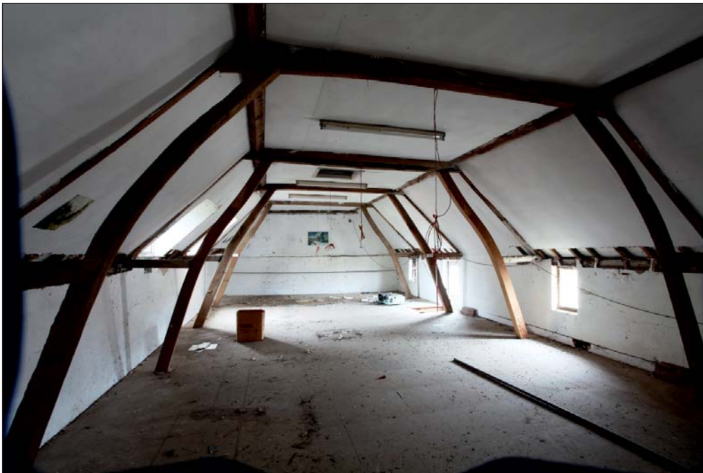
Plate 15: Manor Barn first floor south end
