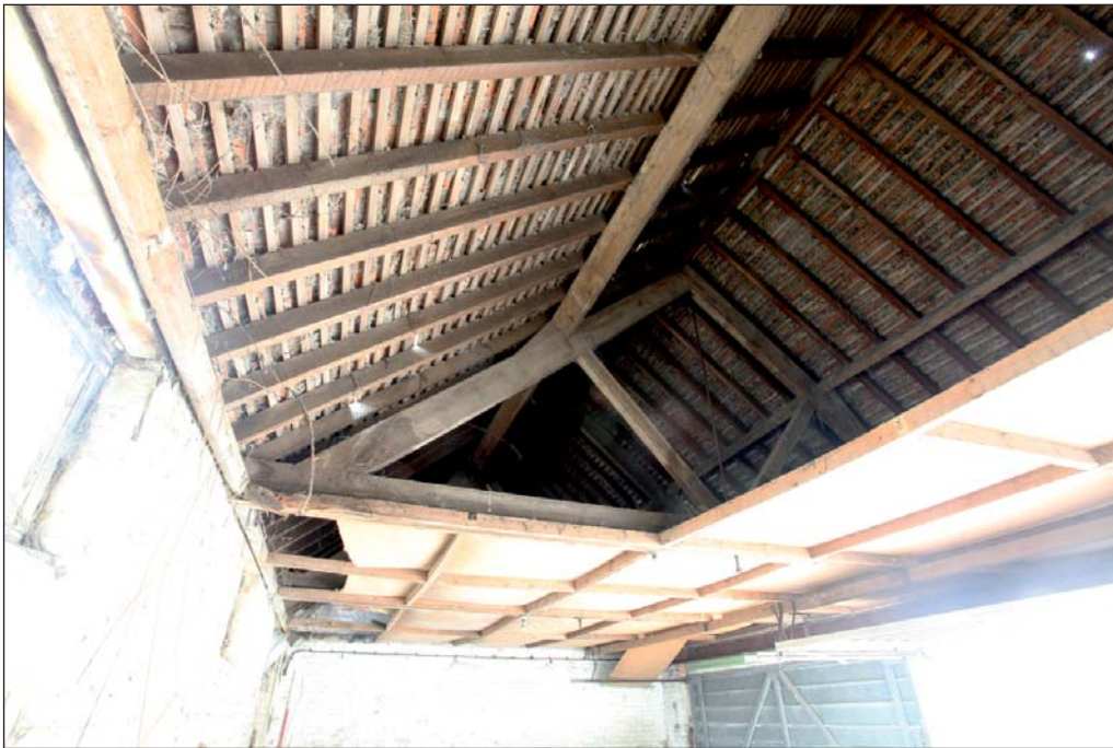
Plate 19: Manor Barn centre section roof timbers
