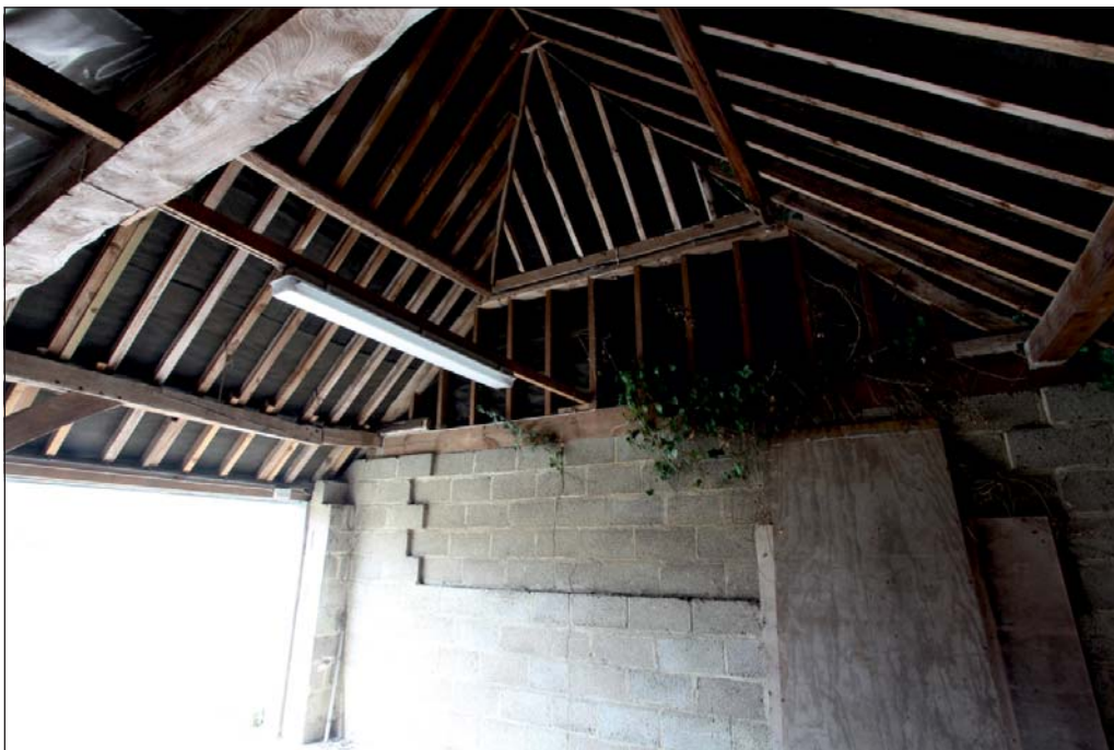
Plate 3: Interior concrete block wall north end of Coach House
