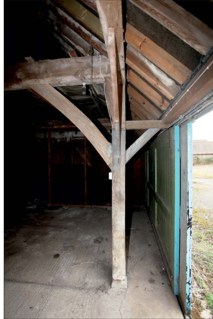
Plate 7: West arcade post and aisle tie of Coach House
