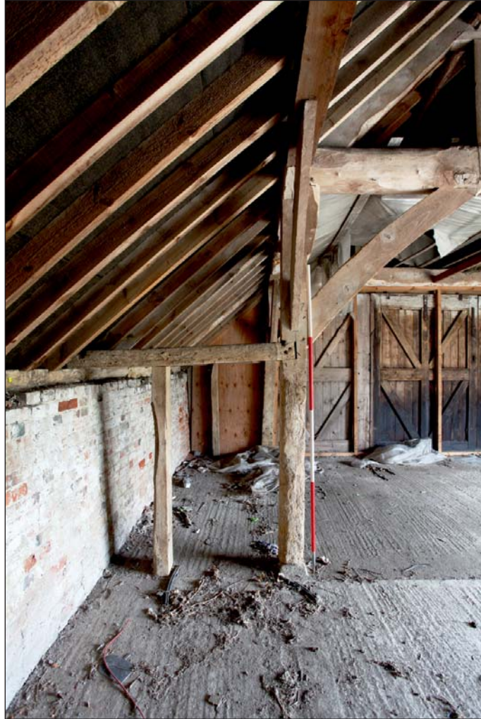
Plate 6: East arcade post and aisle tie of Coach House
