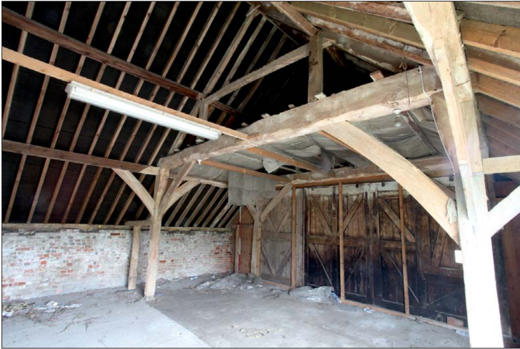
Plate 4: Interior framing of Coach House
