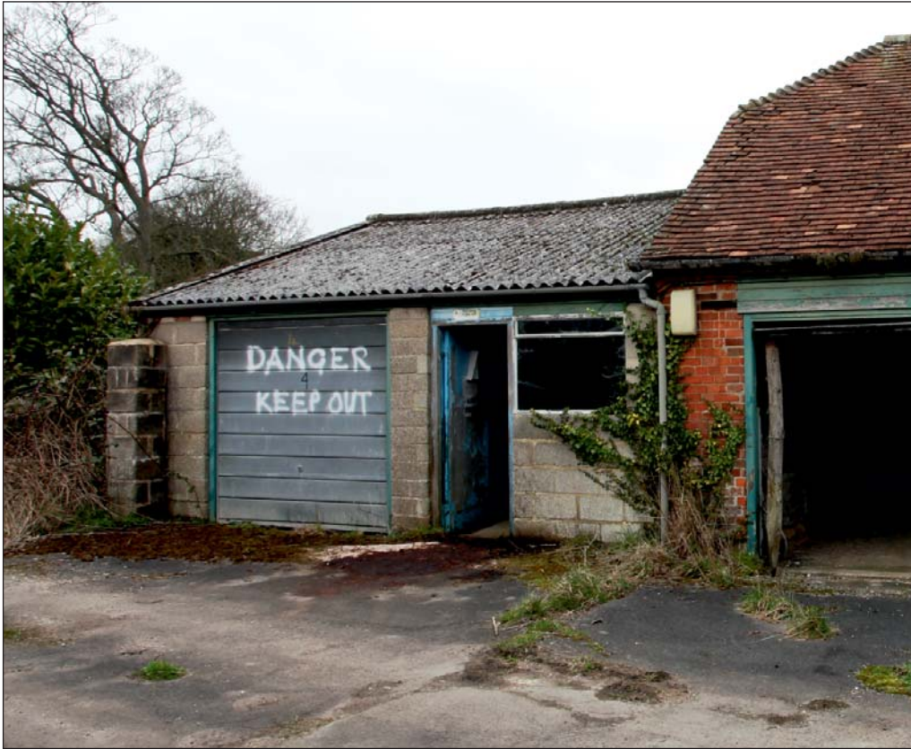
Plate 12: Manor Barn north end modern garage
