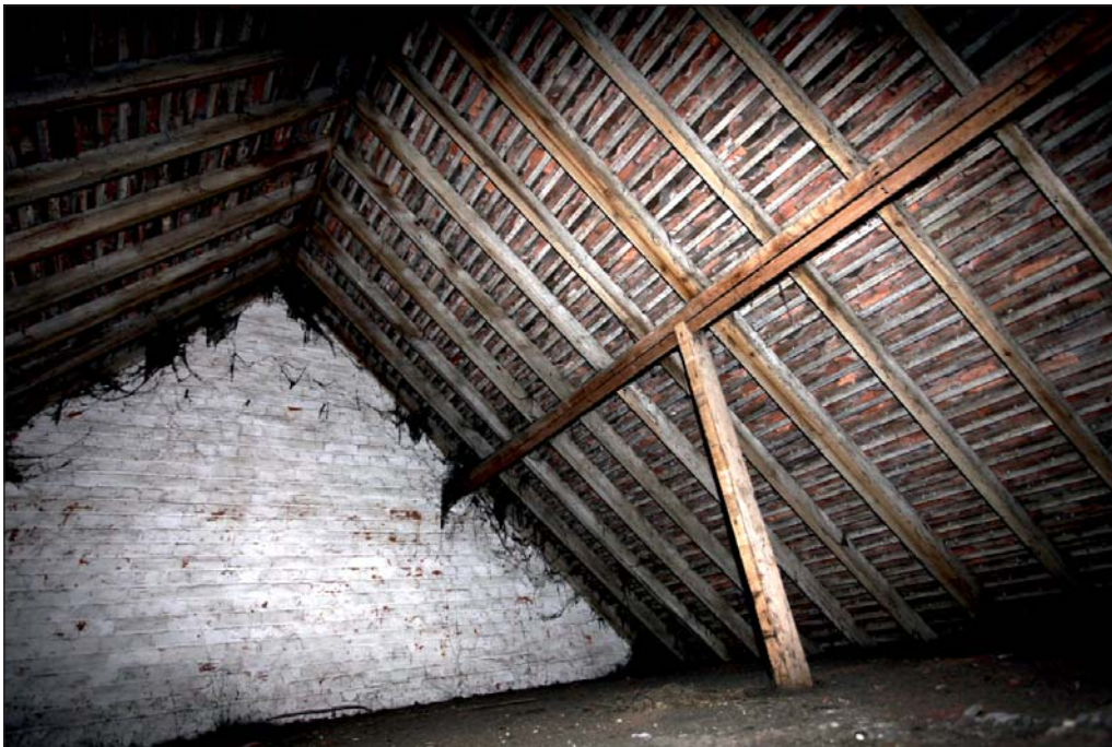
Plate 24: Old Bank roof structure
