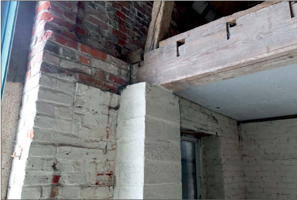
Plate 14: Manor Barn detail showing floor level change
