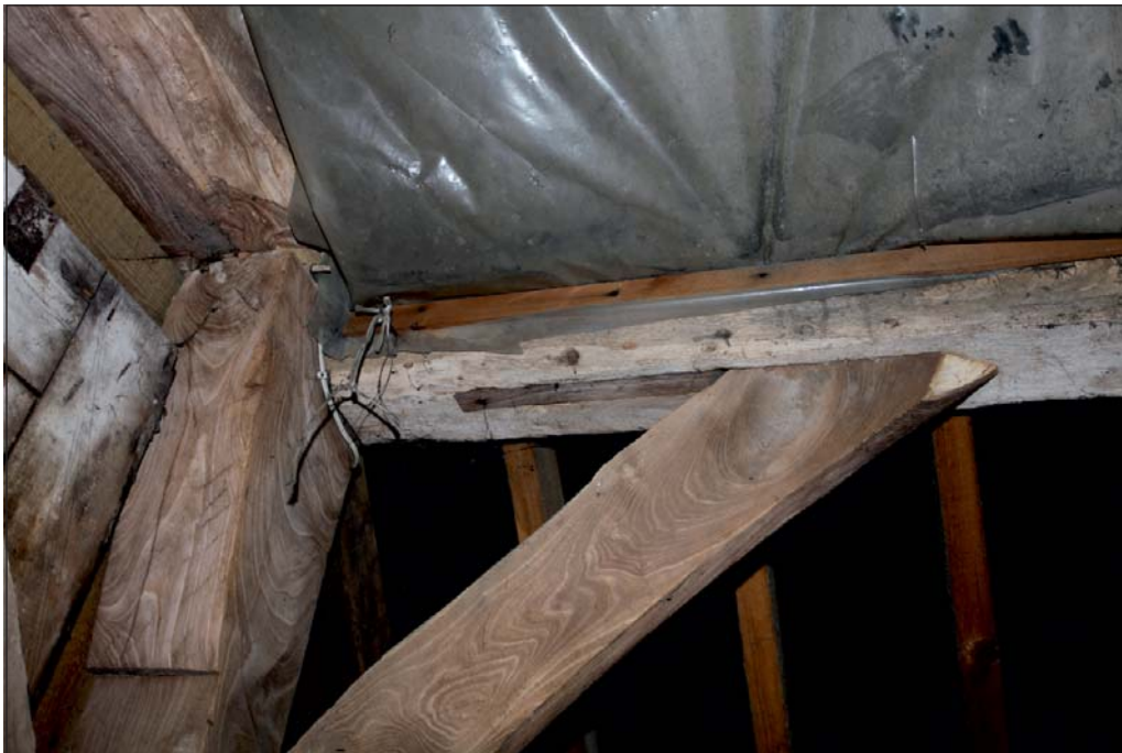
Plate 5: East arcade post and aisle tie of Coach House
