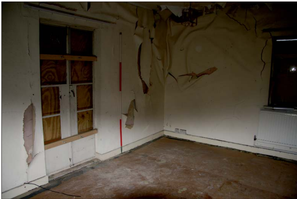
Plate 42: General view of room 2.1, noting doors to rooftop terrace
