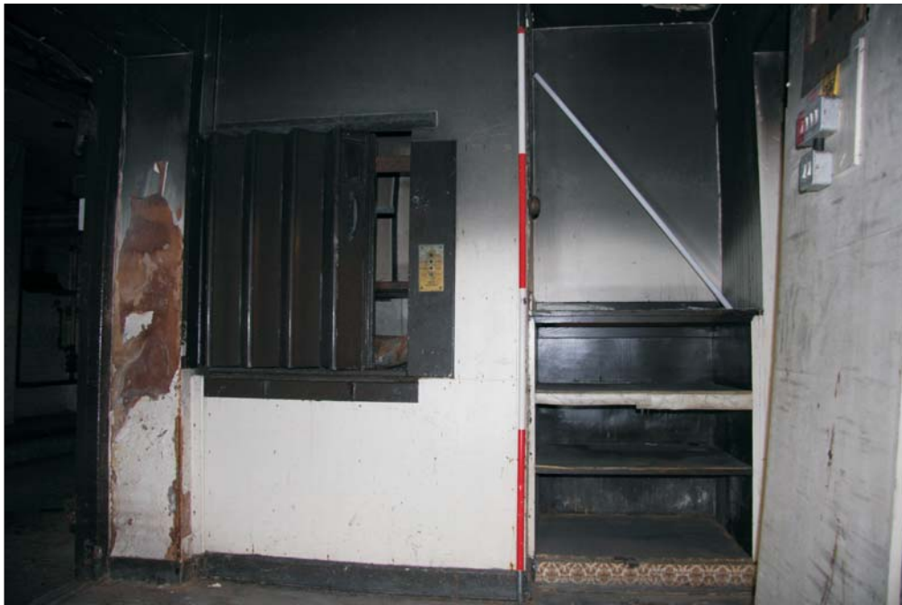
Plate 19: General view of room 0.13 showing dumb waiter
