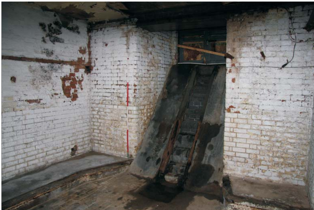
Plate 16: General view of barrel drop in lower ground floor room 0.3
