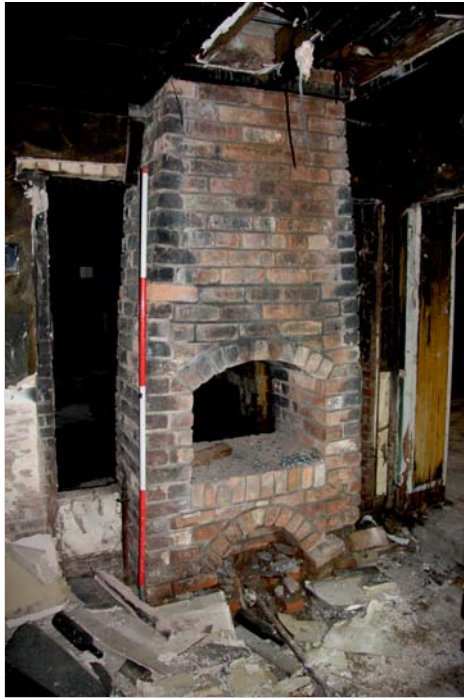
Plate 29: Detail of false rustic fireplace in room 1.3, looking north-west
