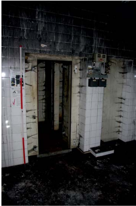
Plate 27: Detail of inserted rooms 1.8 and 1.10, looking south
