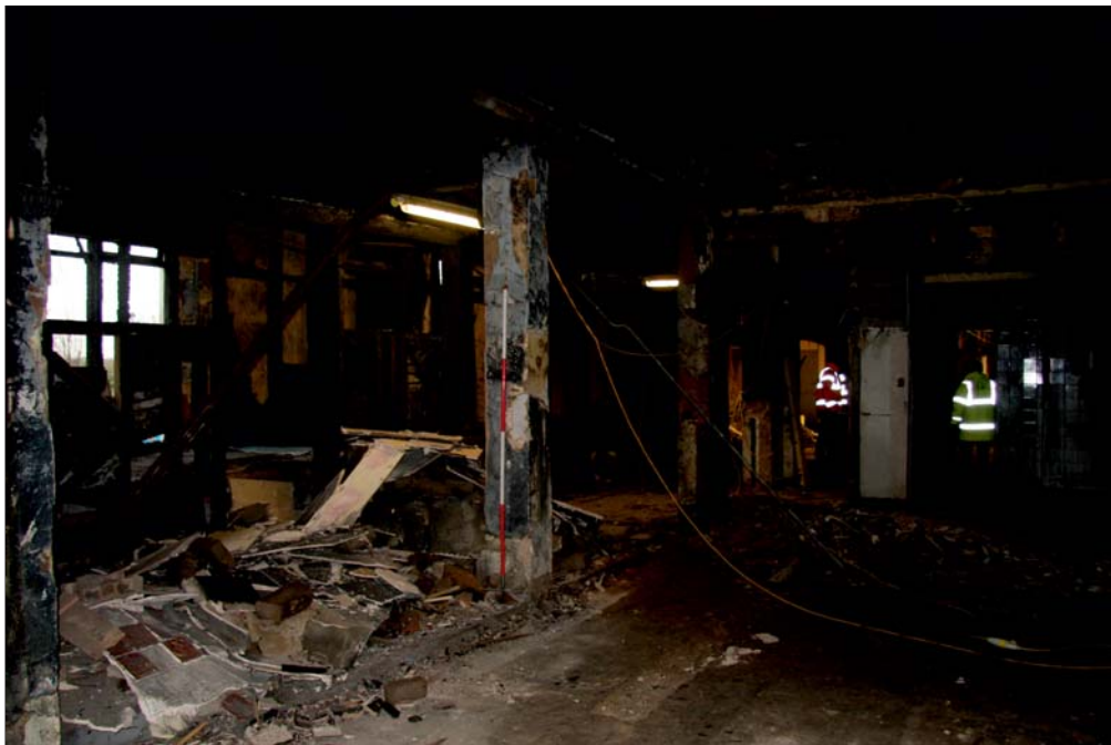
Plate 28: General view of 1.11 looking into rooms 1.6 and 1.7 and showing rusticated partitions
