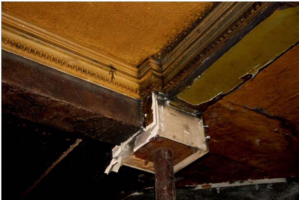
Plate 30: Detail of dentil patterned cornice between rooms 1.4 and 1.5
