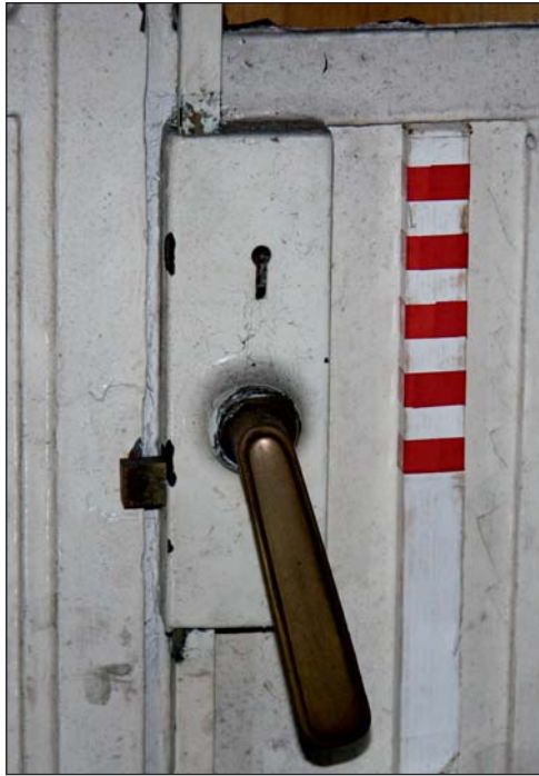
Plate 43: Detail of latch to terrace door in room 2.1
