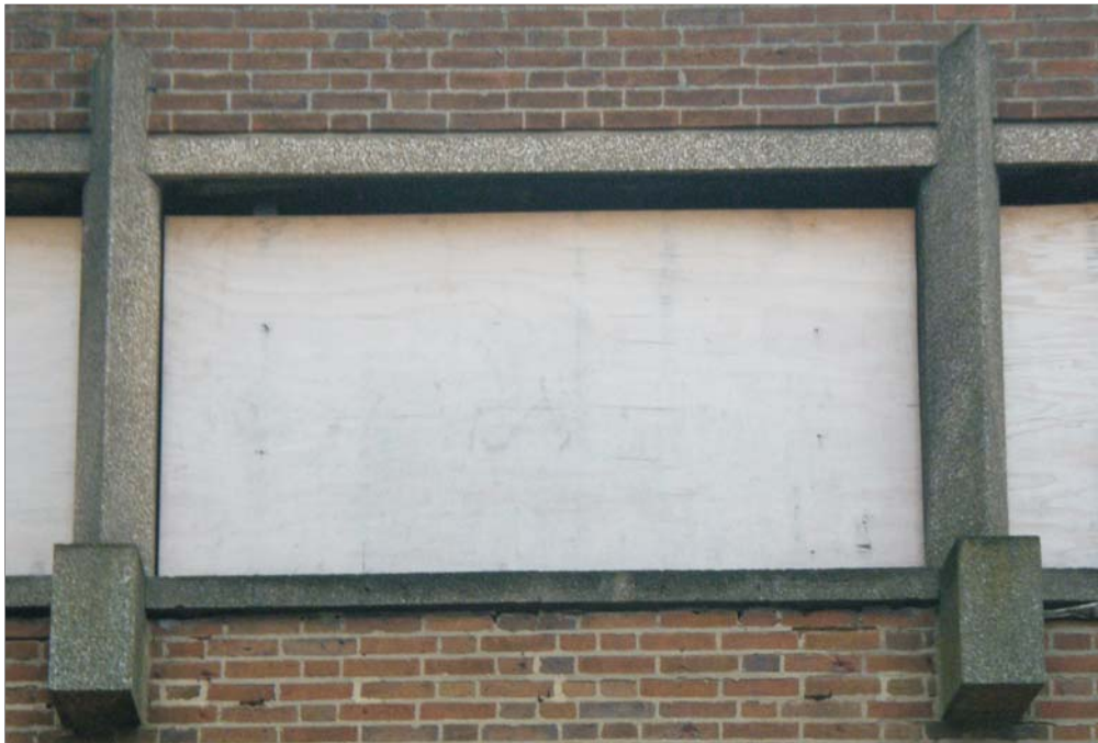
Plate 4: Detail of the first floor windows in the west elevation
