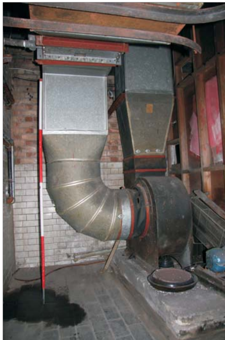
Plate 22: Detail of ventilator in room 0.15
