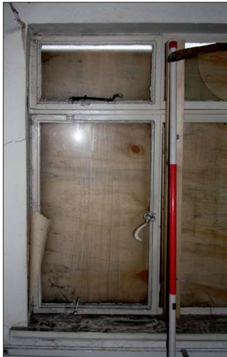
Plate 44: Detail of window in room 2.1
