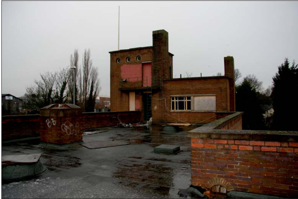
Plate 45: General view of stair tower and second floor room from roof of main block, looking north
