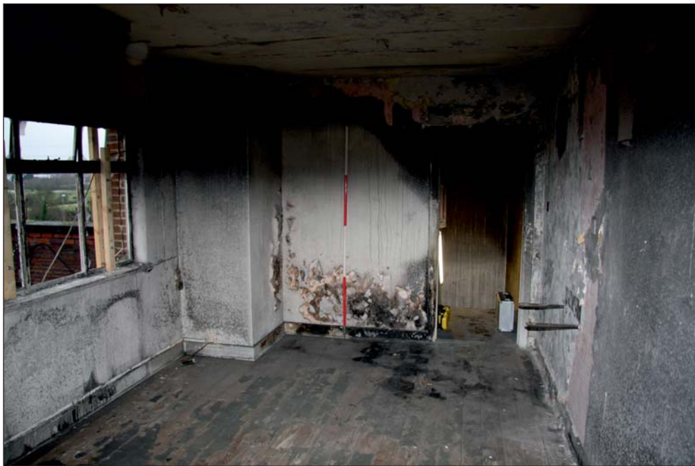
Plate 46: General view of room 2.1, looking west
