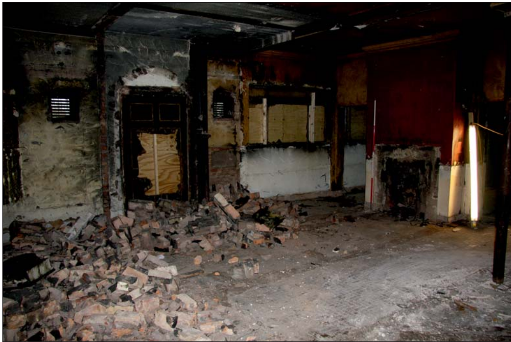
Plate 31: General view of former bar room 1.4, looking west
