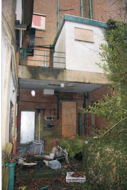
Plate 15: General view of north elevation, showing balcony and service entrances
