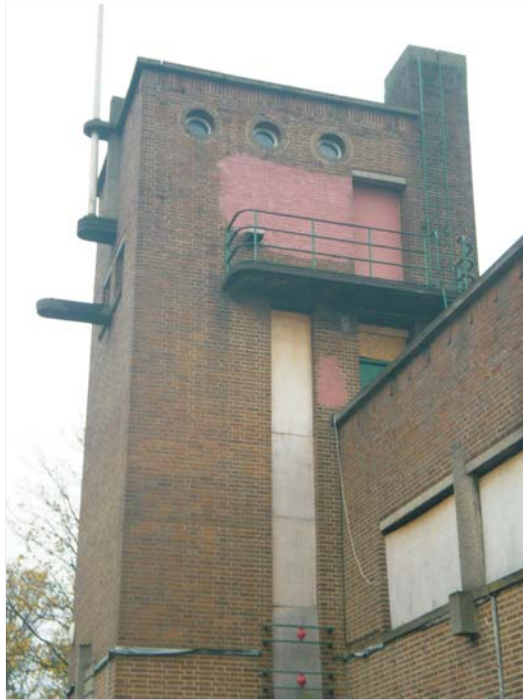
Plate 7: General view of stair tower structure, looking north-east
