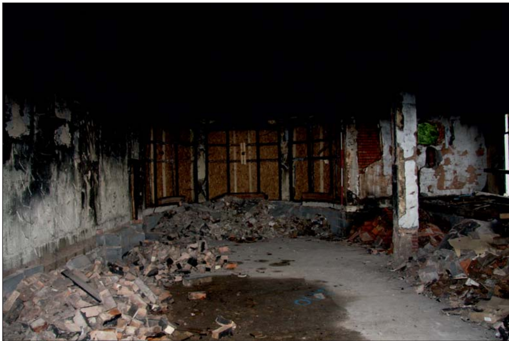
Plate 32: General view of room 1.11, looking north
