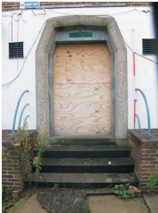
Plate 2: Detail of the southern door in the west elevation
