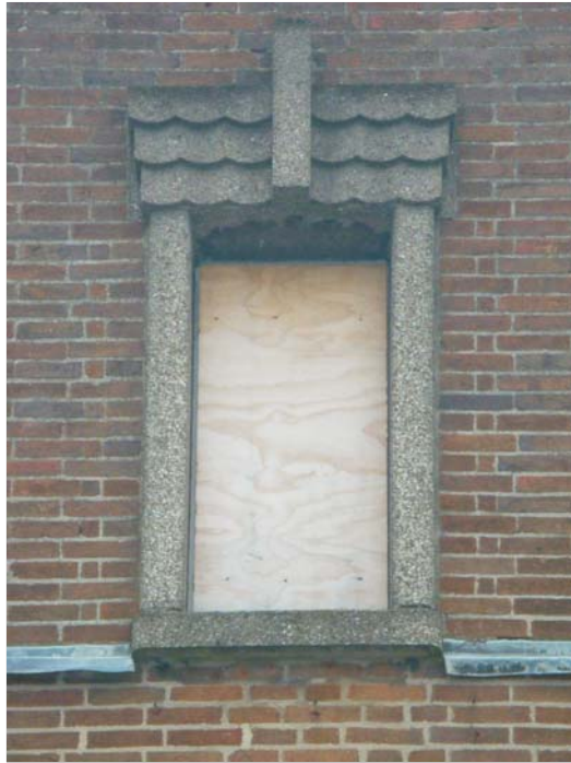
Plate 5: Detail of first floor window with art-deco architrave, west elevation
