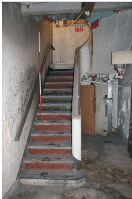
Plate 20: General view of room 0.14 showing staircase
