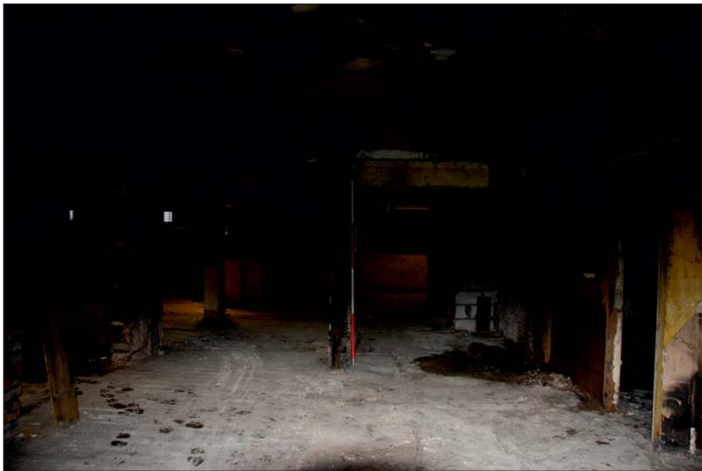
Plate 26: General view of rooms 1.18 and 1.5 showing extent of removed internal walls
