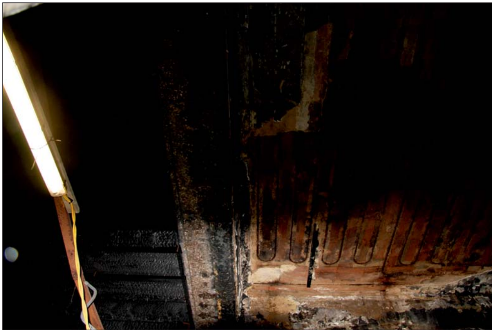
Plate 34: Detail of change in roof structure between 1.6 (left) and 1.11 (right)
