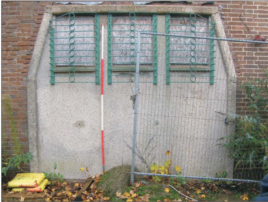
Plate 9: Detail of blocked vehicular door with inserted windows, west elevation
