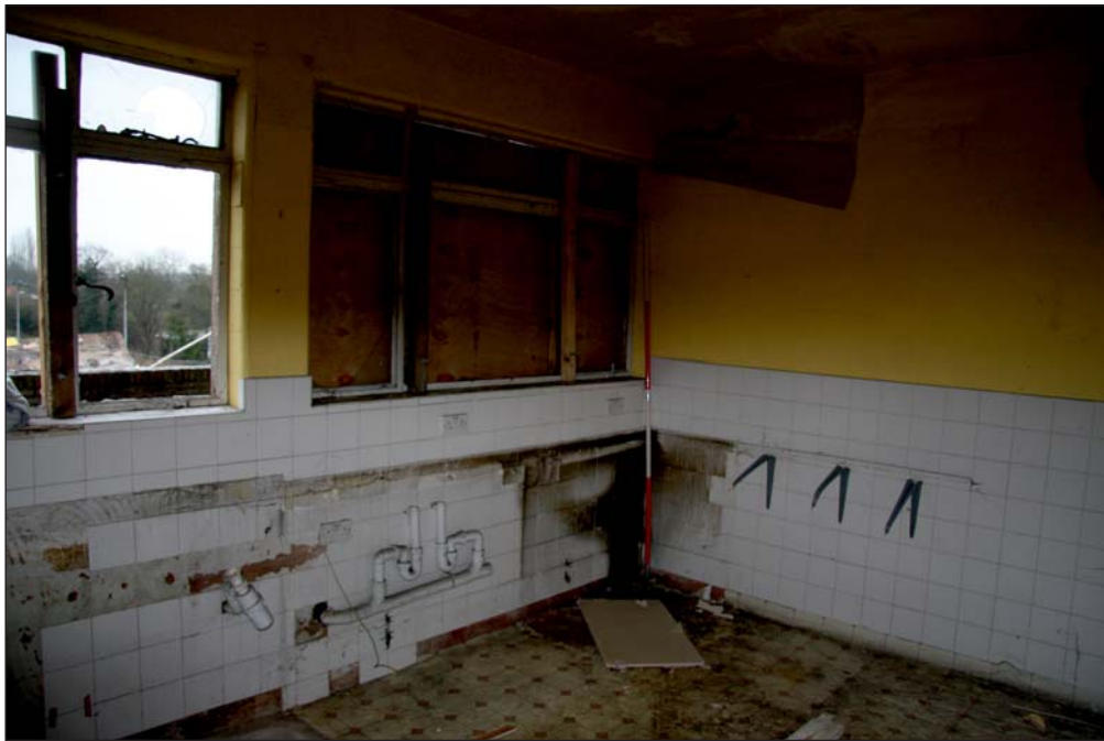
Plate 41: General view of room 2.8
