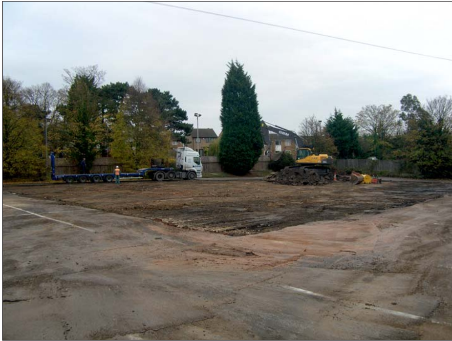
Plate 47: General view of watching brief area, looking north-east
