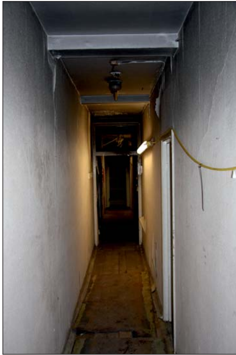
Plate 37: General view of corridor 2.9, looking south
