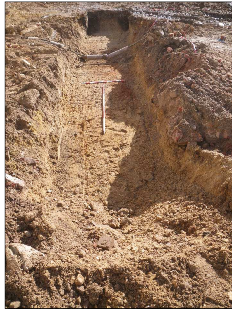
Plate 2: Trench 4 from the south-east
