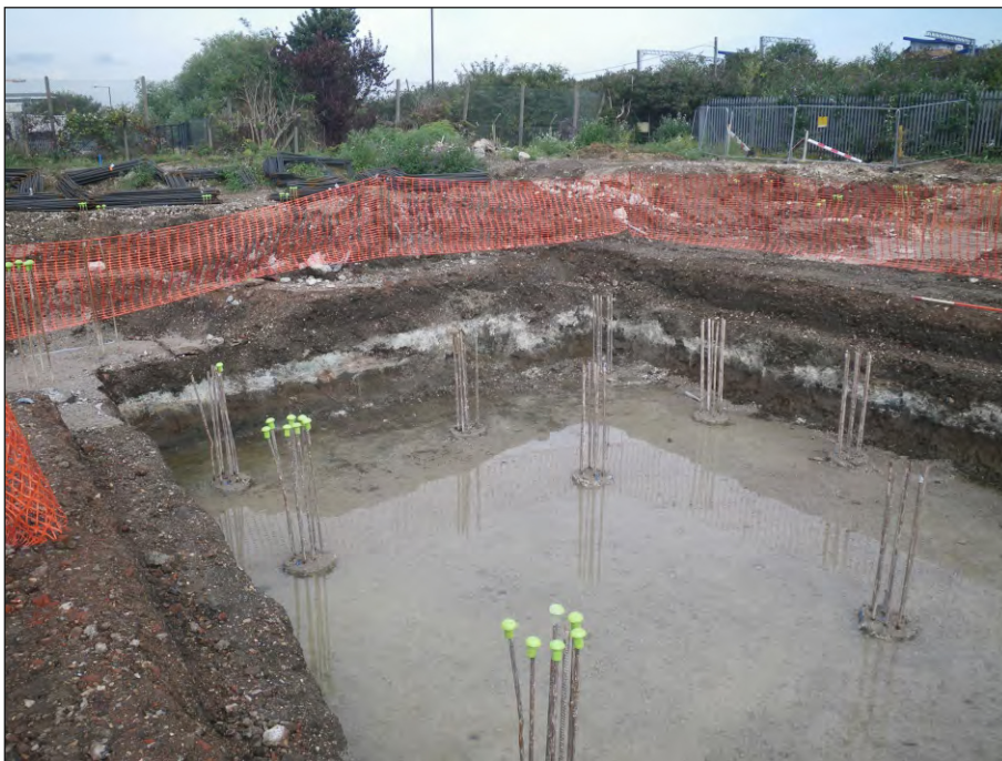
Plate 2: Trench 1 viewed from the south
