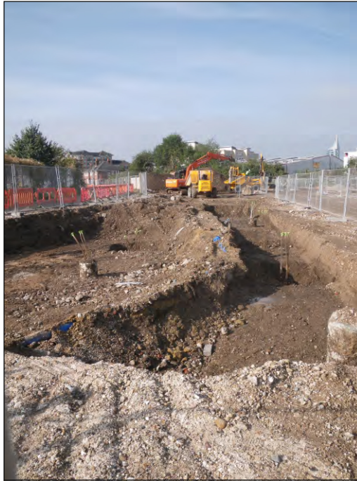
Plate 7: View of the Site
