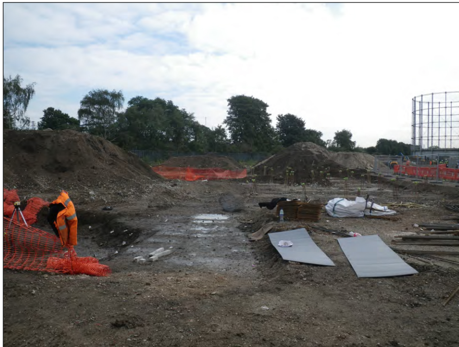
Plate 8: View of the Site
