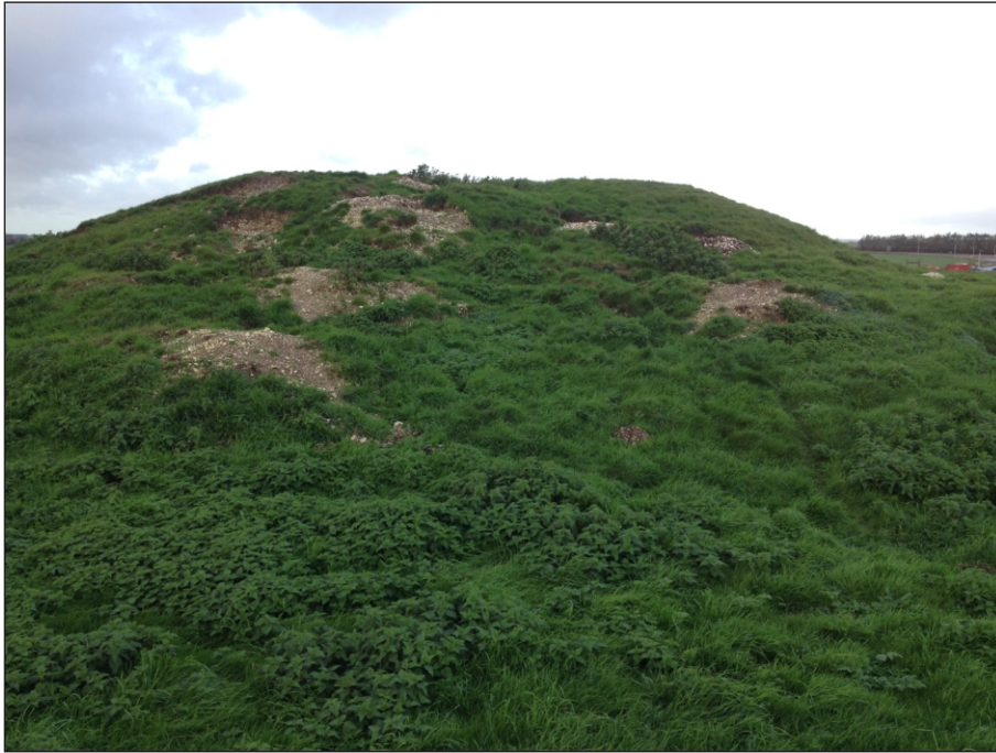
Plate 3: Example of badger sett damage (Barrow B)
