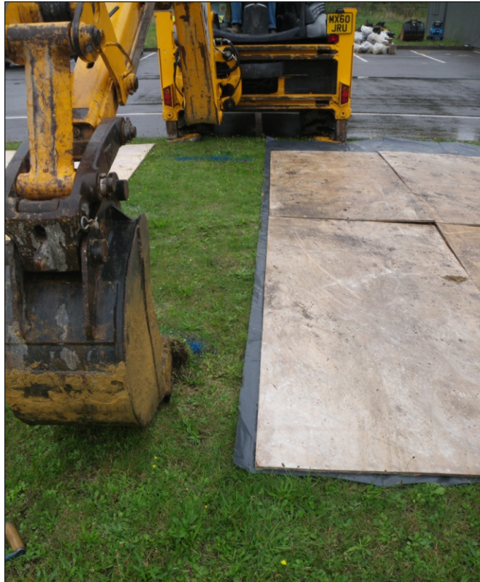
Plate 1: Working shot: Test Pit 1109
