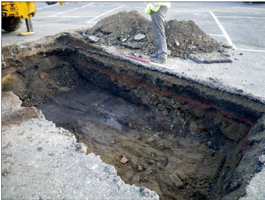
Plate 2: Trench 2, looking south-east
