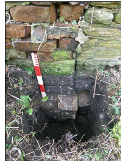
Photograph of Inspection Pit 5, looking east
