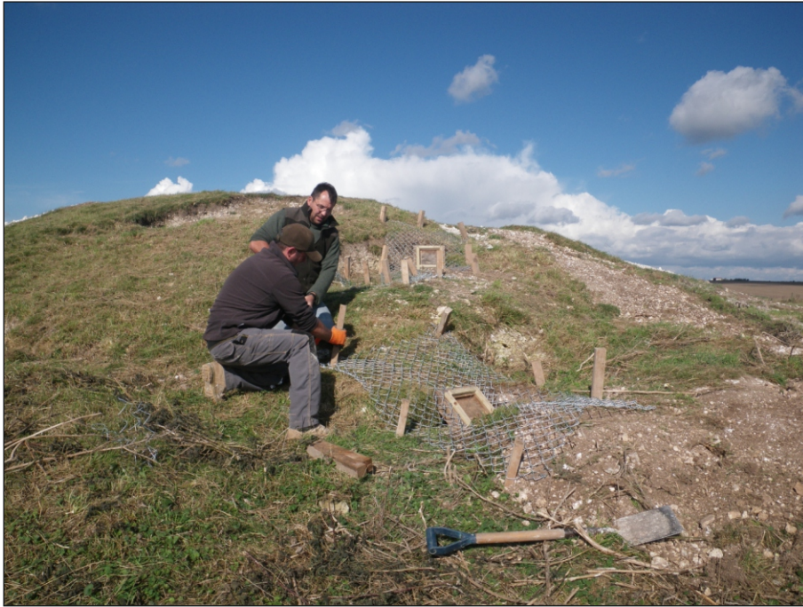
Plate 1: Wildlife Co. installing badger sett closure measures (Barrow A)
