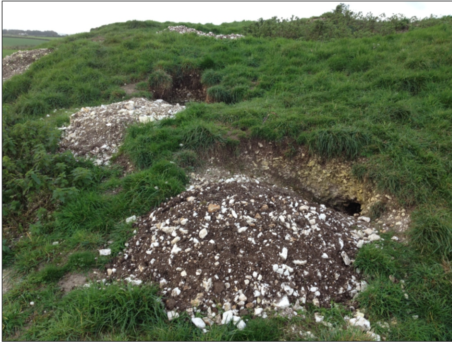
Plate 5: Example of badger sett damage (Barrow B)
