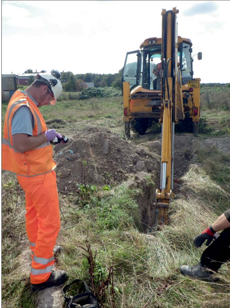
Plate 7: Larkhill: machine excavation (Test pit 1340)
