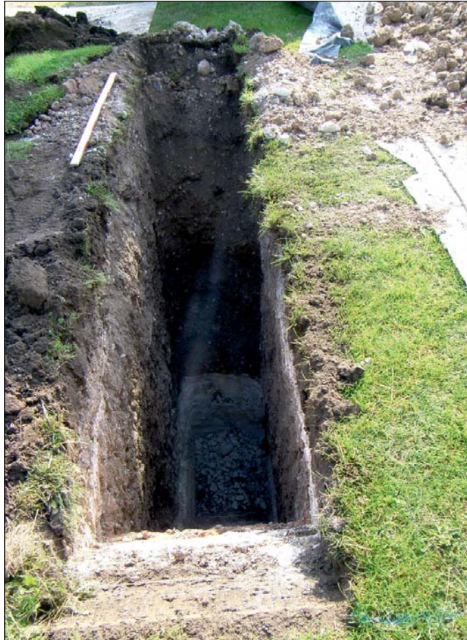
Plate 16: Tidworth: Test pit 1566 from the west, showing deep made-ground
