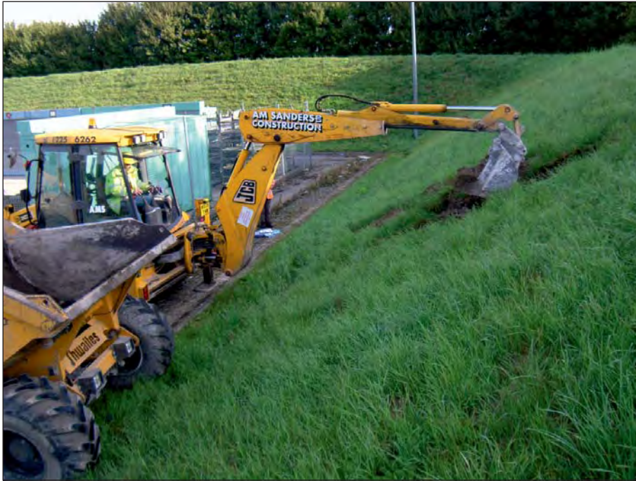
Plate 12: Perham Down: machine excavating into a bank (Test pit 1433)
