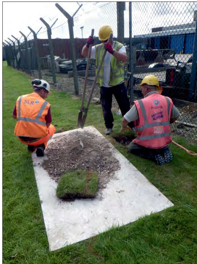
Plate 6: Larkhill: hand-excavation (Test pit 1347)
