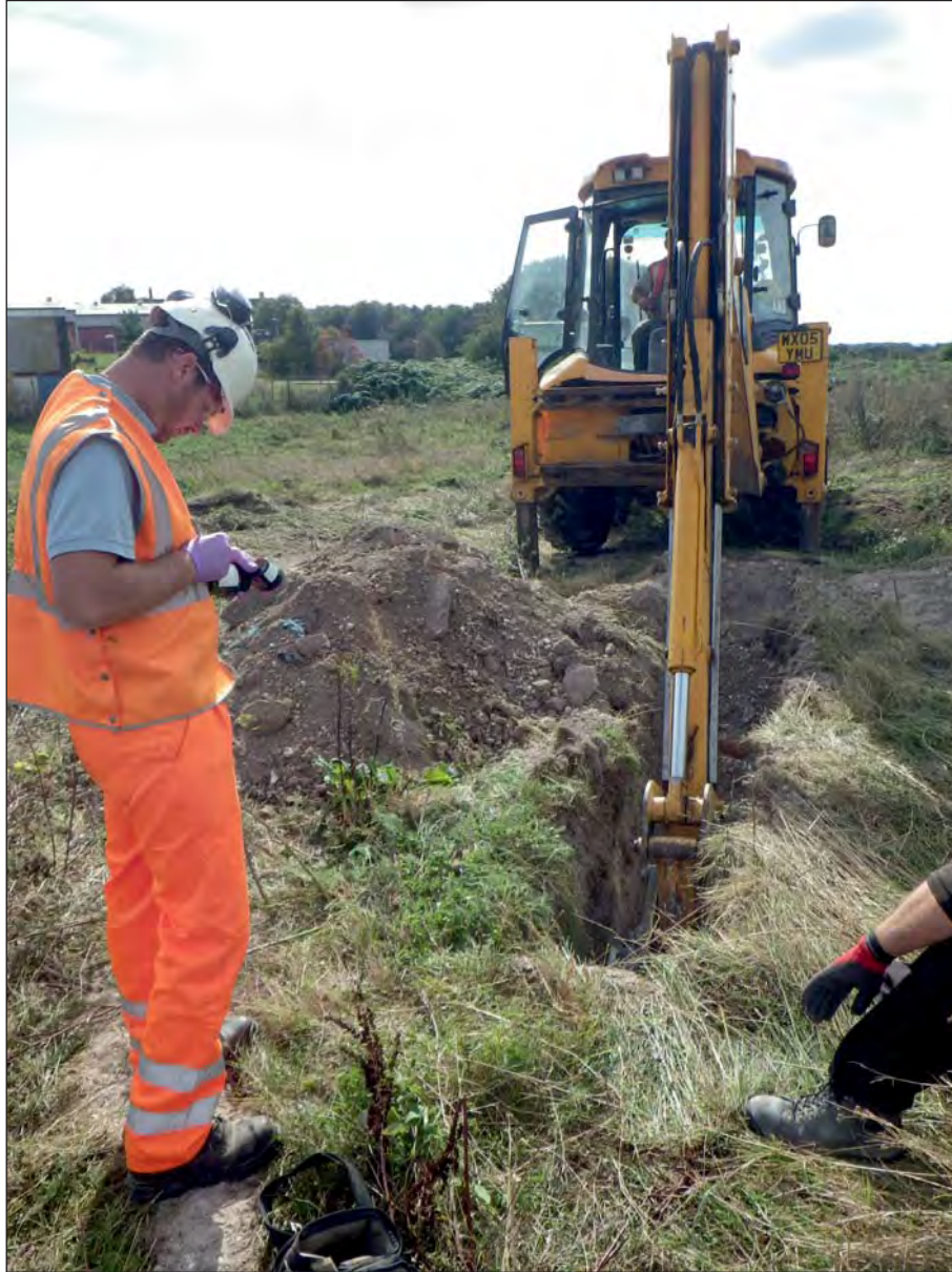
Plate 7: Larkhill: machine excavation (Test pit 1340)
