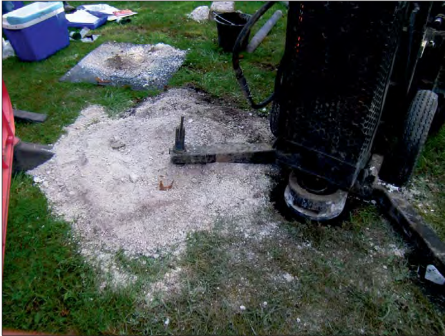
Plate 10: Perham Down: borehole sampling
