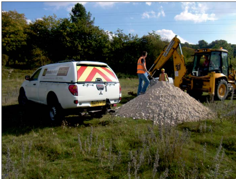
Plate 2: Bulford: working shot near Test pit 1266
