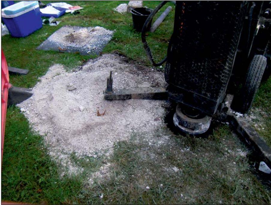
Plate 10: Perham Down: borehole sampling
