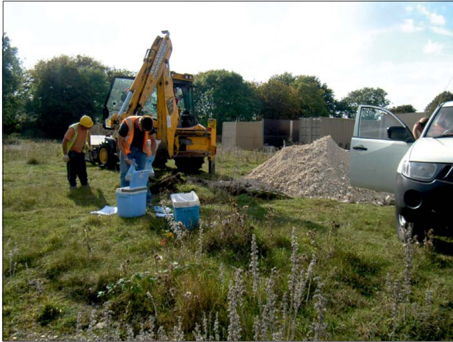
Plate 1: Bulford: working shot near Test pit 1266
