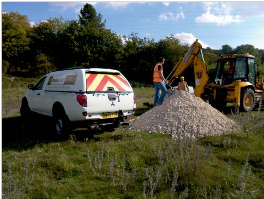
Plate 2: Bulford: working shot near Test pit 1266
