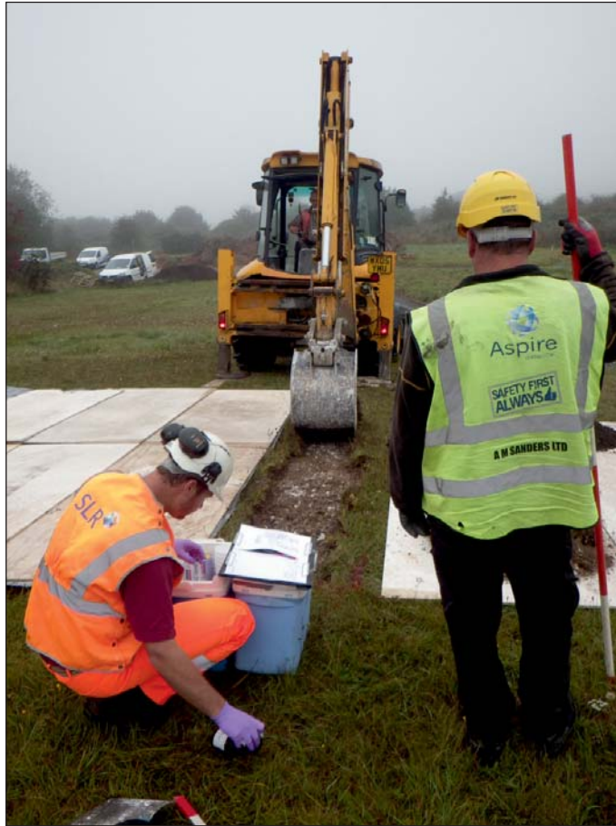
Plate 8: Larkhill: machine excavation (Test pit 1366)
