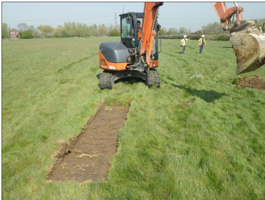
Plate 2: Working shot showing typical scheme landscape and operations
