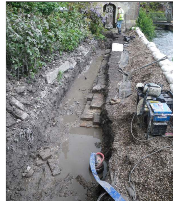
Plate 4: North facing view of wall 1616
