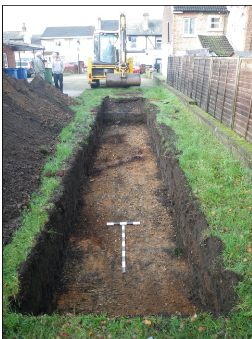
Plate 1: Trench 1, view from the east
