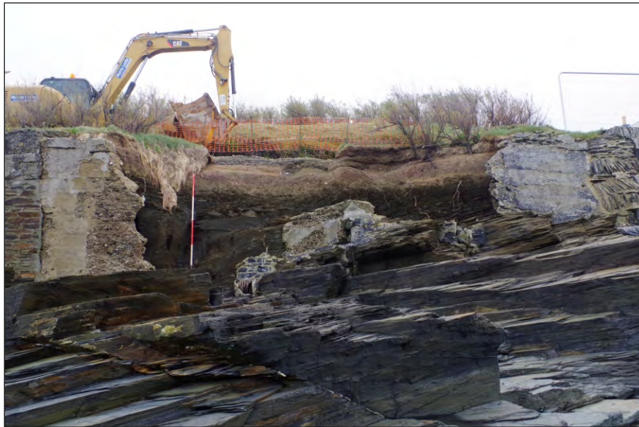
Plate 1: Trevone sea wall pre excavation from North West
