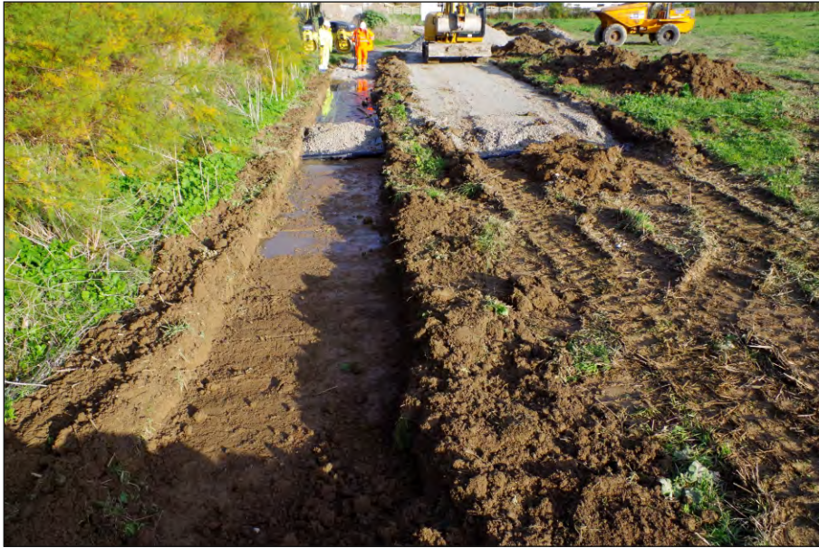
Plate 3: General view of the footpath diversion trench from South West
